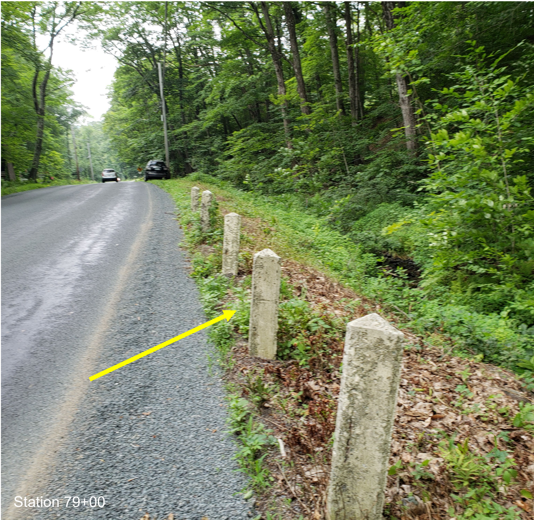
Substandard side slope protection from steep slopes/brook
