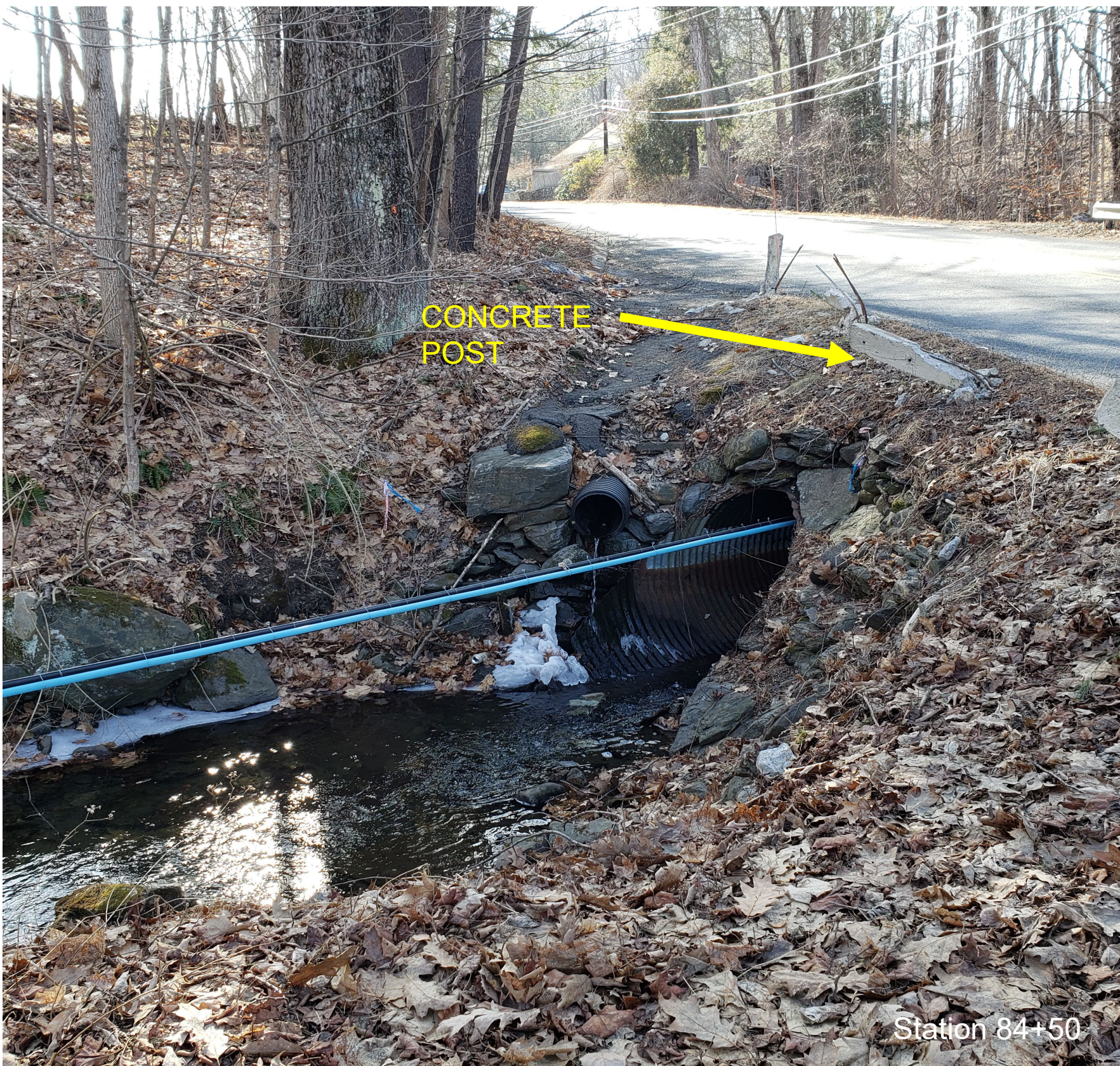
Substandard side slope protection from steep slopes/brook, roadway discharge to brook
