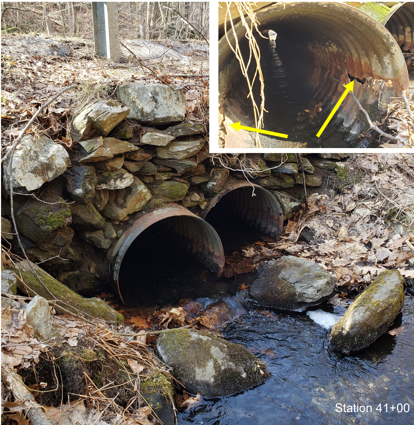
Deteriorated drainage pipes, headwalls with erosion
