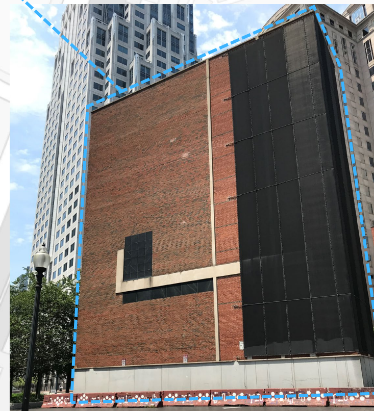
Essex St. Vent Structure
