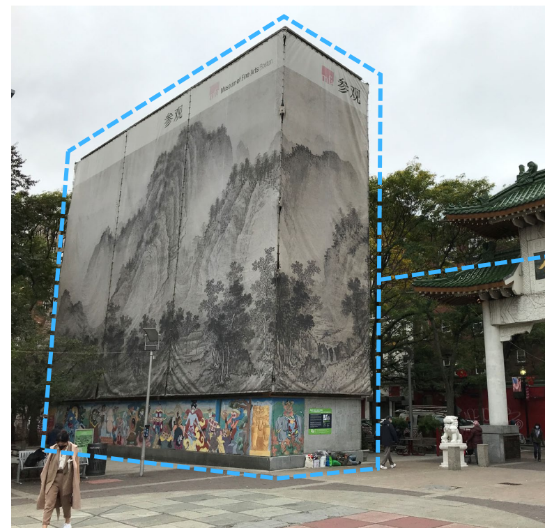
Beach St. Vent Structure
