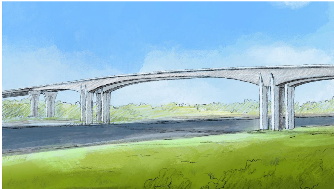
Concrete Box Girder
