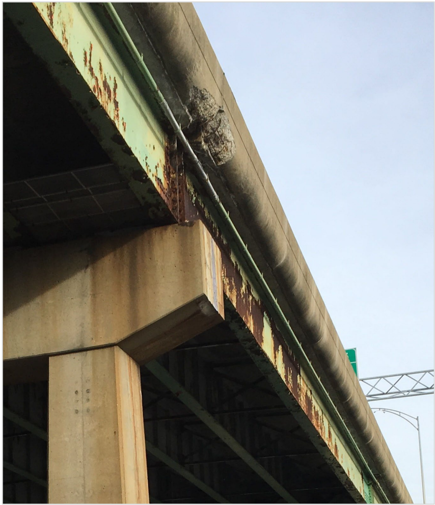
Deteriorated steel
