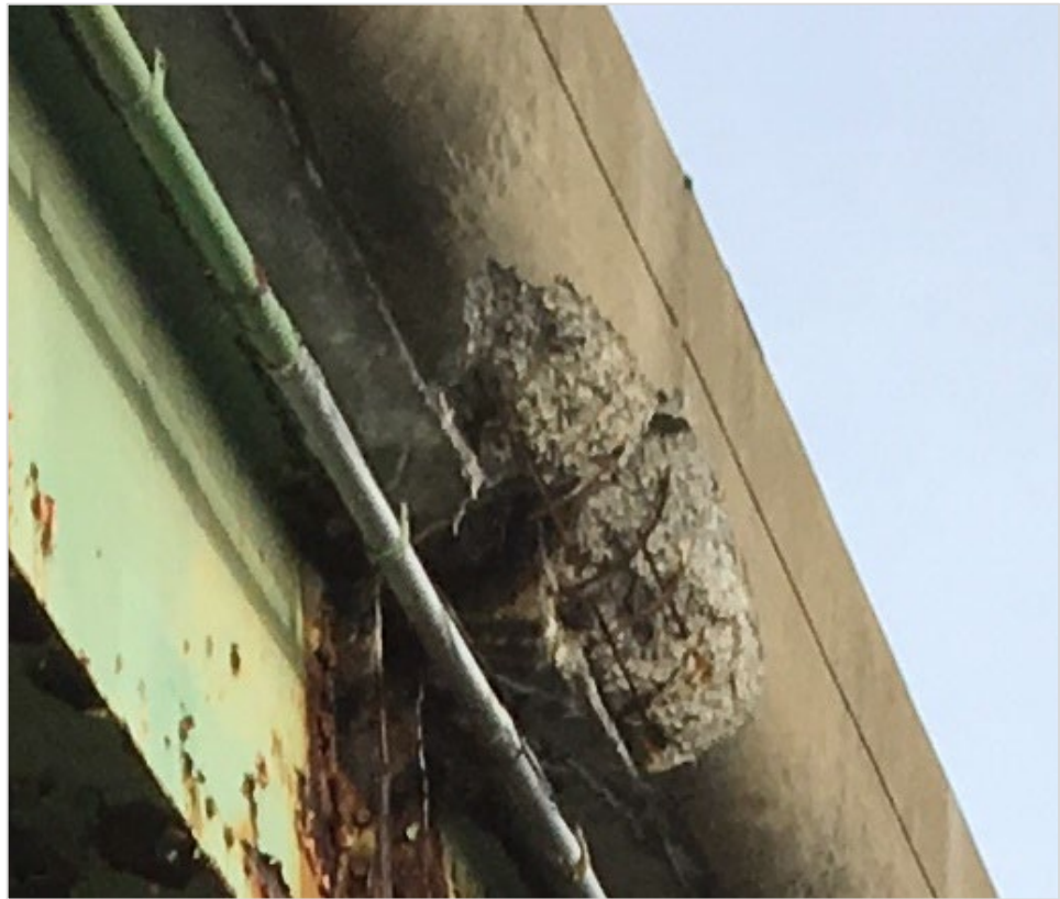
Spalling concrete
