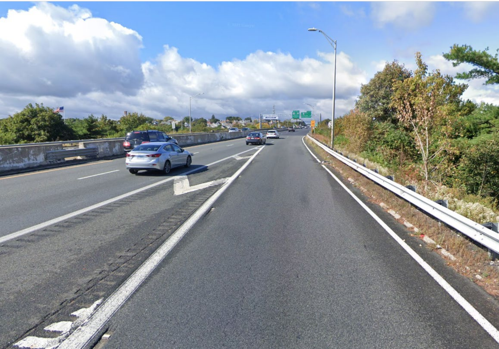
Limited weaving area when merging onto I-195 WB from Ramp D
