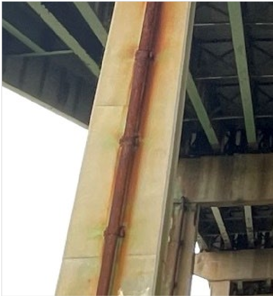
Rusted pipes
