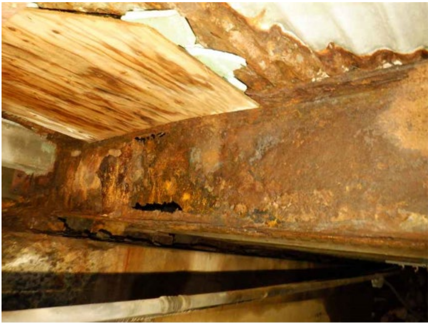
Existing Beam with Advanced Deterioration and a Corrosion Hole in the Web
