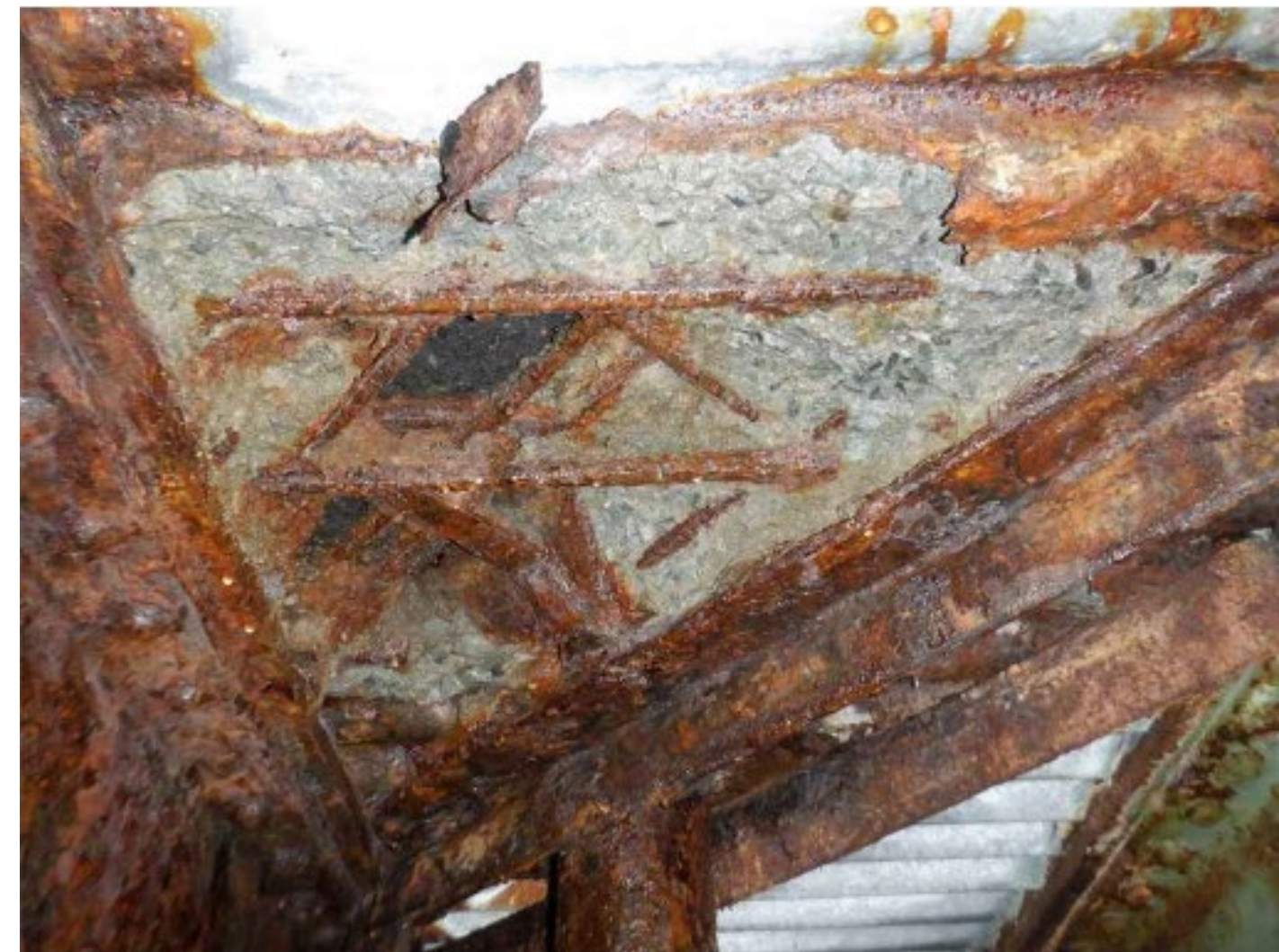
Deterioration of the Underside of Bridge Deck
