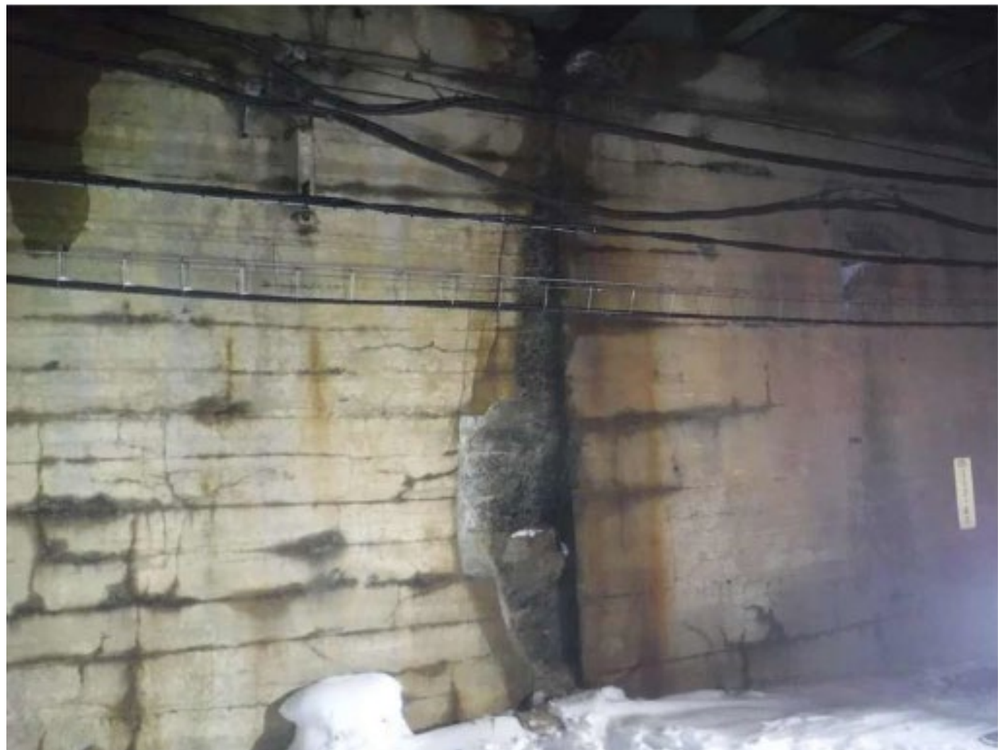
Existing Concrete Abutments with Spalls, Cracks, and other Deterioration
