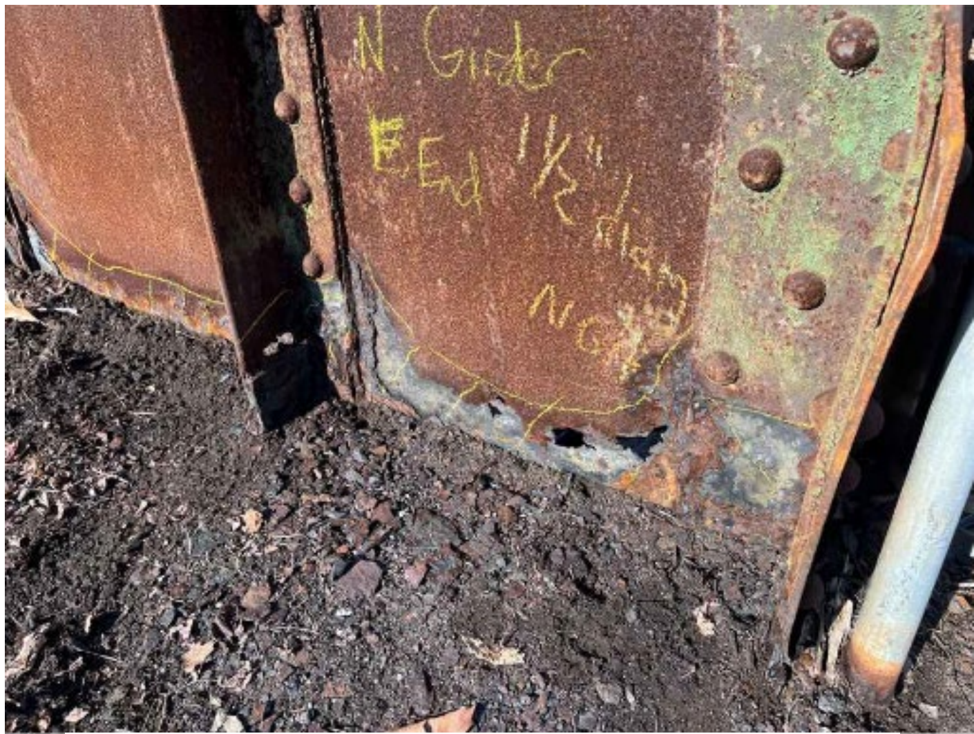
Fascia Girder with Advanced Section Loss and Holes in the Web Plate
