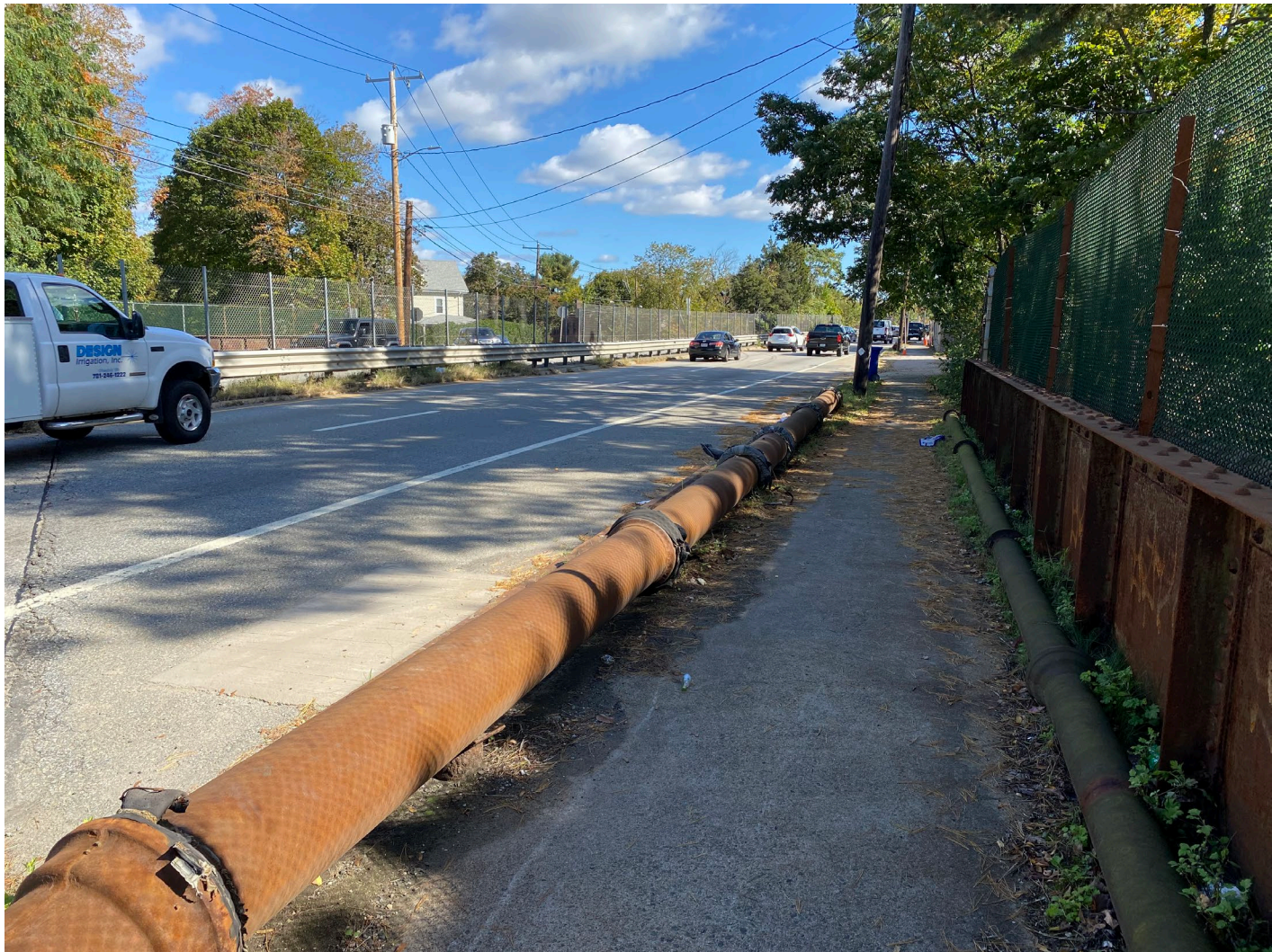
Existing Sidewalk with Exposed Utility Pipe and Girder Serving as Bridge Rail
