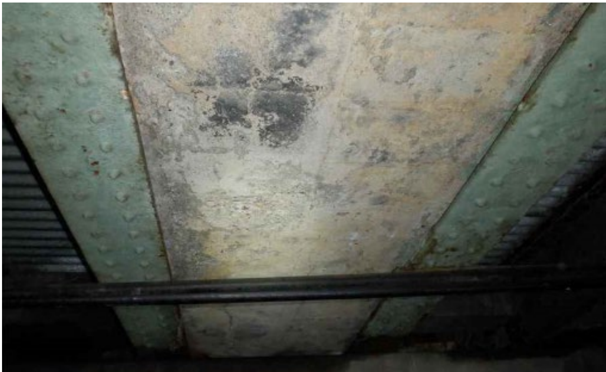
Conc. Encased Conduit Bay Below
