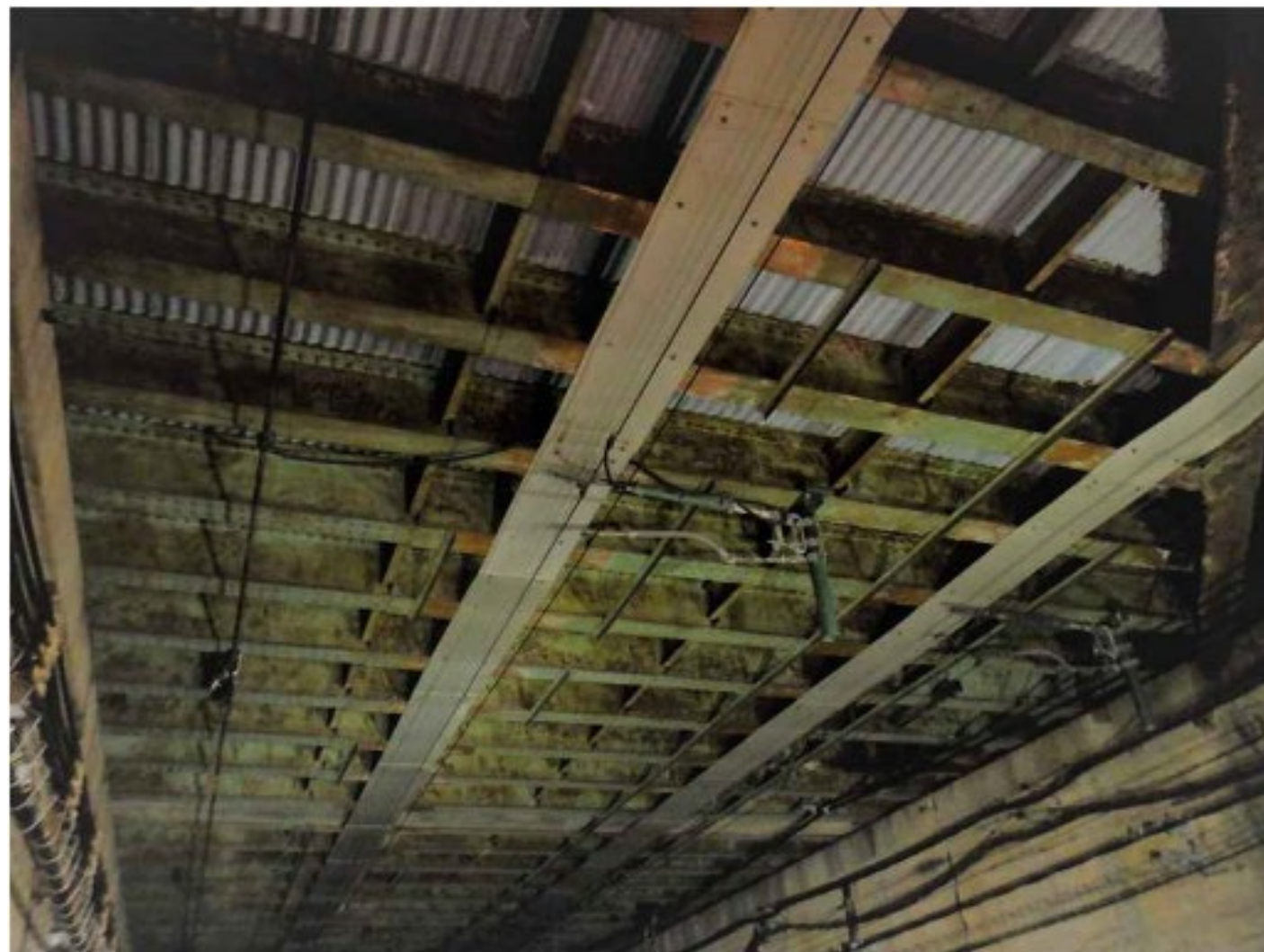
Underside of Bridge with Rust and Section Loss to Steel Framing
