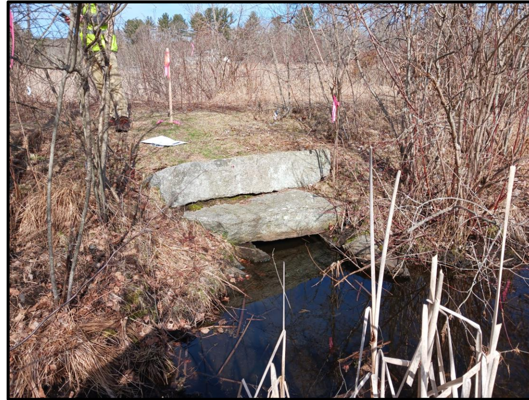
Existing granite culvert
