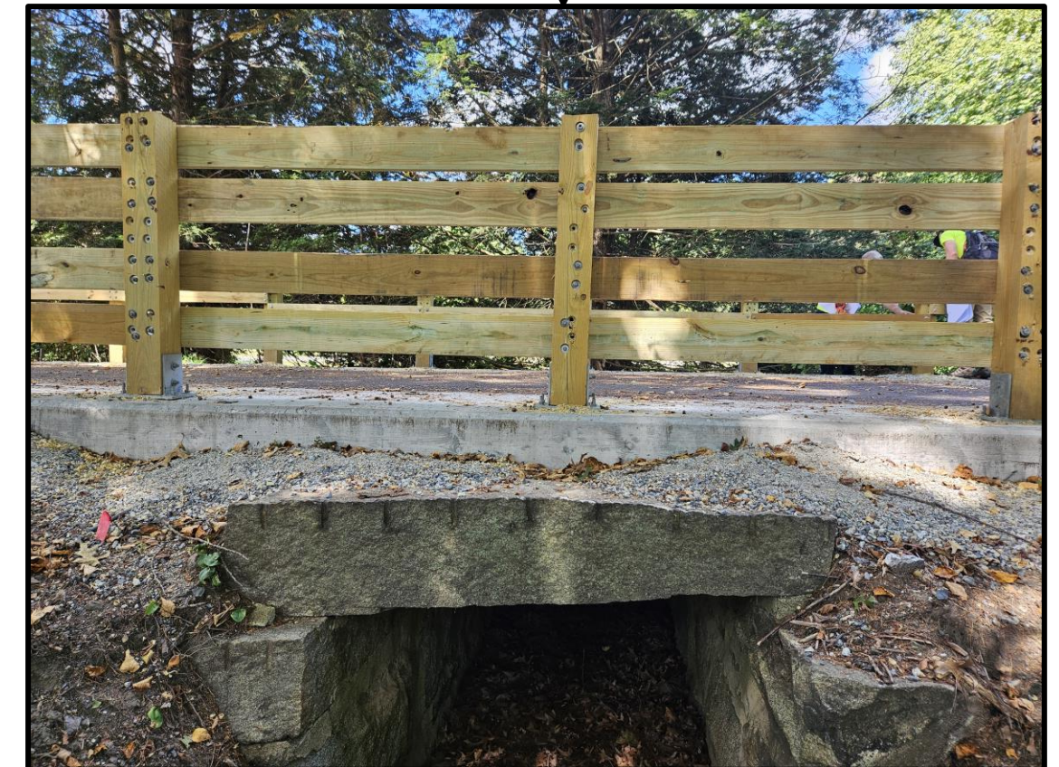
Reinforced cattle crossing on BFRT Phase 2D
