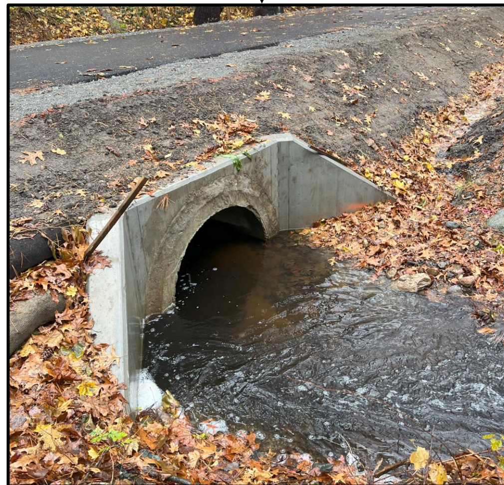
Precast concrete culvert on BFRT Phase 2D
