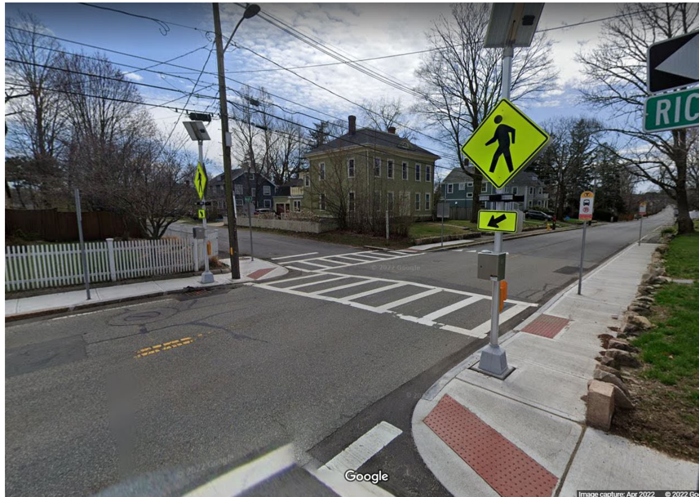
Recently reconstructed MBTA stop in Dedham
