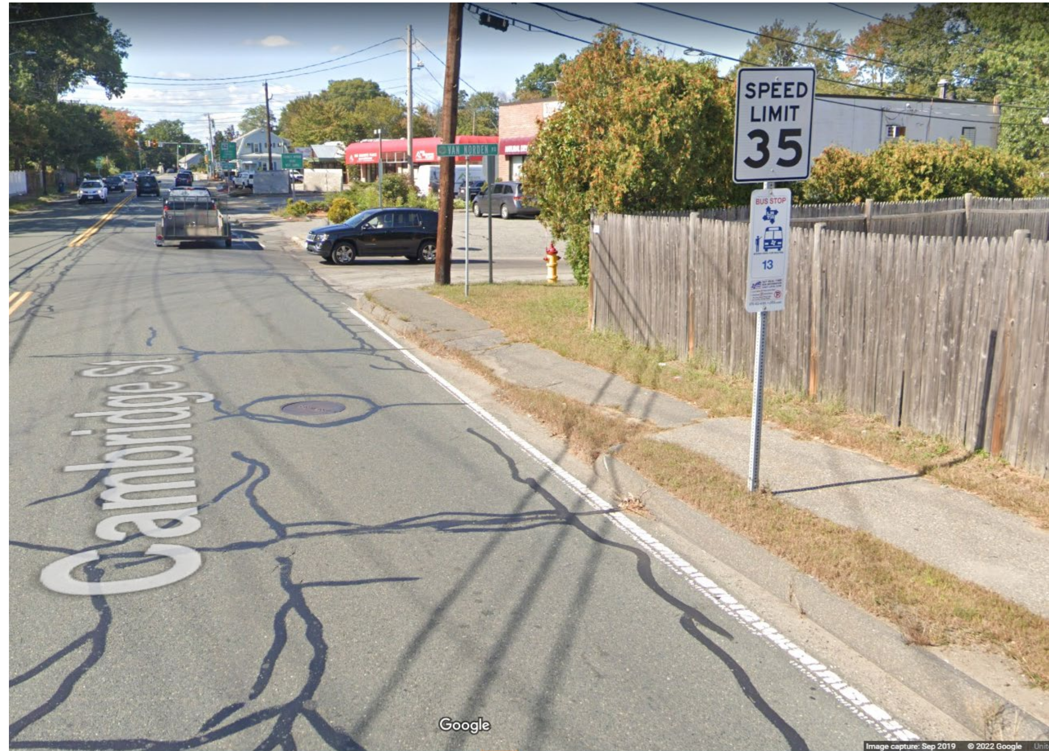
Existing northbound LRTA stop at Van Norden to be improved
