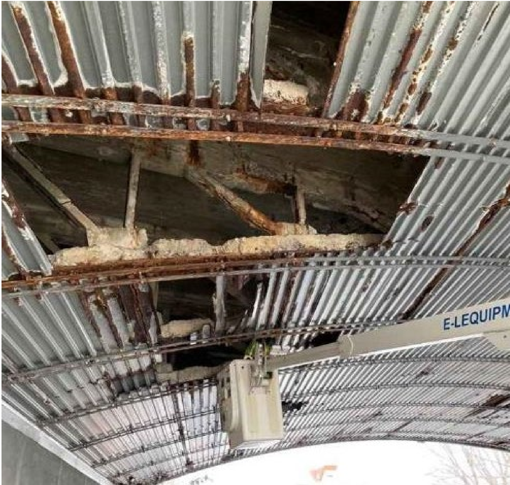
Superstructure frame concrete and steel deterioration
