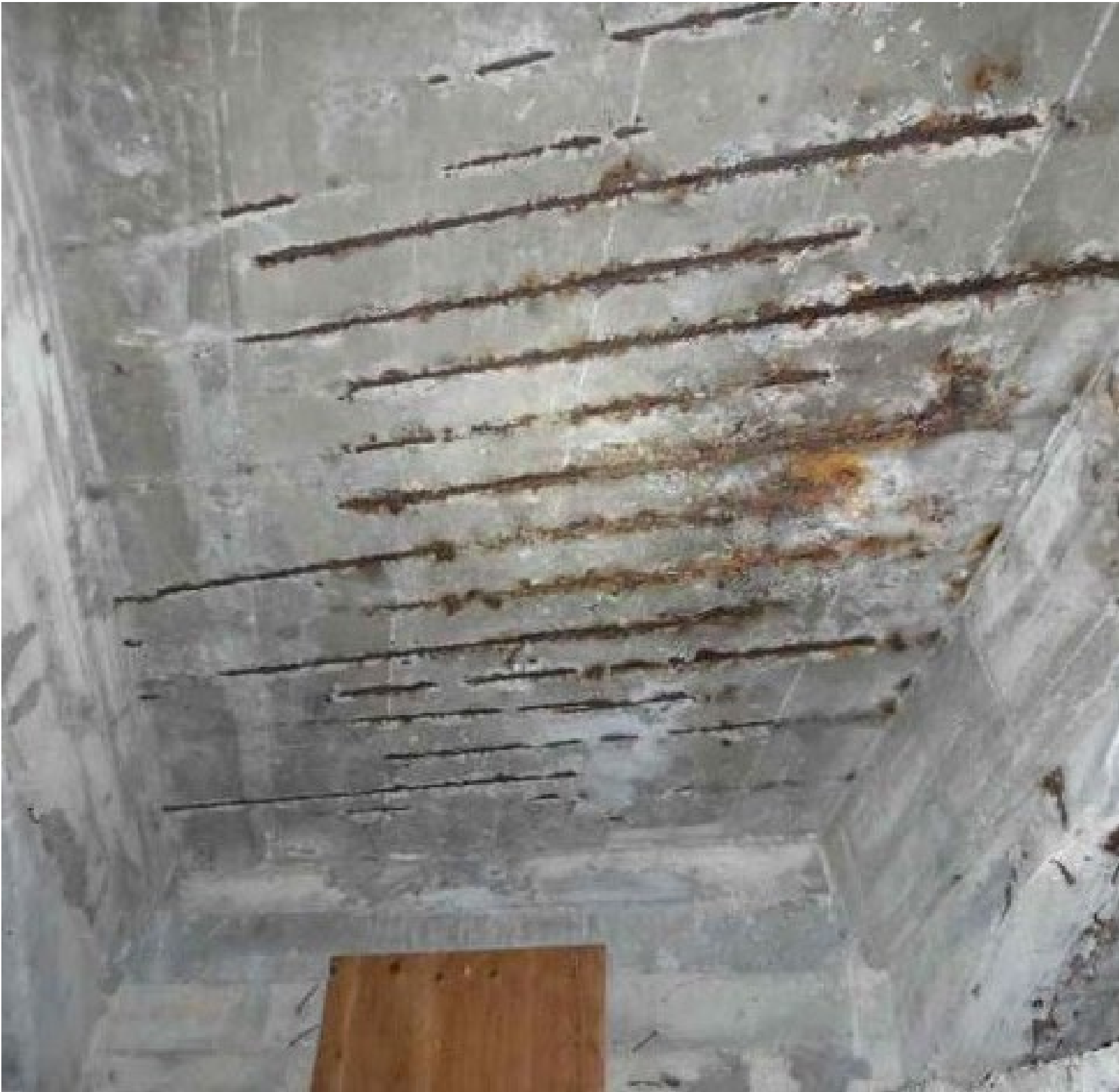
Deck Underside with exposed and deteriorated rebar
