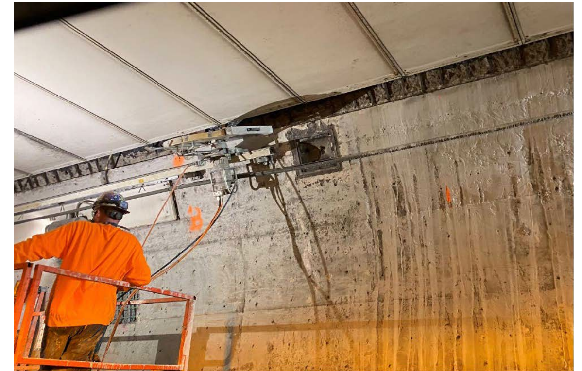
Keyway prep for precast arch panels
