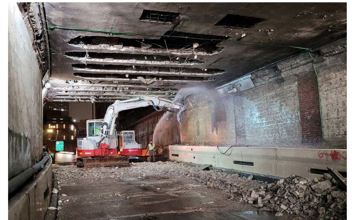
Box section ceiling demolition
