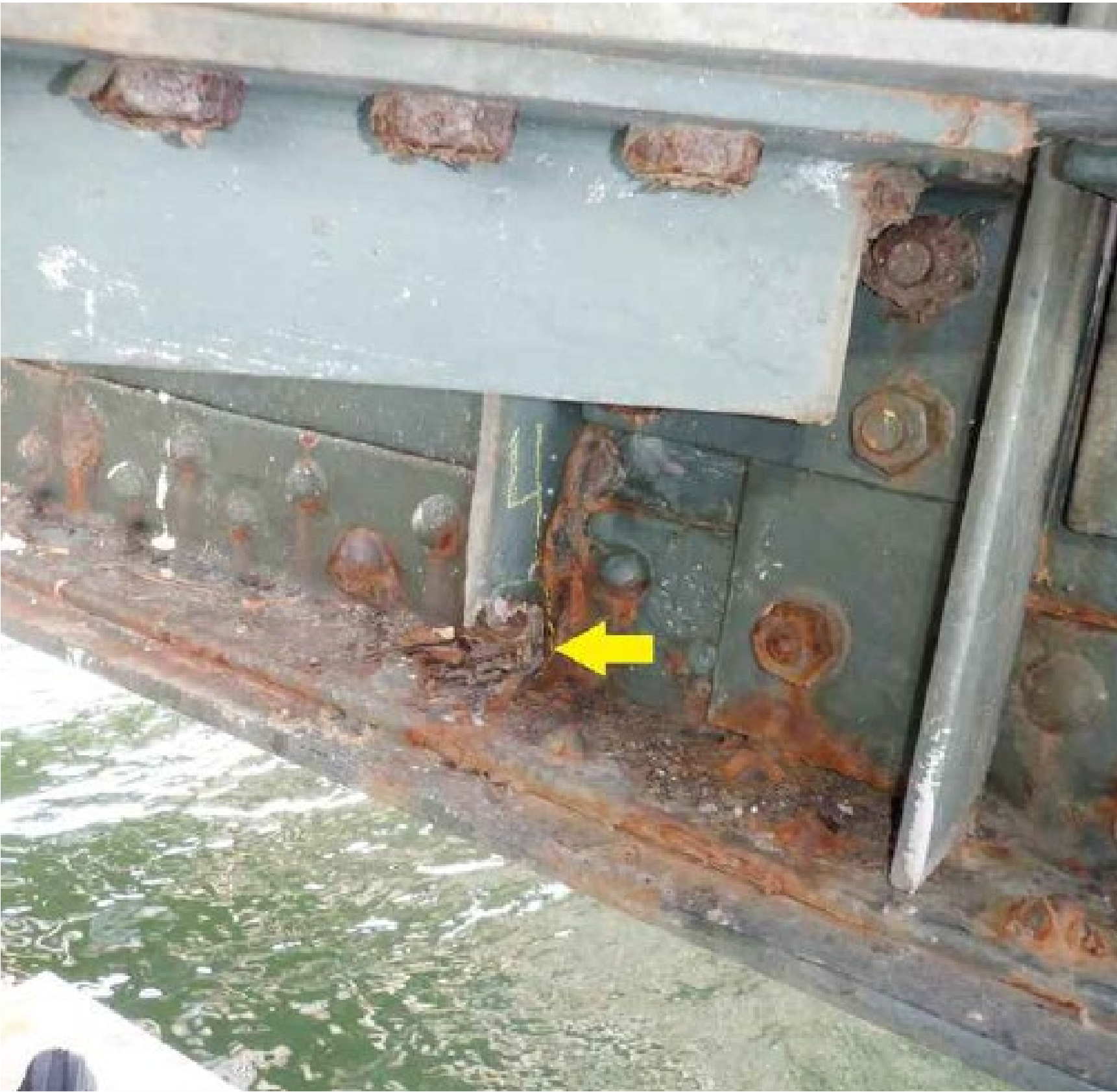
Floor System Corrosion
