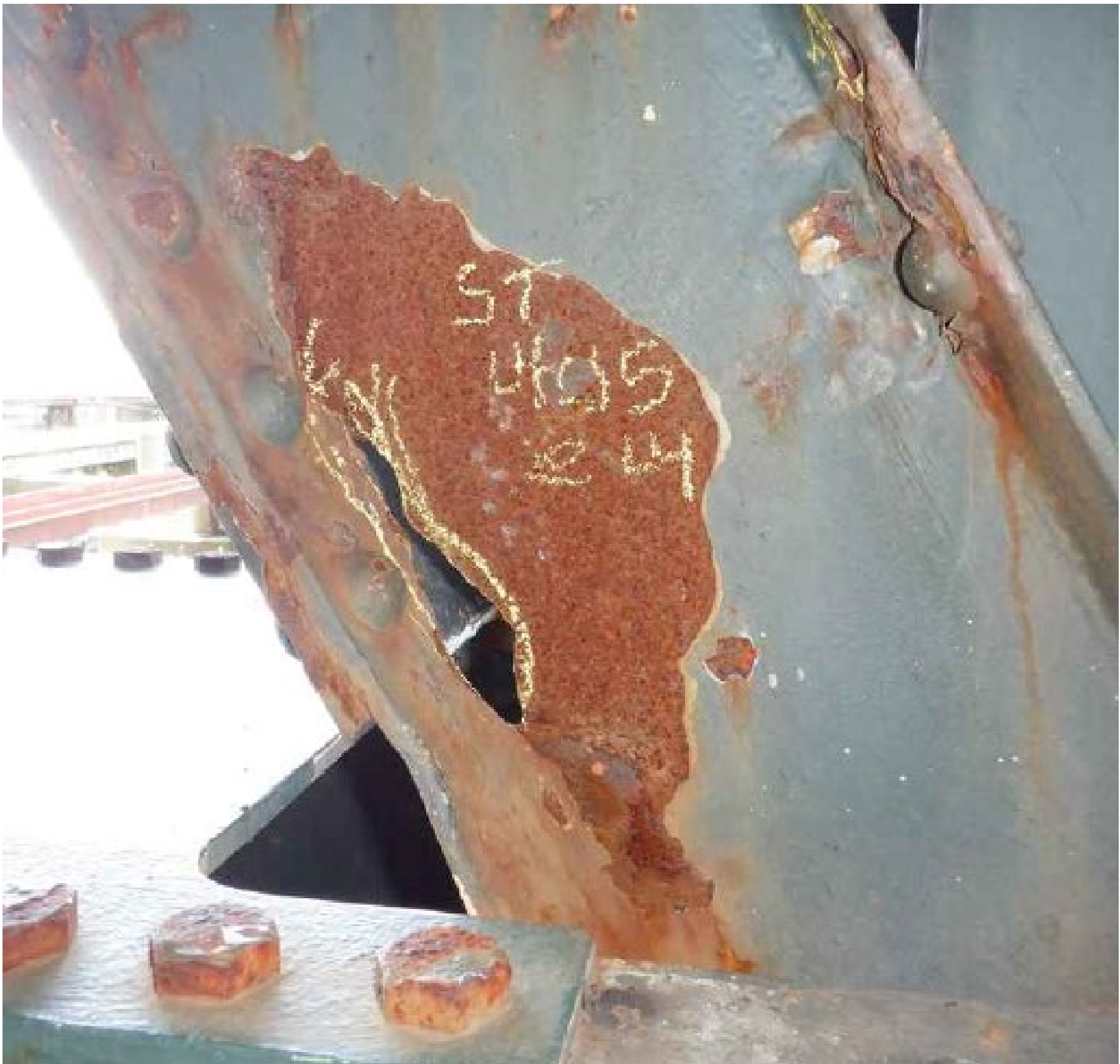
Truss Member Corrosion
