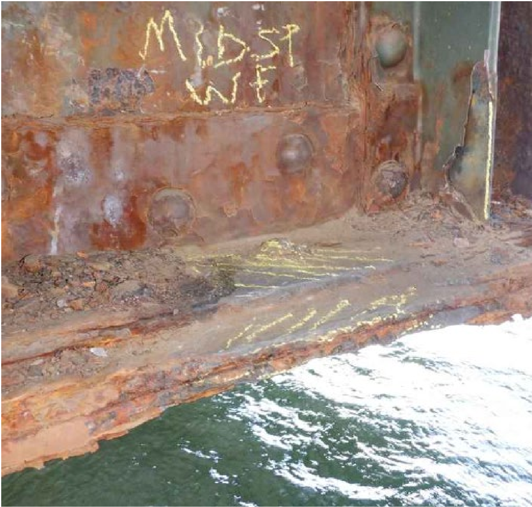
Floor System Corrosion
