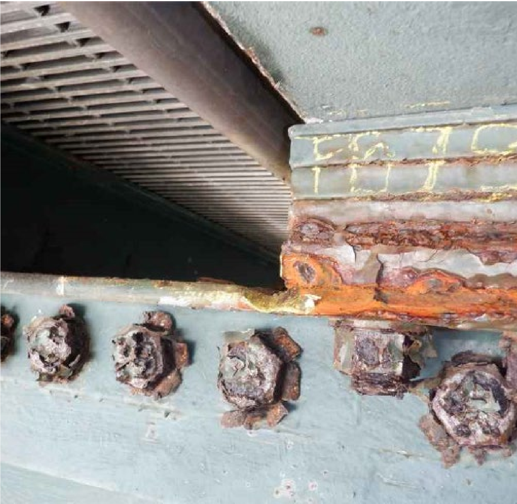
Deteriorated Bolts
