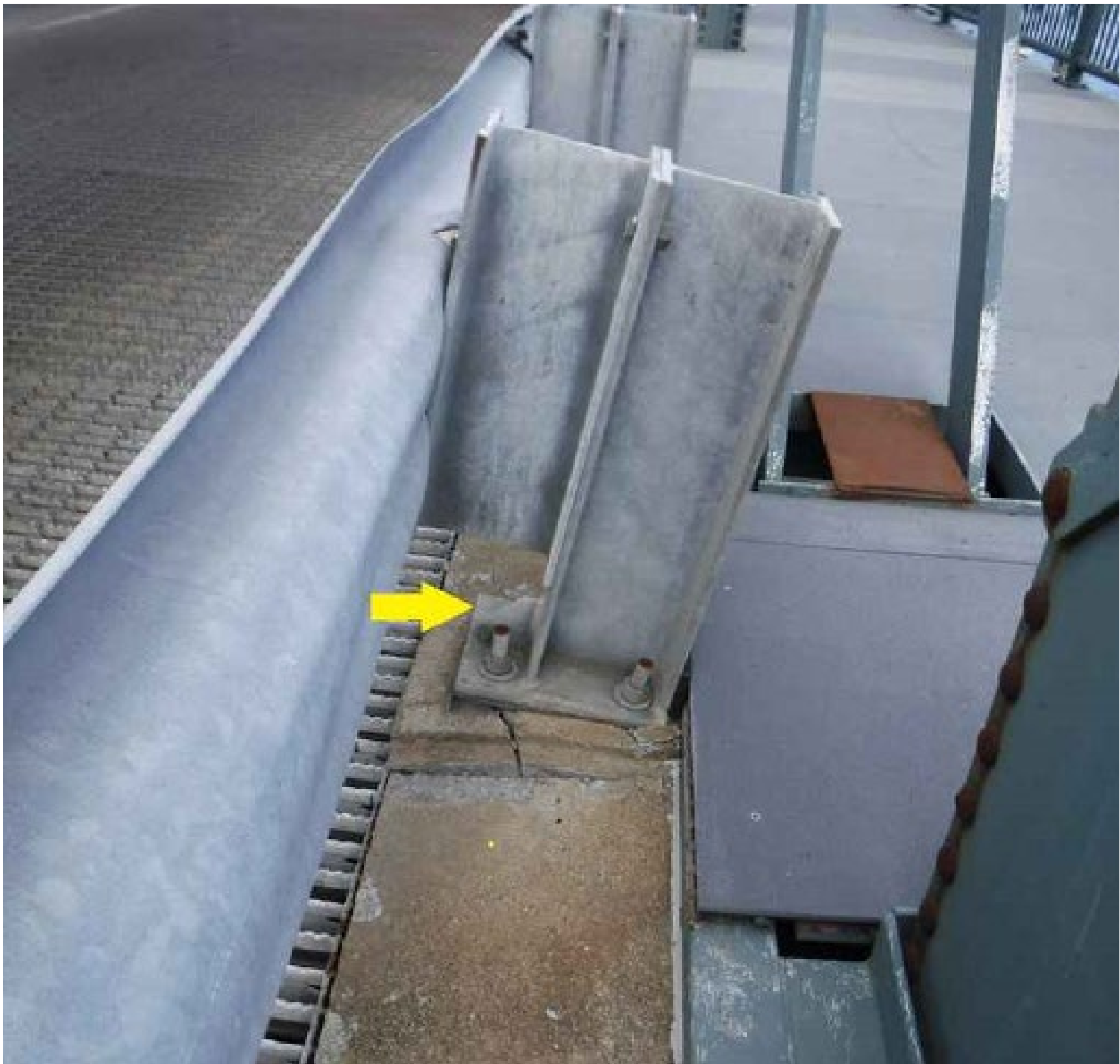
Guard Rail Impact Damage
