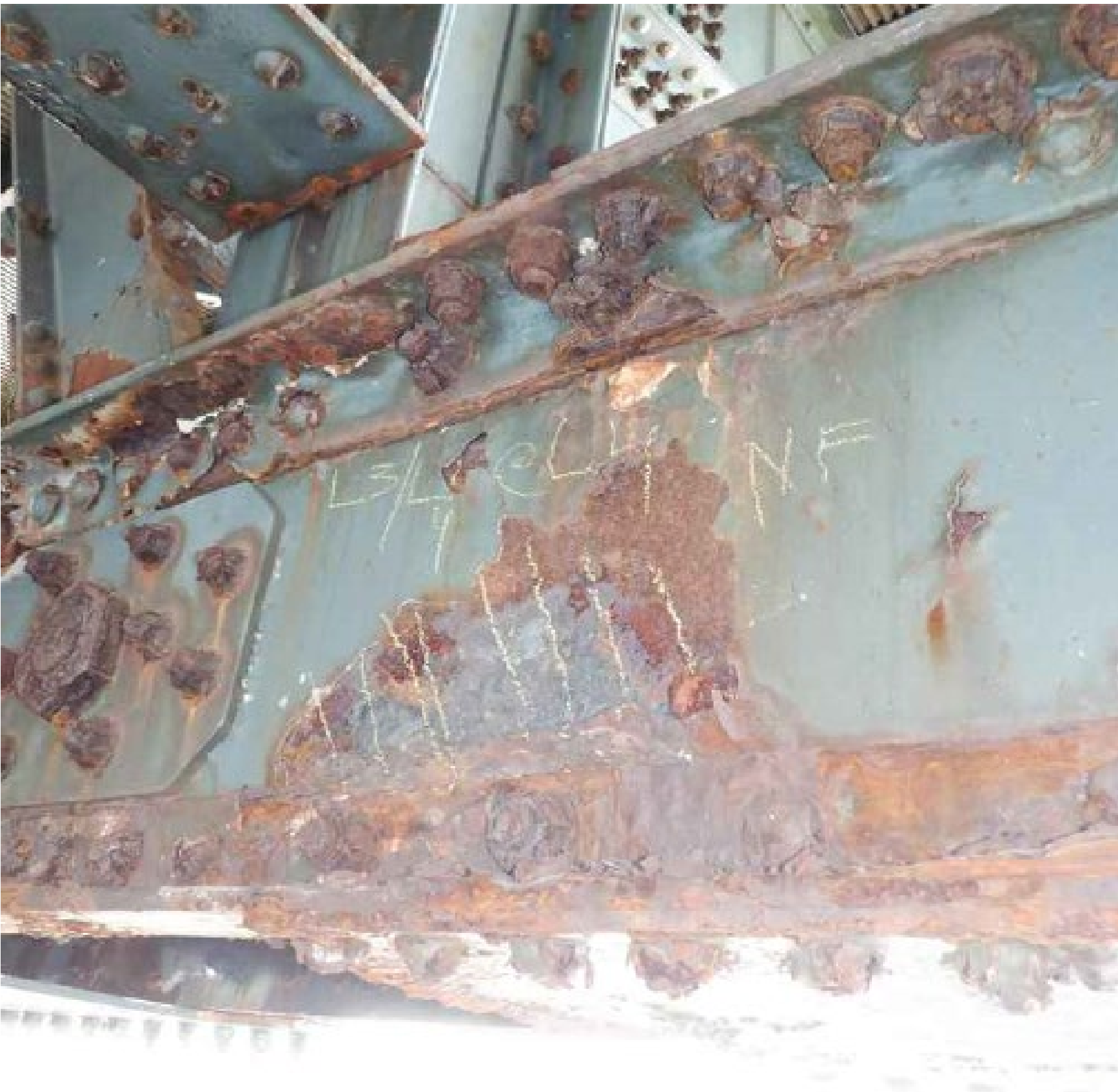
Truss Member Corrosion
