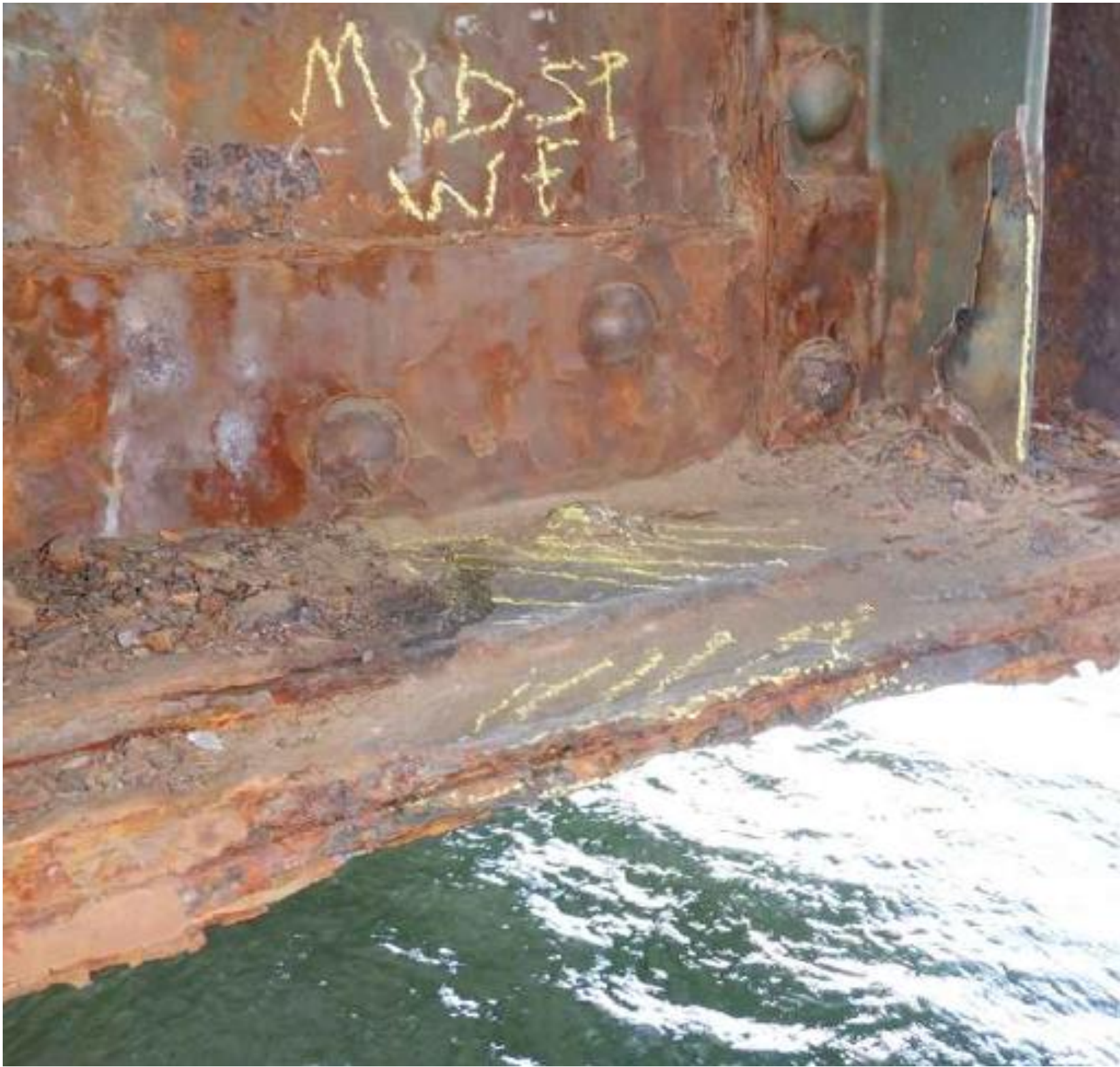
Floor System Corrosion
