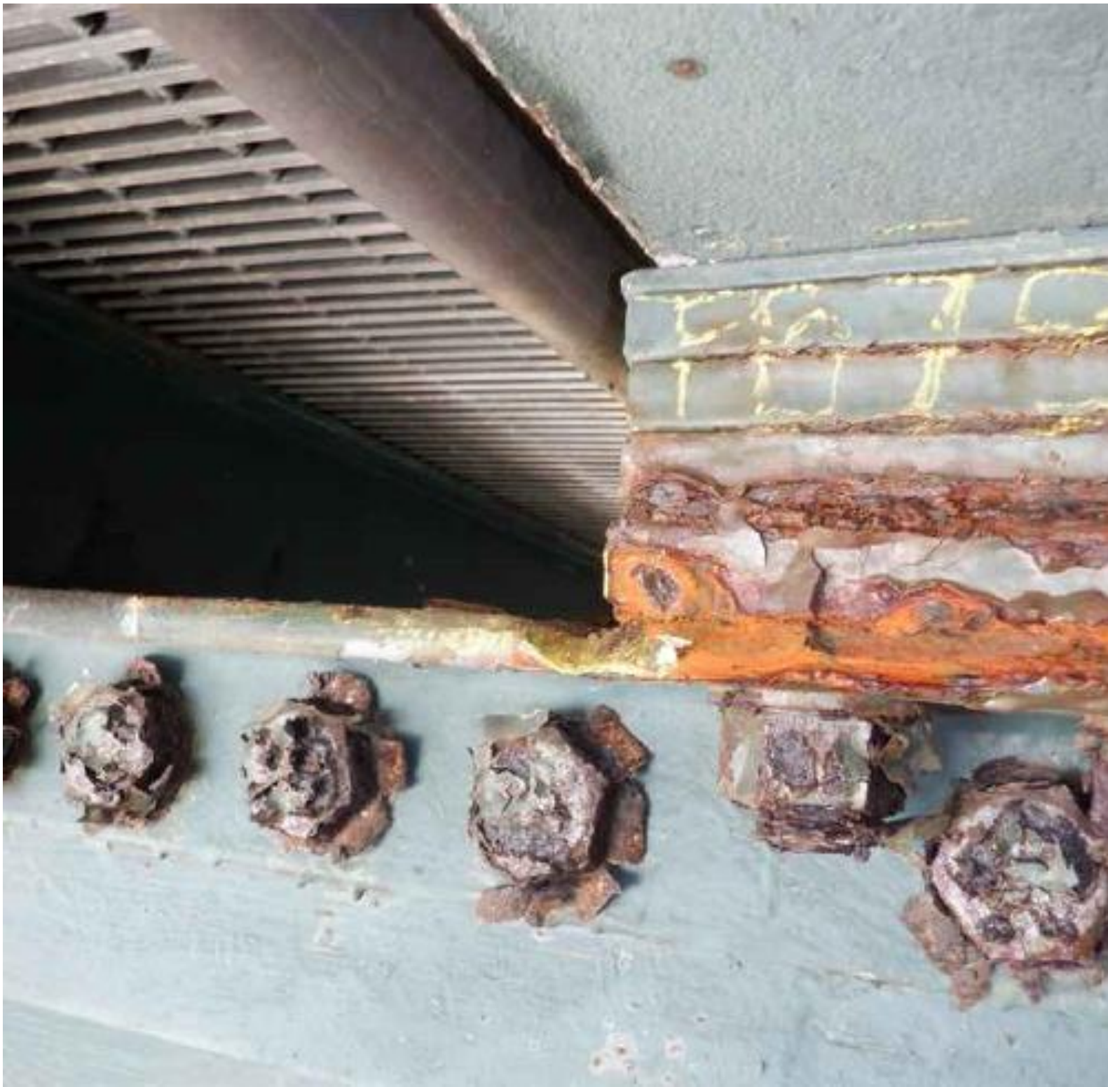
Deteriorated Bolts
