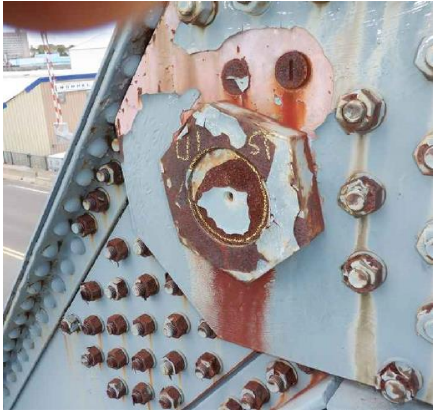
Failing Paint System
