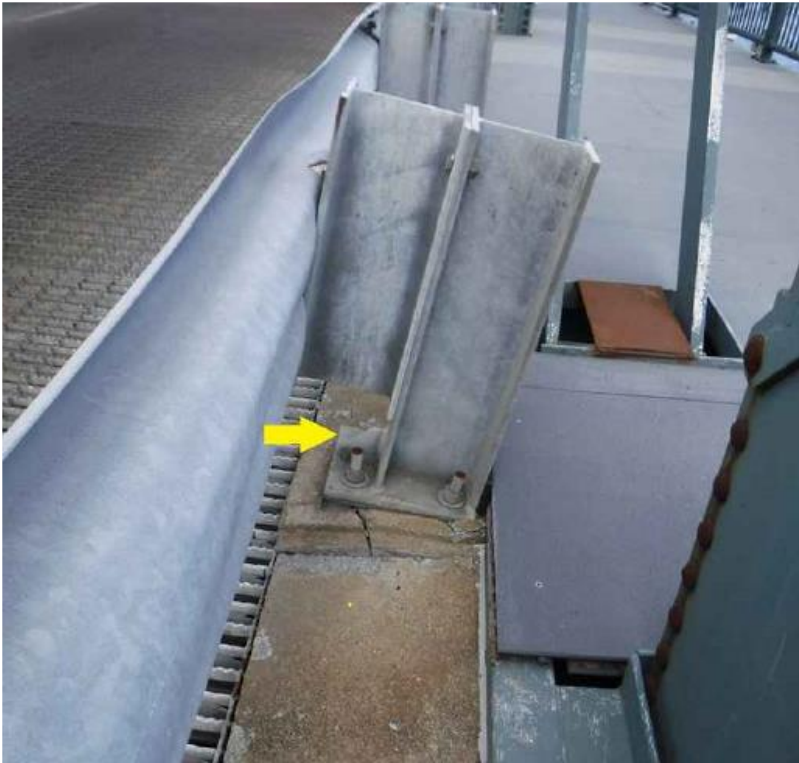
Guard Rail Impact Damage
