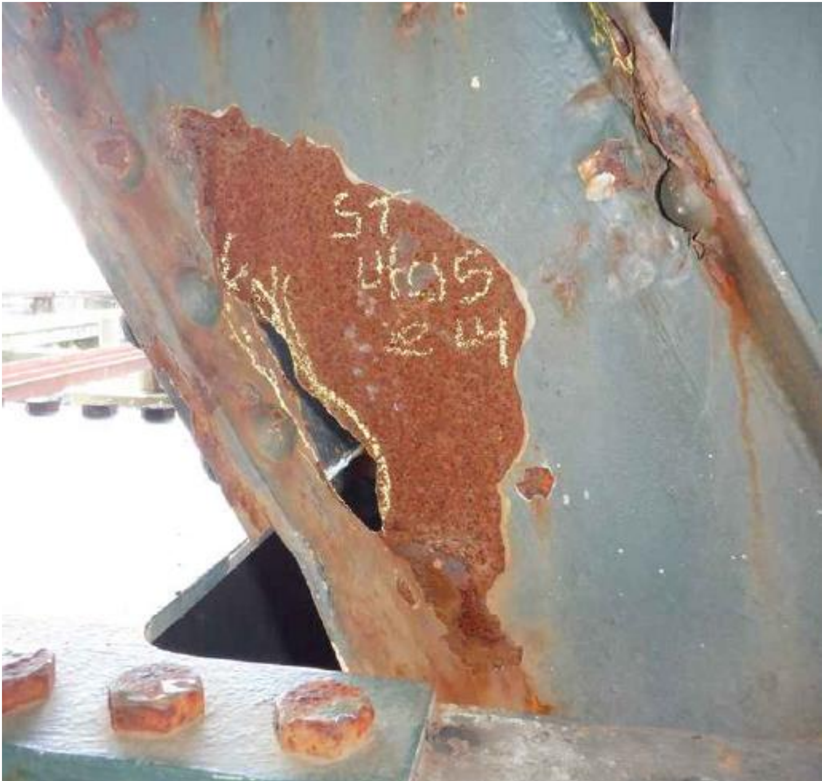
Truss Member Corrosion
