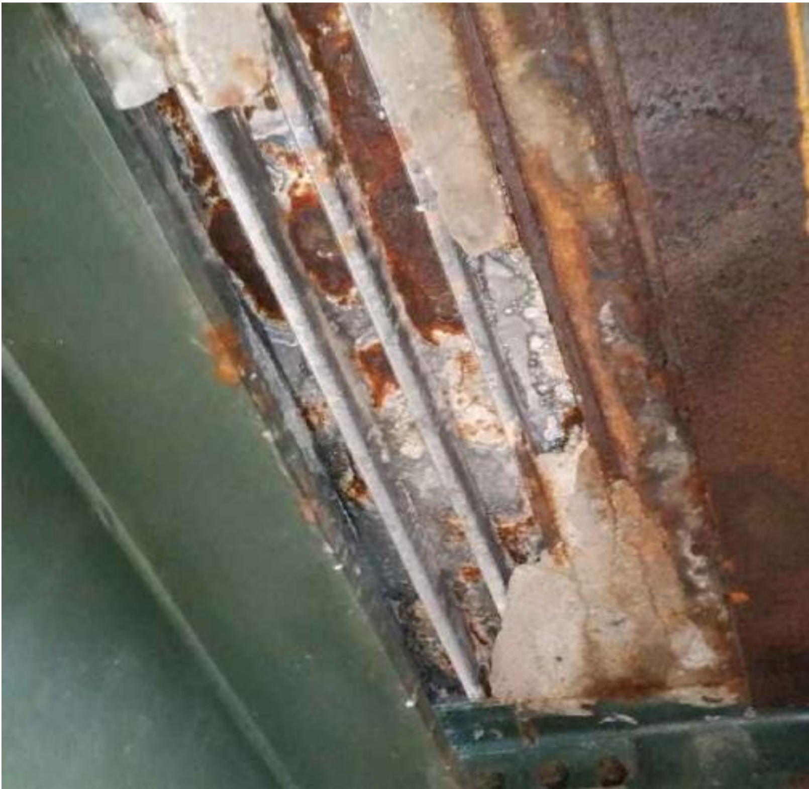
Deck Deterioration
