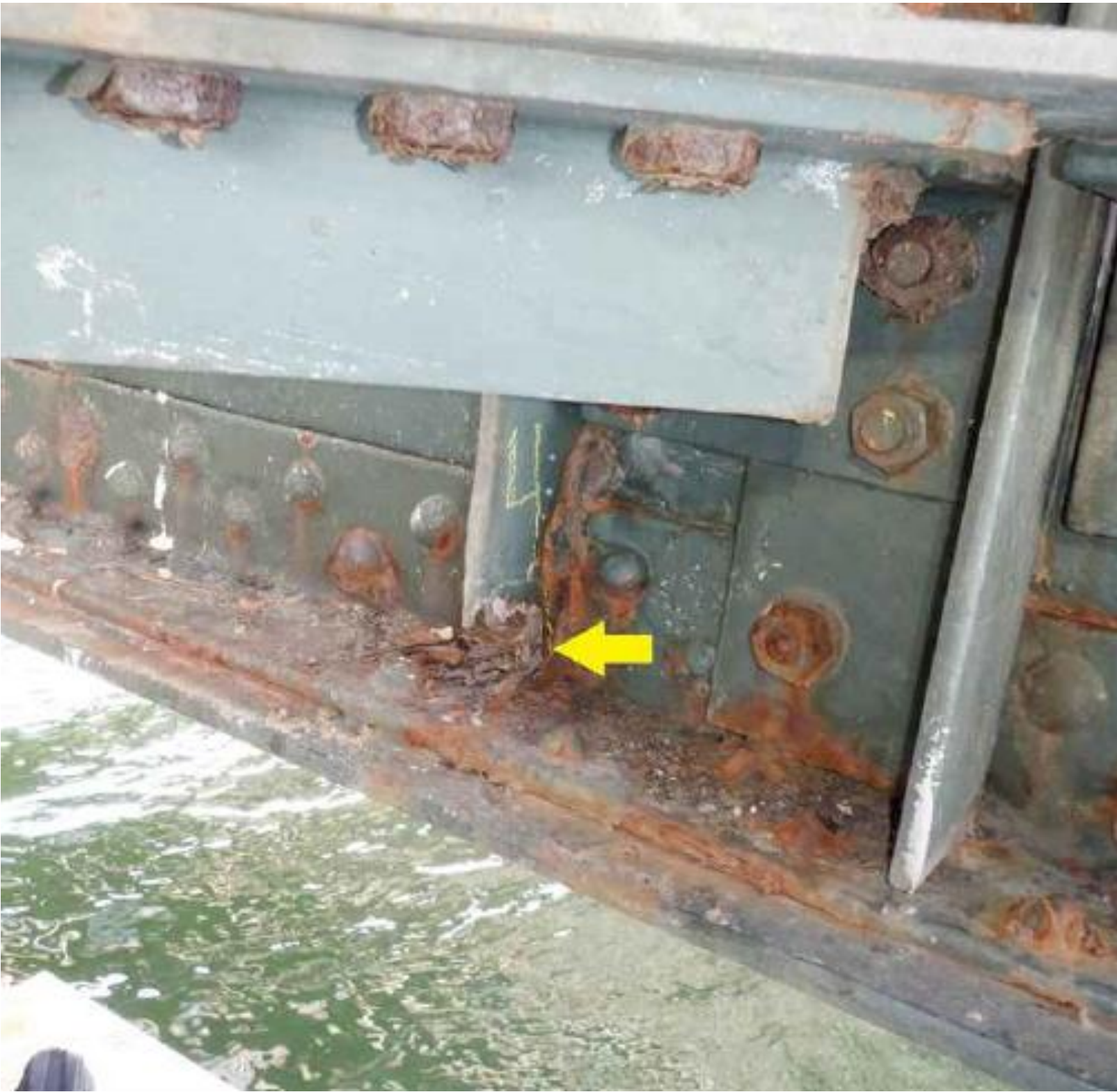
Floor System Corrosion
