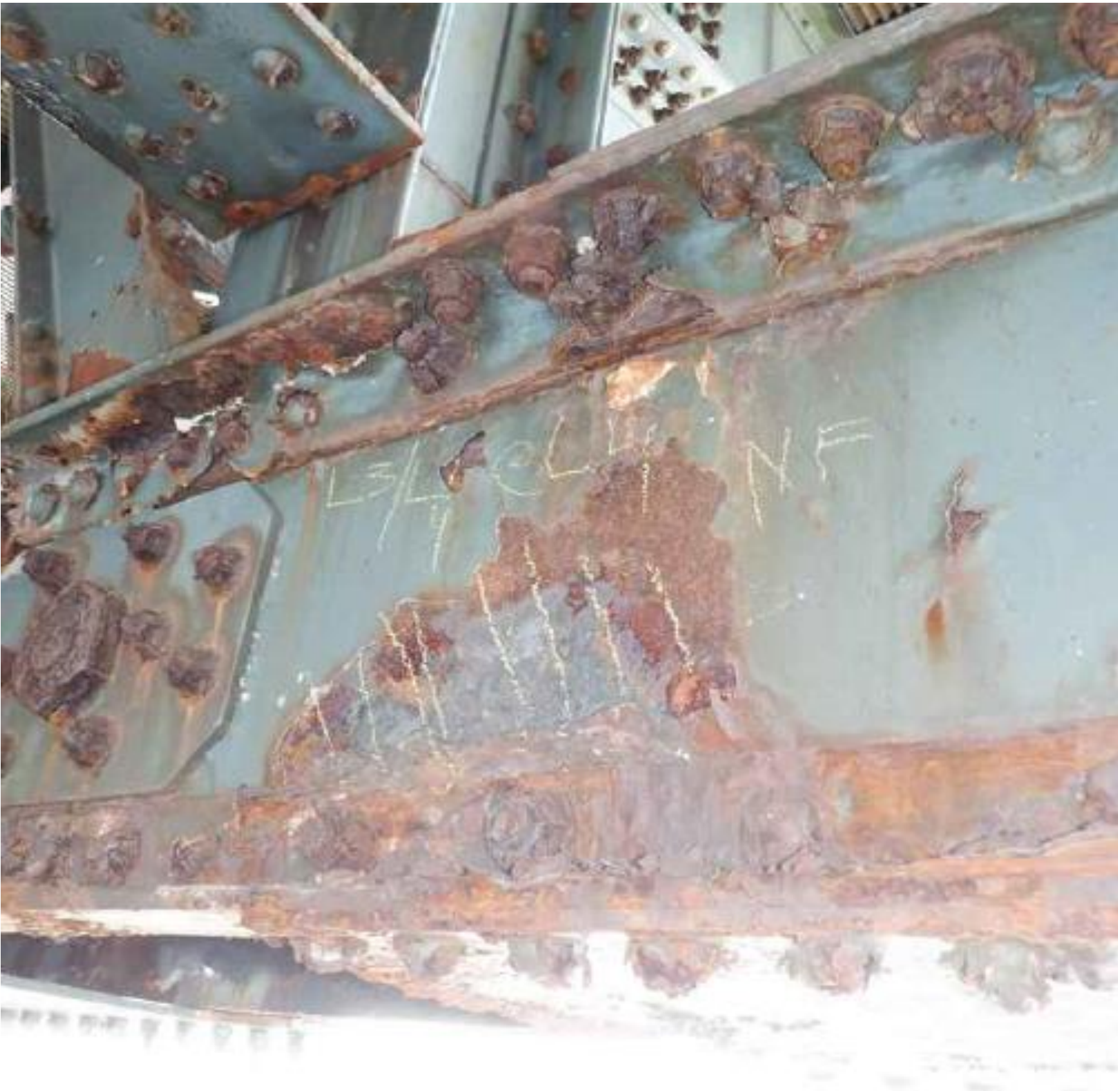
Truss Member Corrosion
