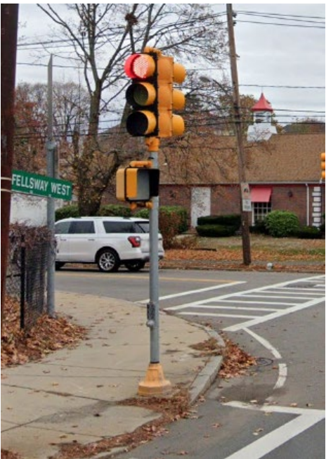
Pedestal mounted signal
