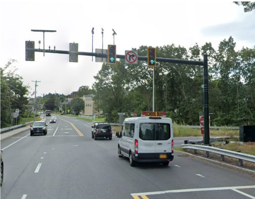
Overhead (mast arm) mounted signal
