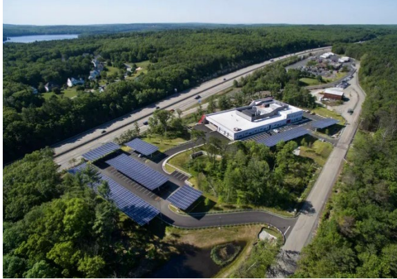
Solar panels at MassDOT Lab
