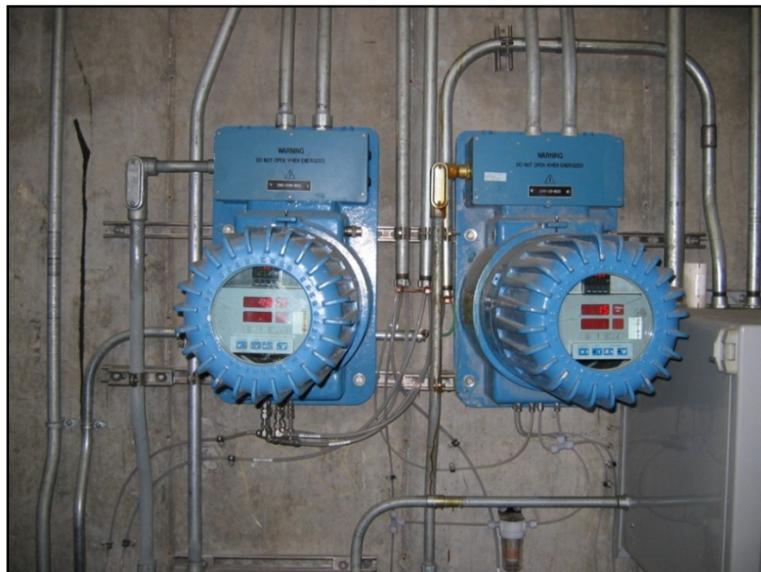
FIGURE 3-3: CO MONITORS LONGITUDINALLY FOR VENTILATED TUNNELS
