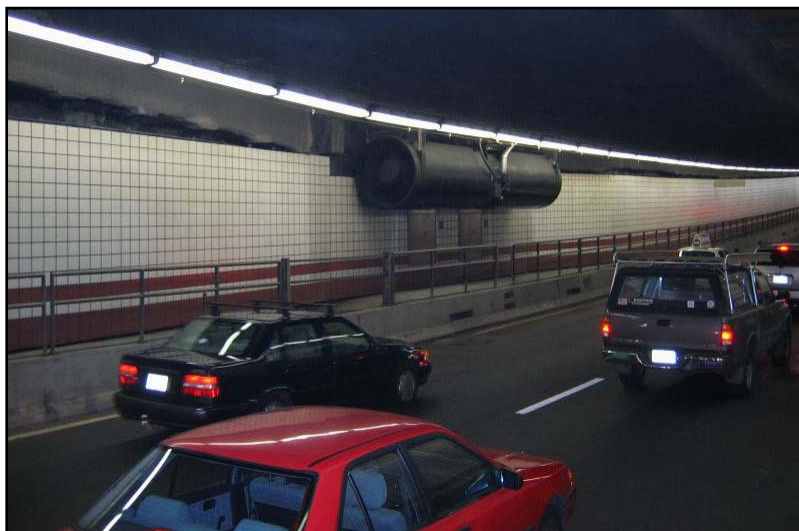
FIGURE 1-16: JET FAN AT LONGITUDINALLY VENTILATION RAMP
