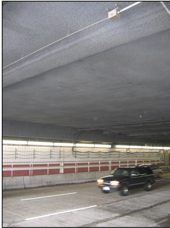
FIGURE 3-1: CO CEILING MONITORING PROBE AT DST
