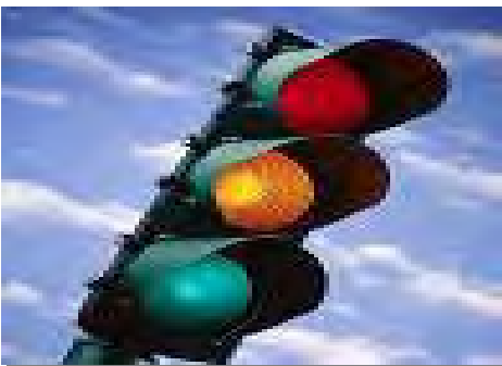
Traffic Lights and Streetlights
