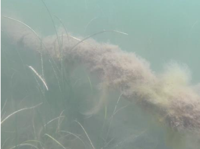
Figure 17. Floating, fouled rode at mooring 265
