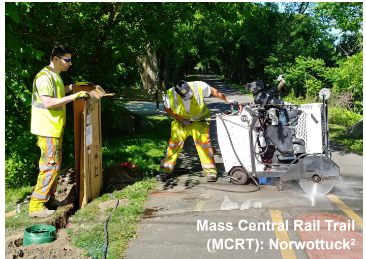
Sawcutting grooves into the pavement where the induction loops will go.
