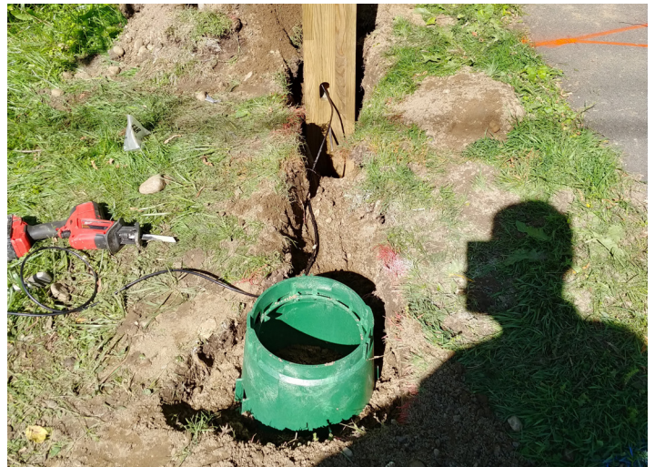
Post and handhole with trench for wiring.
