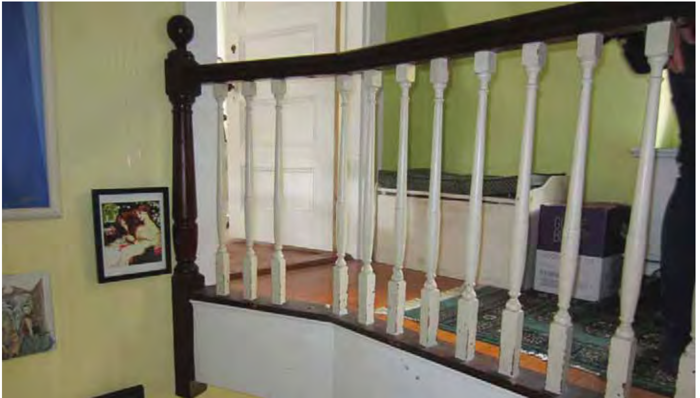
Image #45: 2nd floor guardrail with missing balustrades
