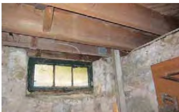
Image #31: Basement walls and first floor framing
