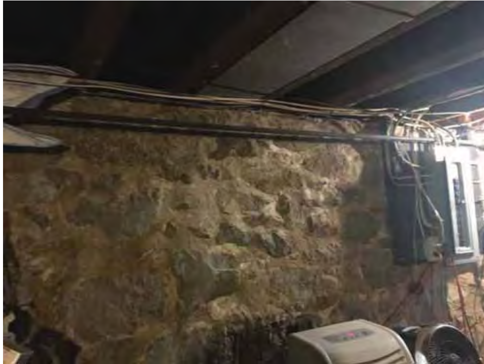
Photo 3 – Granite foundation wall viewed in the basement.
