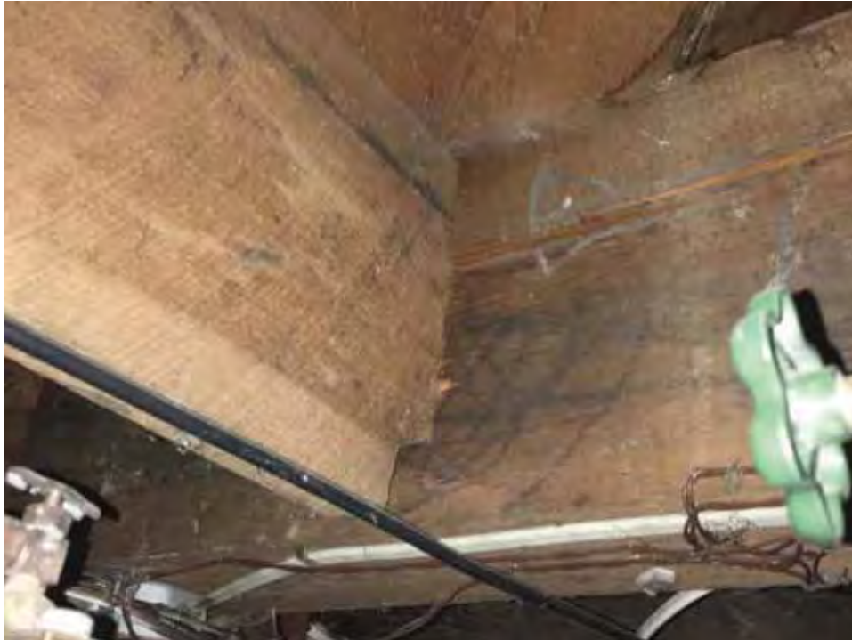
Photo 7 – First floor framing joist-to-beam connection
