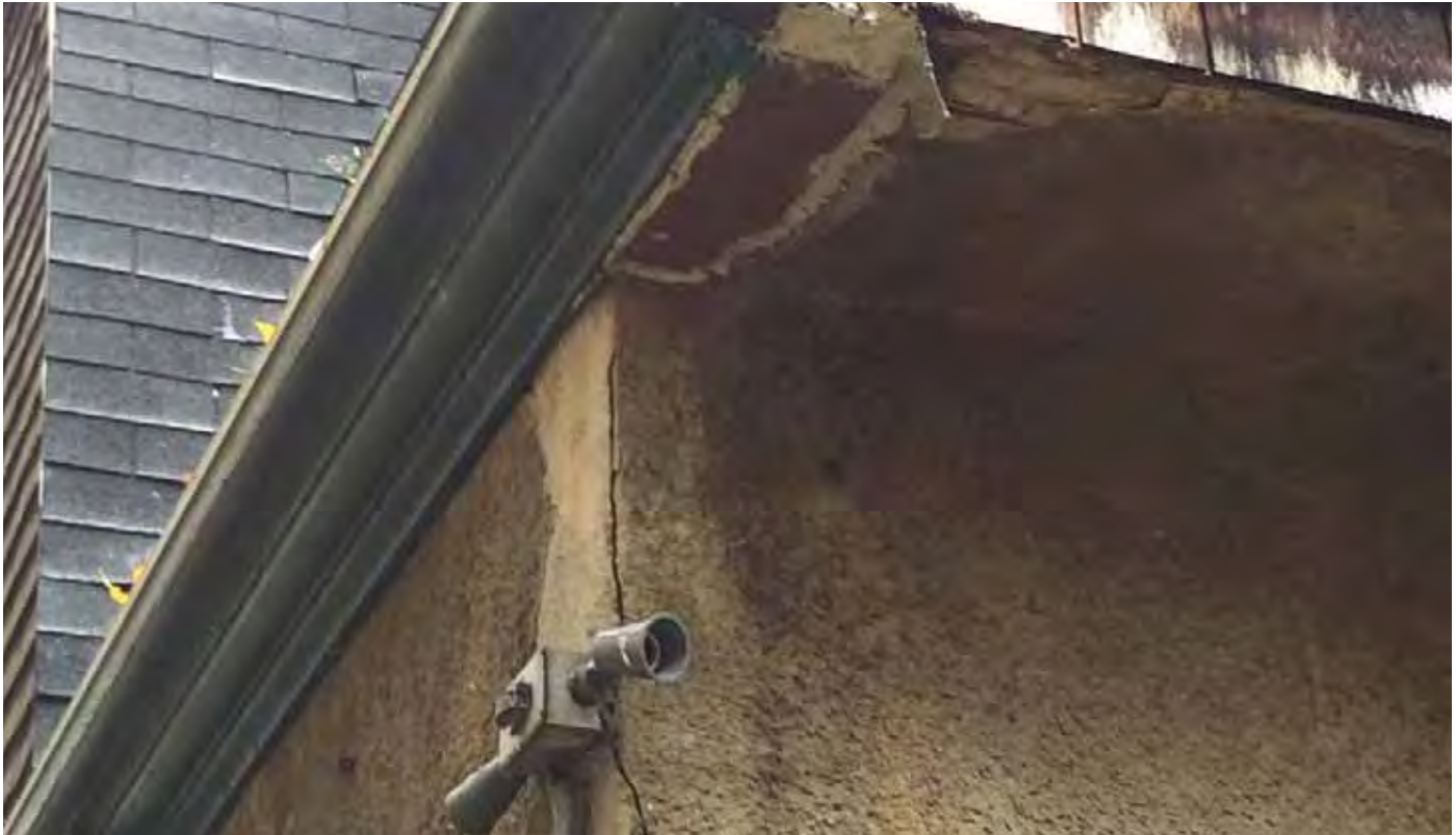
Image #22: Cracked stucco on northwest corner of house
