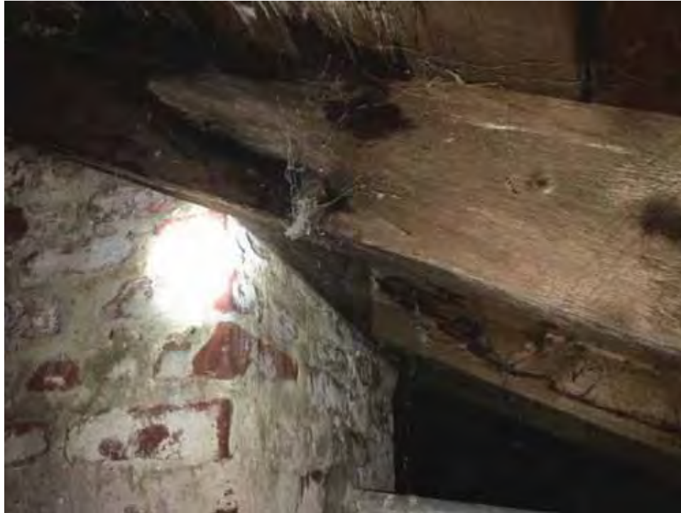
Photo 9 – Water staining on the main building roof framing.
