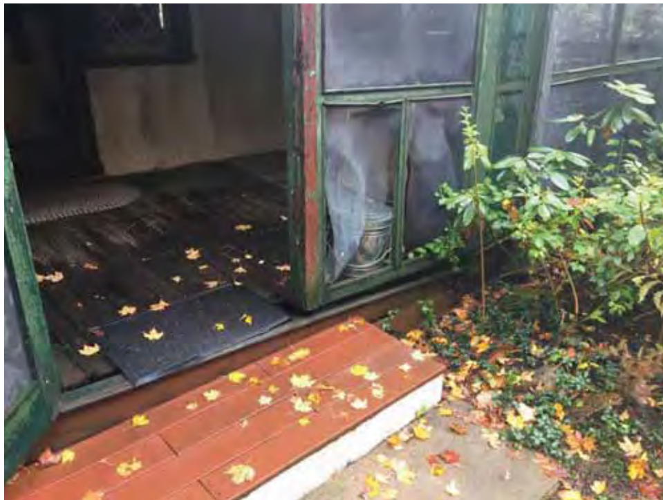
Photo 10 –Deteriorated framing at porch perimeter near the entrance.
