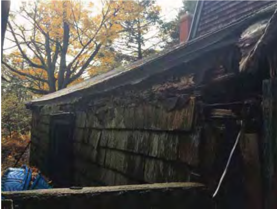
Photo 15 – Deterioration at the top of the attached shed's east wall.
