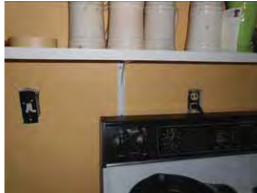
Outlet & Switch Without Cover
