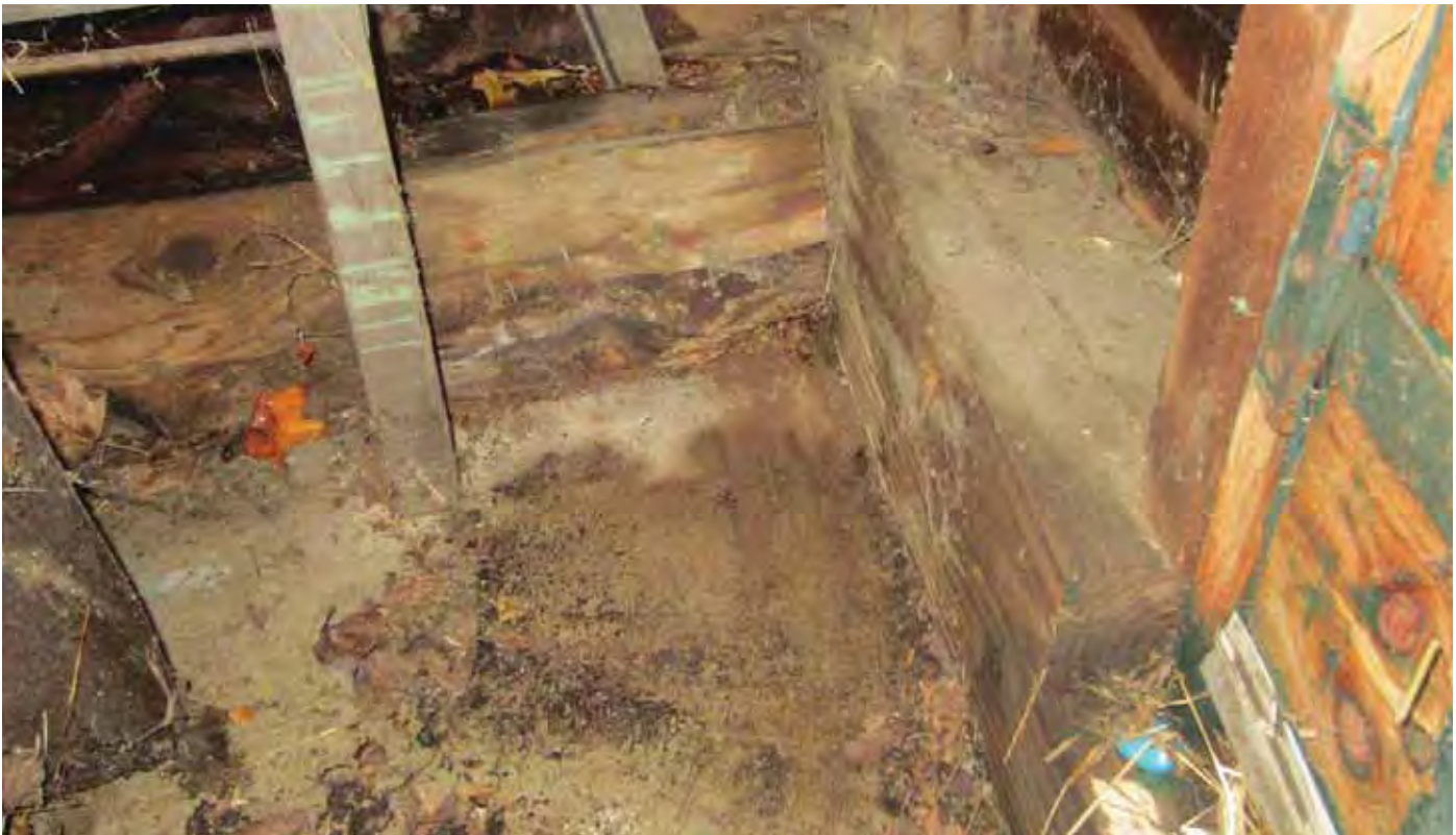
Image #27: Rotted framing in shed at southeast corner
