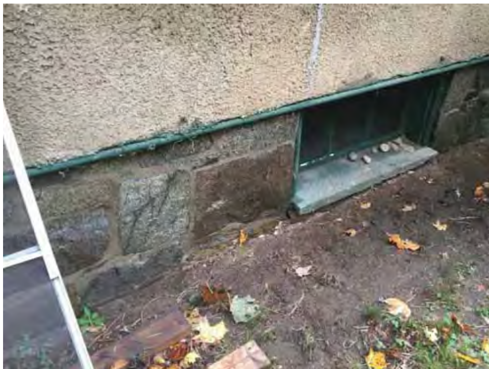
Photo 2 – Granite foundation wall exterior face at the north elevation.
