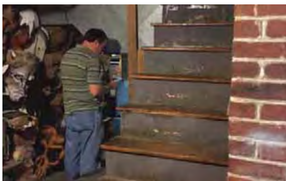
Image #50: Basement stair with no handrail
