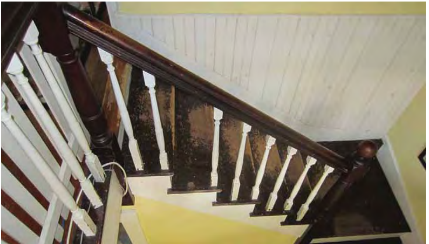
Image #46: Main stair with worn treads and missing railing balustrades
