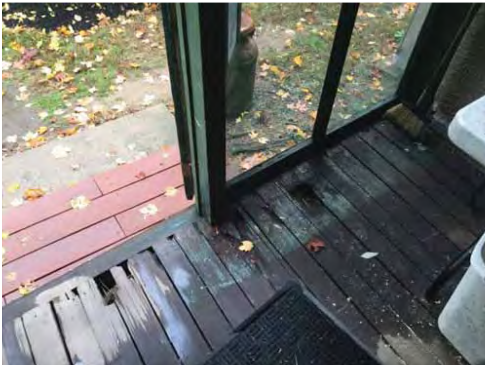
Photo 12 – Deteriorated decking at the porch perimeter near the entrance.
