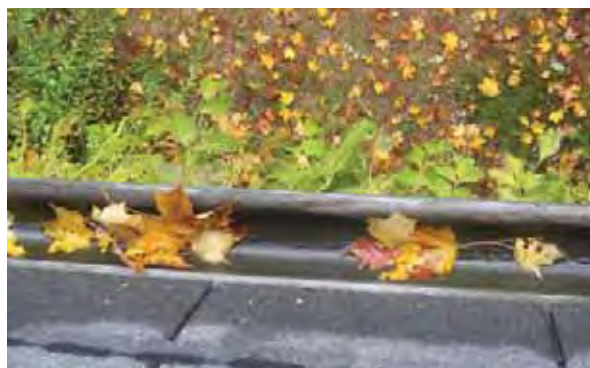
Image #19: Existing wood gutter with no lining
