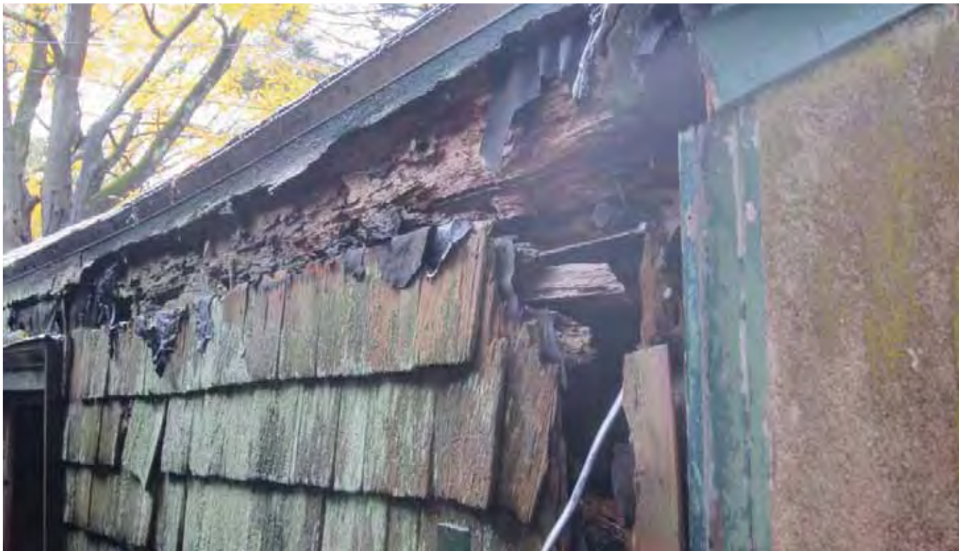
Image #51: Deteriorated east wall of shed
