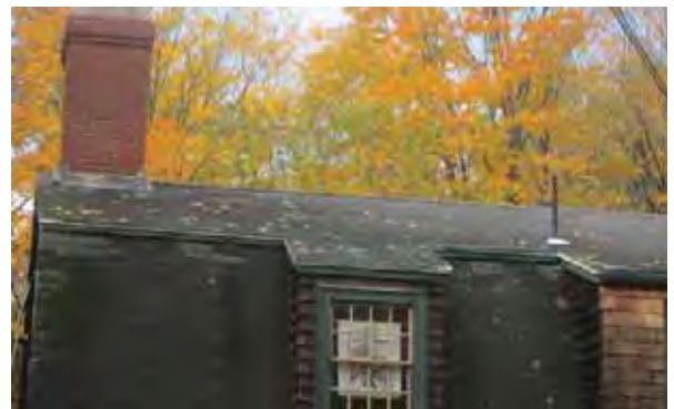
Image #13: Missing asphalt shingles at gambrel breakline, deteriorating trim
