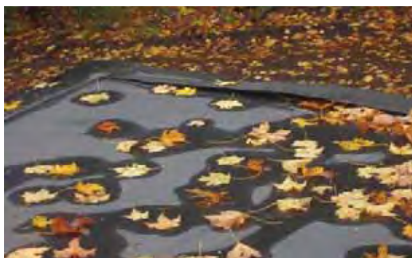
Image #17: Failing membrane roofing on porch
