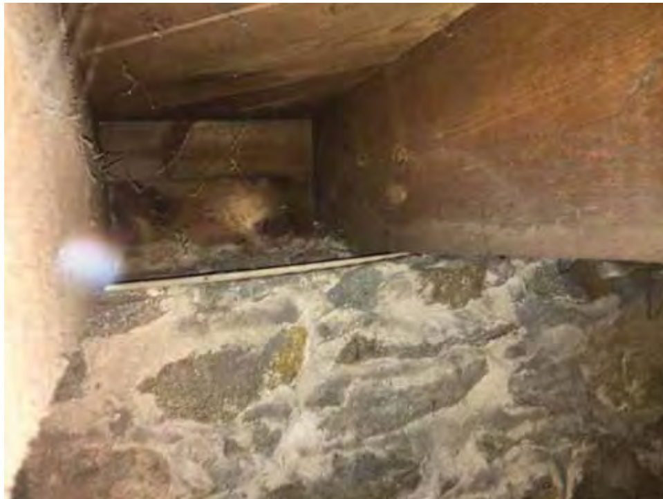
Photo 6 – First floor joists bearing on the granite foundation walls.
