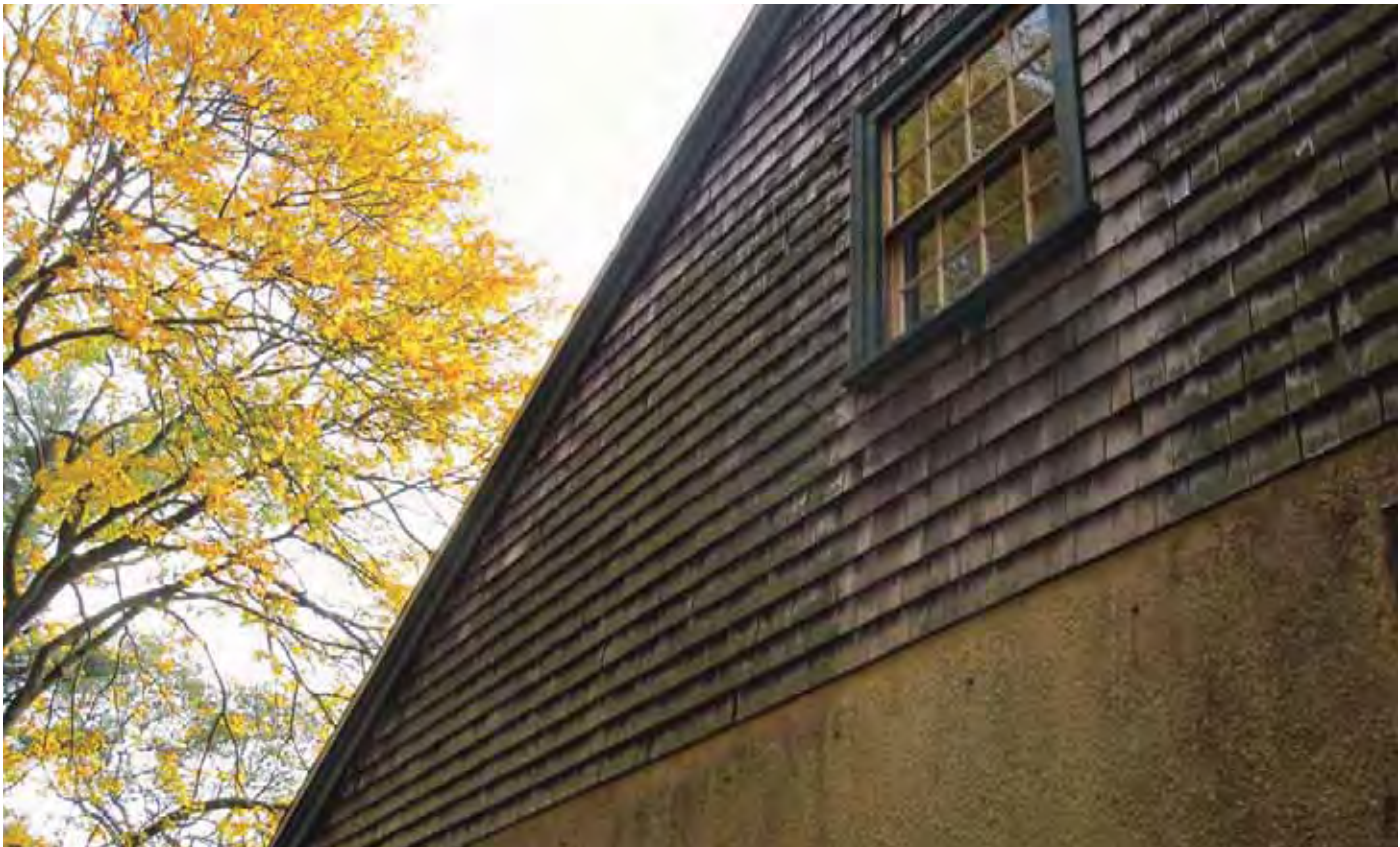
Image #21: Stained shingles on north elevation
