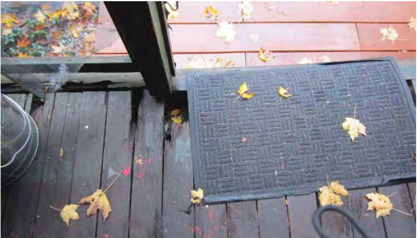
Image #28: Front porch deterioration at front steps
