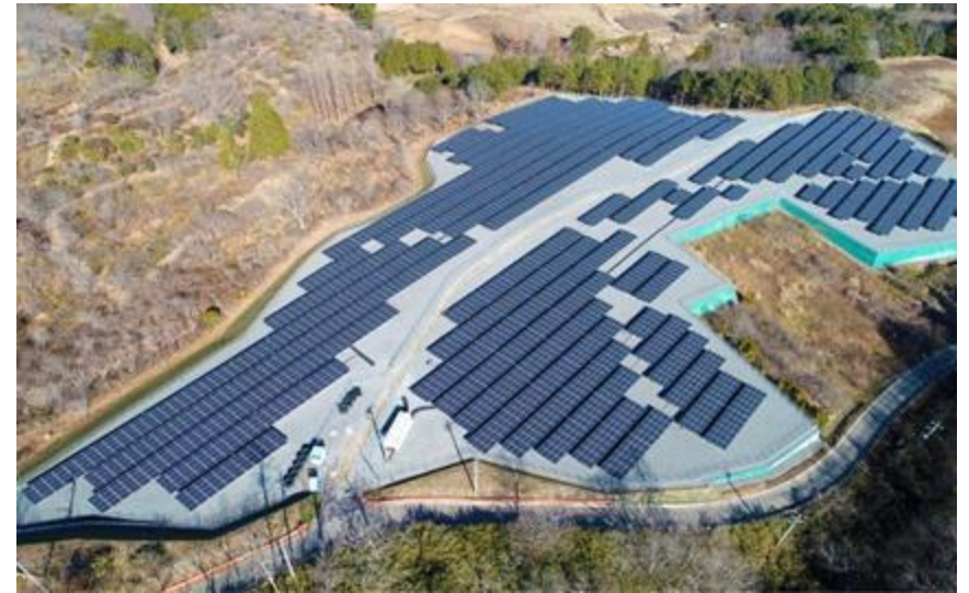
2 MW Class III Facility
