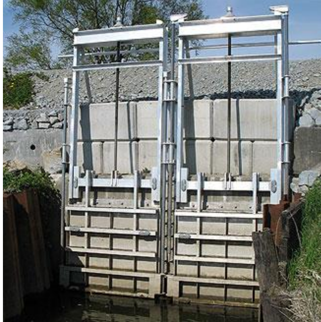
Figure 15 Golden Harvest GH-50 sluice-flap combination gate.
