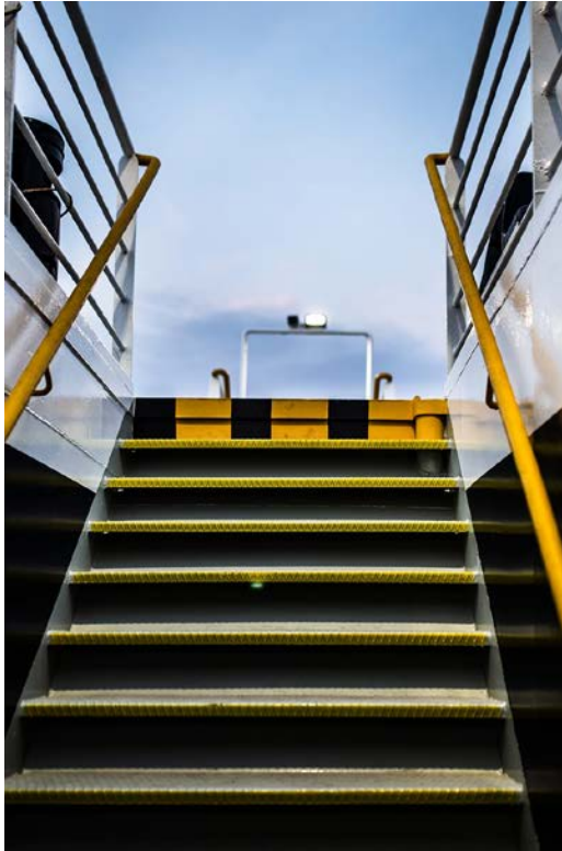
Figure 5. This view of a stairway shows contrasting railings on both sides and contrasting strips along the treads. 55
