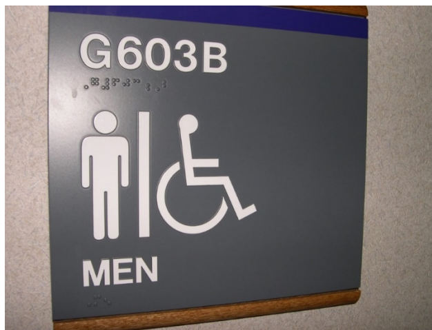
Figure 1. This ADA-compliant men's toilet room sign has good contrast, universal symbols for men, and the International Symbol of Accessibility, as well as braille and raised lettering. A person with some vision may be able to stand close enough to read it. Experts argue that the braille and raised lettering are not widely used by people with vision disabilities.
