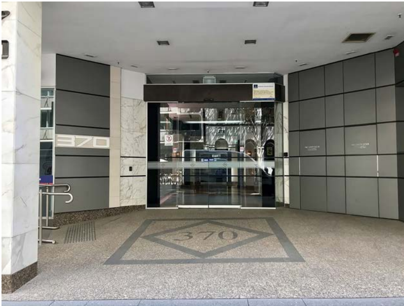
Figure 3. This photo shows an exterior view of a building entrance that is likely confusing and difficult to navigate for a person with low vision. The address is located in two places that are difficult to see: on a wall, with stretched numbers that do not contrast well with their background, and on the floor, which would be easy to miss. Glass entry doors are so reflective that it is almost impossible to see where to enter, despite some glass manifestation. 47
