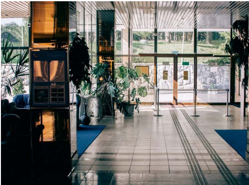
Figure 4. Helpful features include detectable floor strips leading to/from the entry/exit doors. However, there is a stanchion blocking access to the exit door from the inside and to the inside from the entry door. There are some variations in floor materials that may be useful, including a walk-off mat near the entrance/exit and both smooth and matte tiles. Potentially problematic features include reflective column materials that provide glare, large expanses of glass, and a reflective ceiling.
