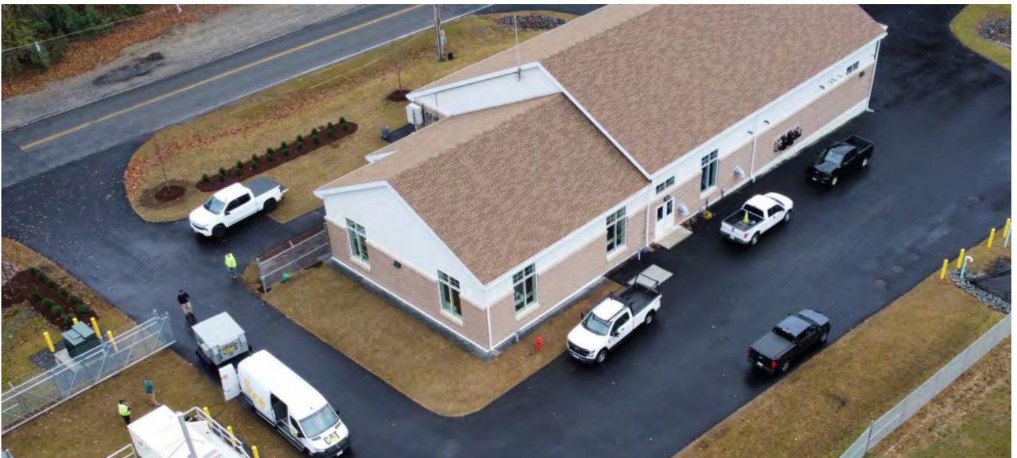
Source: MassDevelopment, Devens Water Treatment Plant
