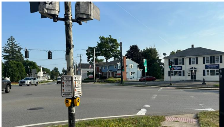
Route 9 features many areas with consecutive or extremely wide curb cuts that interrupt sidewalks
