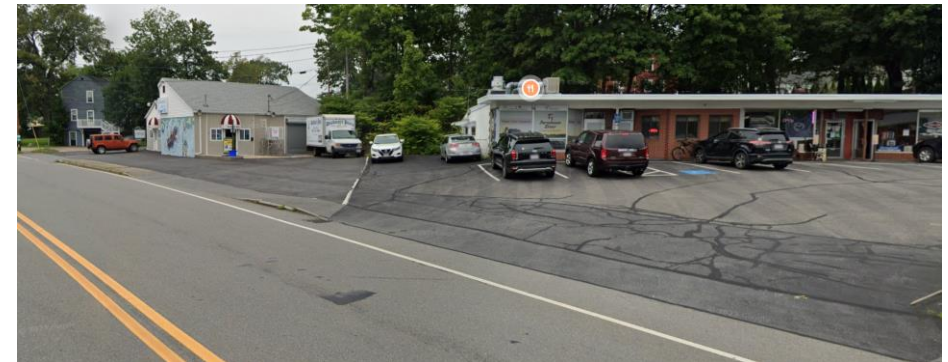
The S. Main St./Route 9 intersection is intimidating to cross and the Crosswalk in need of re-stripping for visibility
