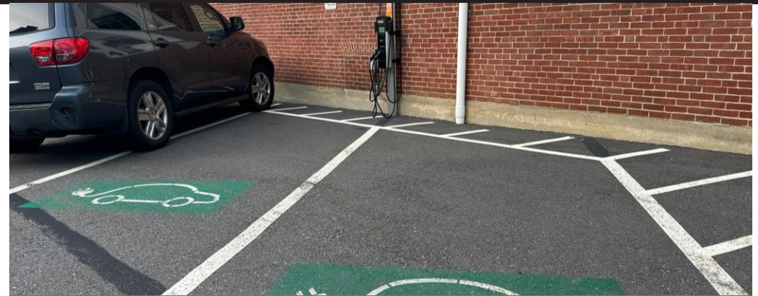
Electric vehicle parking and charging areas at the Town Hall lot
