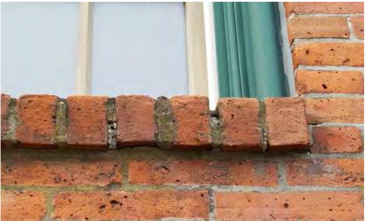
TYPICAL EXAMAPLE OF DETERIORATED ROXLOC BRICK SILLS
