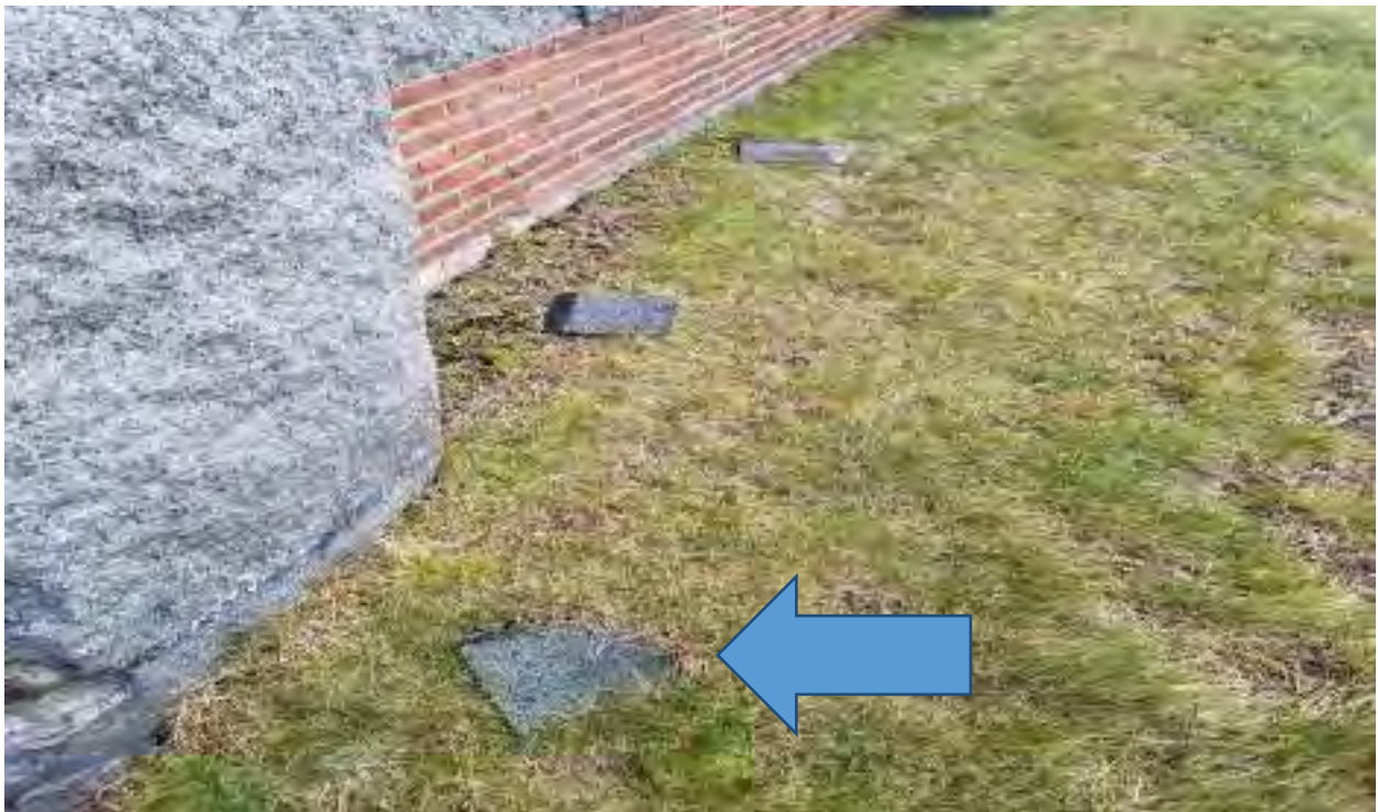
FALLEN ASPHALT SHINGLED SCATTERED AROUND BUILDING PERIMETER
