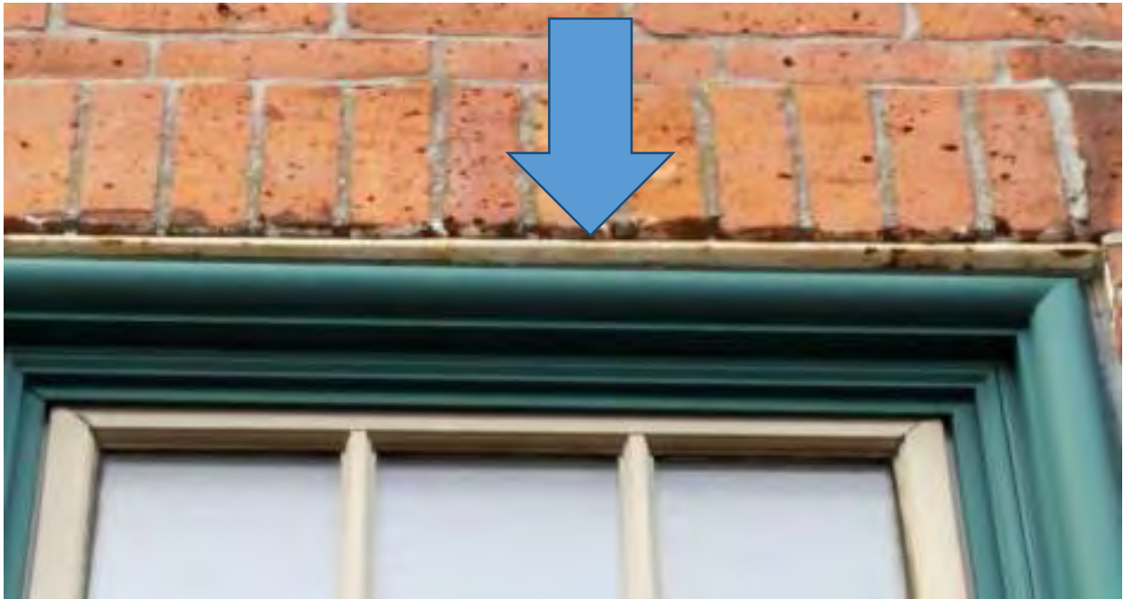
TYPICAL STEEL LINTEL NEEDING SCRAPE & PAINT
