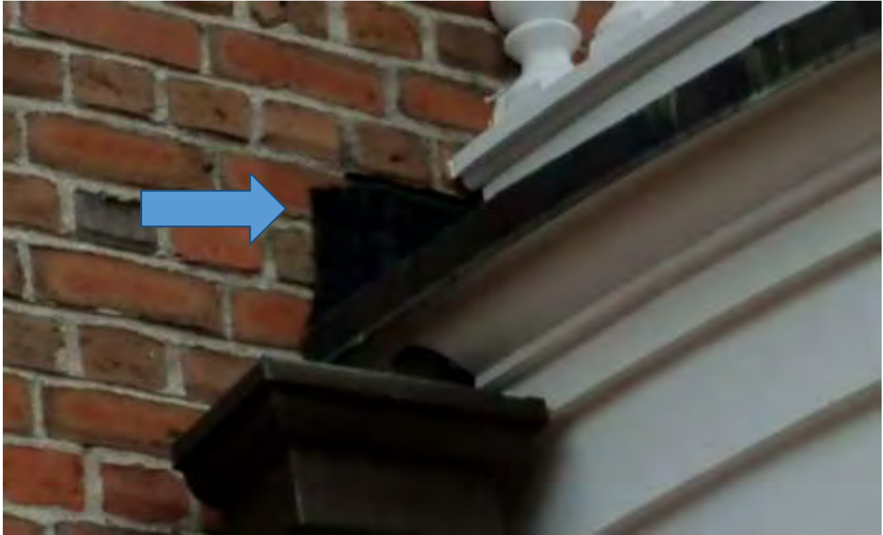
MEMBRANE ROOF AT EAST ENTRY NOT PROPERLY TERMINATED (ARROW)
