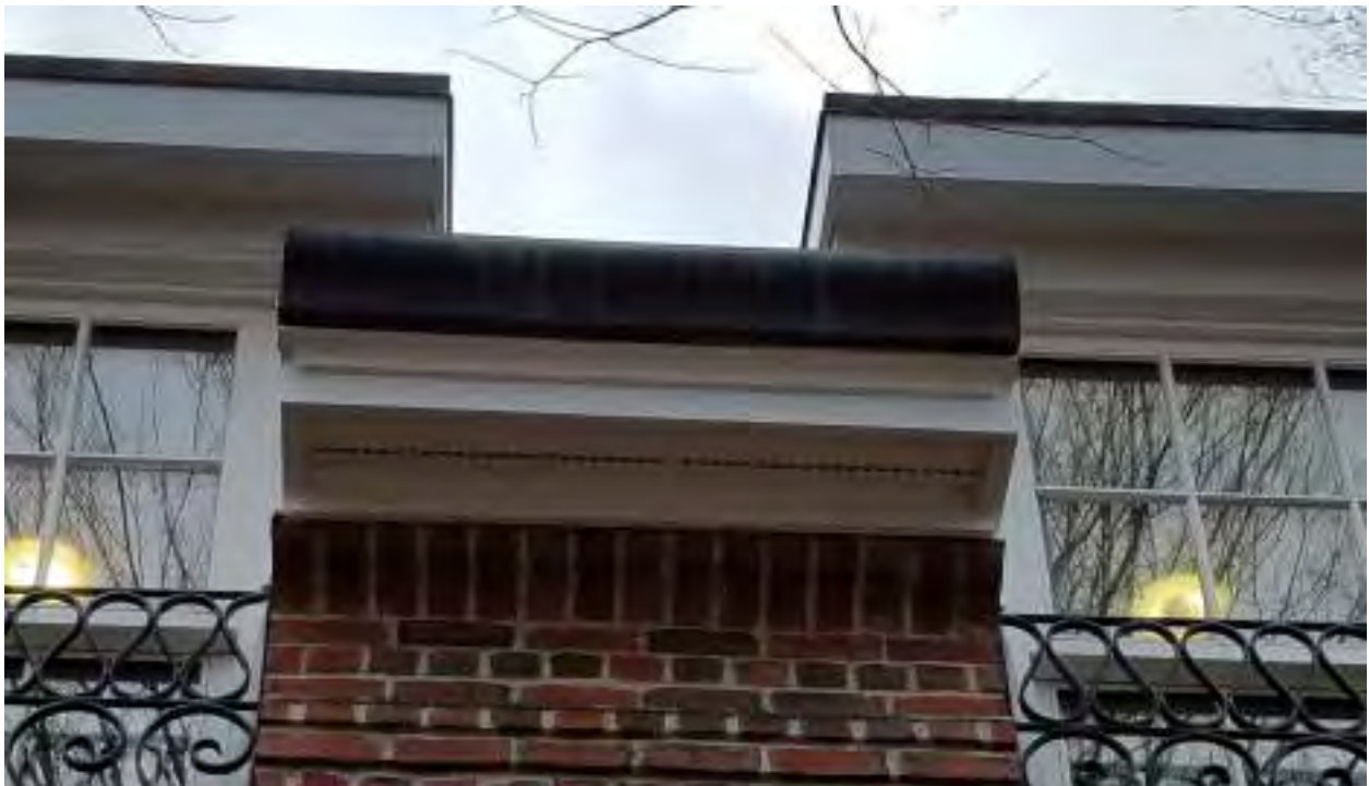
GUTTER WITH NO APPARENT DOWNSPOUT (EAST ELEVATION)
