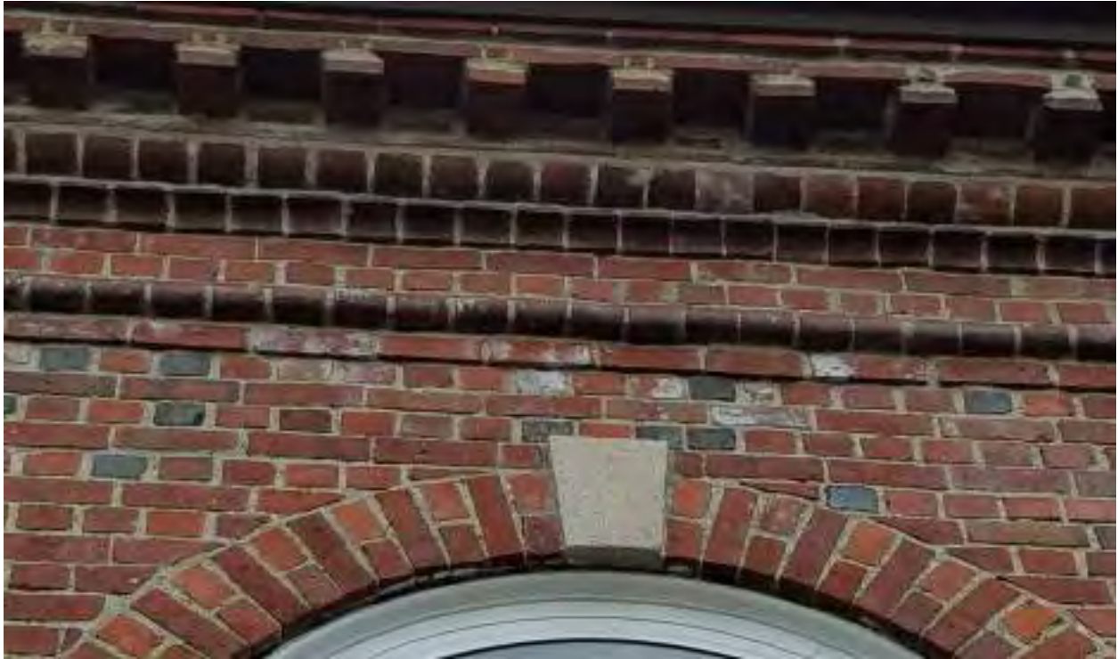
SHOWING POSSIBLE INFILTRATION ON WEST ELEVATION CAUSING EFFLORESCENCE
