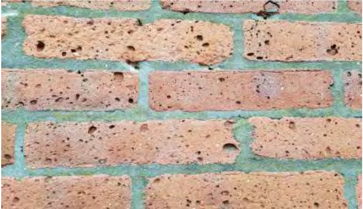
EXAMPLE OF EXTREMELY POROUS CONDITION OF EXISTING BRICK – SUSCEPTIBLE TO MOISTURE INFILTRATION AND FREEZE/THAW DAMAGE – ALSO ORGANIC GROWTH ON MORTAR
