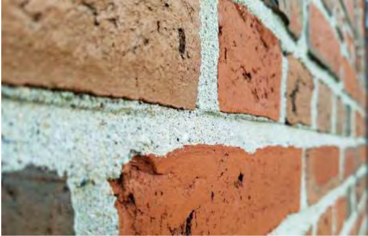
CLOSE-UP OF "WEATHERED-STYLE" BRICK JOINT IN NEW ADDITION
