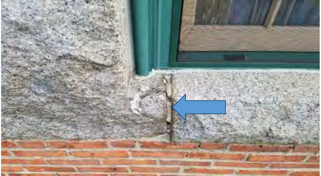
SHOWING REPOINTING NEEDED AT GRANITE SILLS
