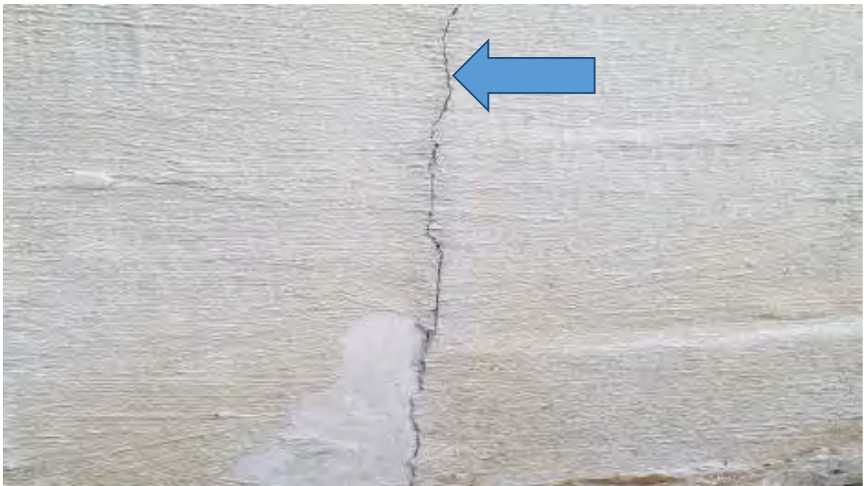
STUCCO PARGING IN EXTERIOR STAIRWELL NEEDING REPAIR and CONTROL JOINT
