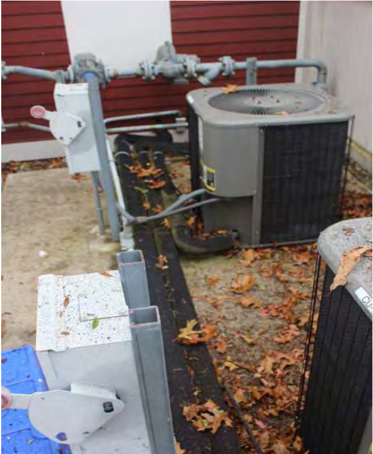
Ground mounted condensing units
