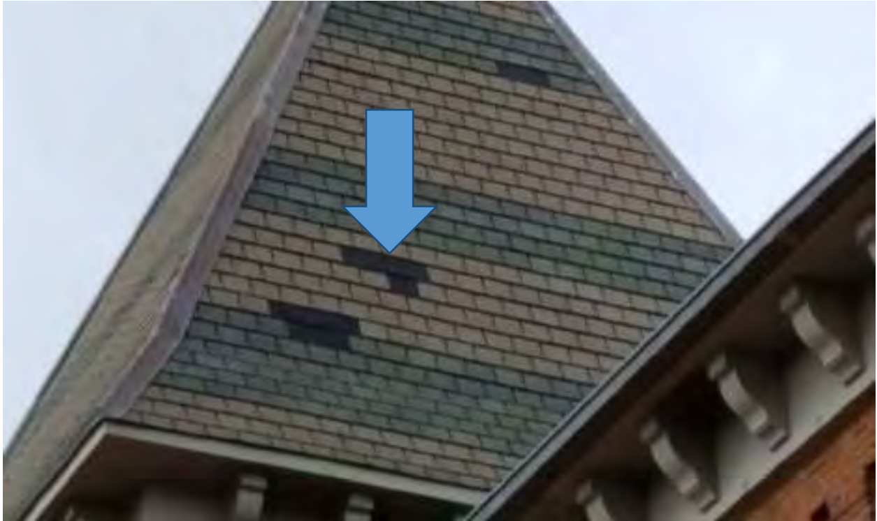
MISSING SHINGLES ON TOWER ELEMENTS
