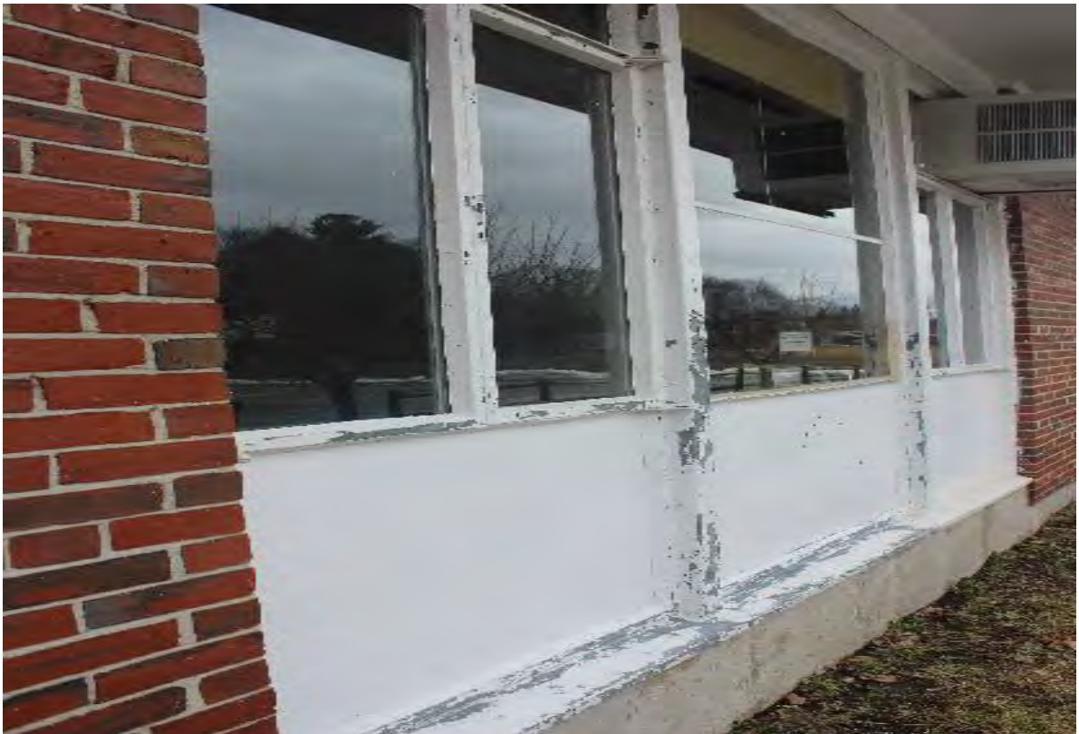
Typical 1960 window single pane, non insulated panel, failing caulking and paint
