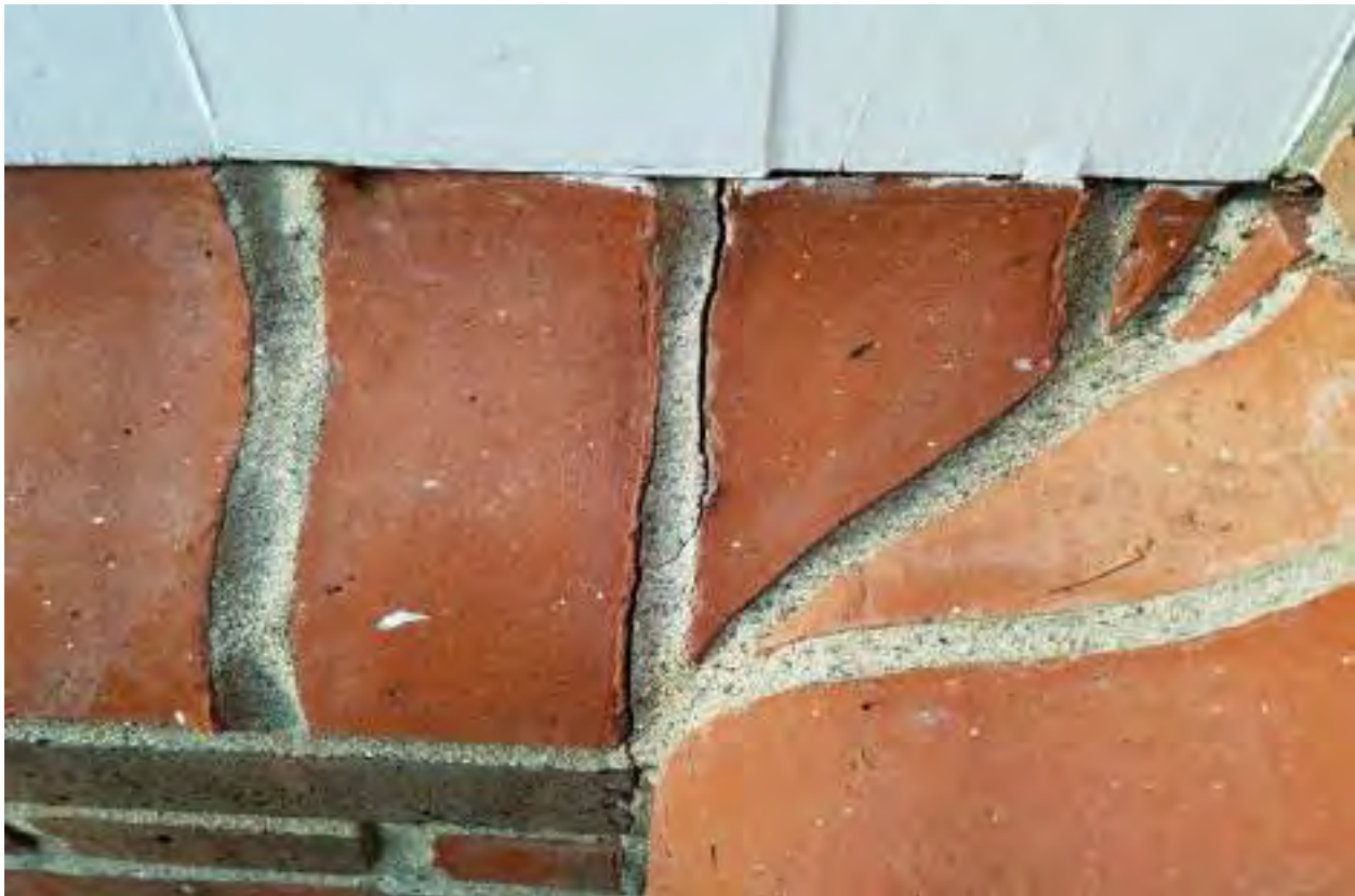
TYPICAL OPEN JOINTS IN WATER TABLE BRICK JOINTS NEEDING REPOINTING
