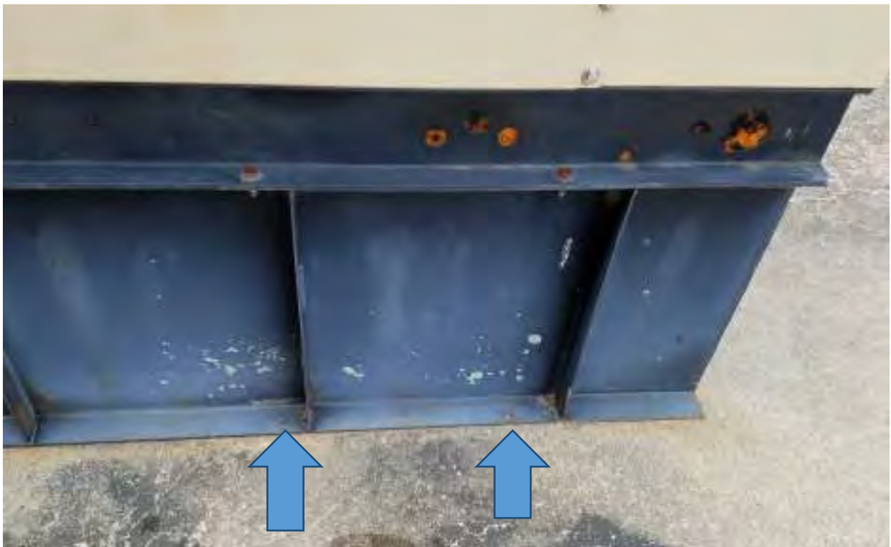
GENERATOR UNSECURED TO CONCRETE PAD
