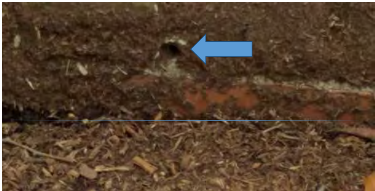
SHOWING TYPICAL CLOGGED WEEP HOLES DUE TO MULCH
