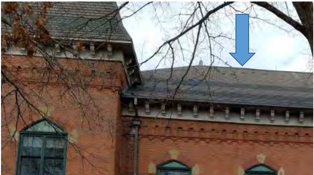
FRONT SHINGLED ROOF SHOWING MISSING SHINGLES
