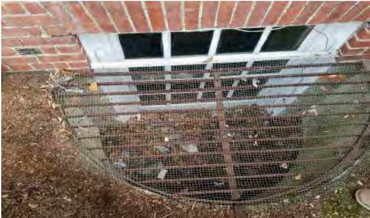
SHOWING TYPICAL AREA WELL NEEDING DEBRIS REMOVED
