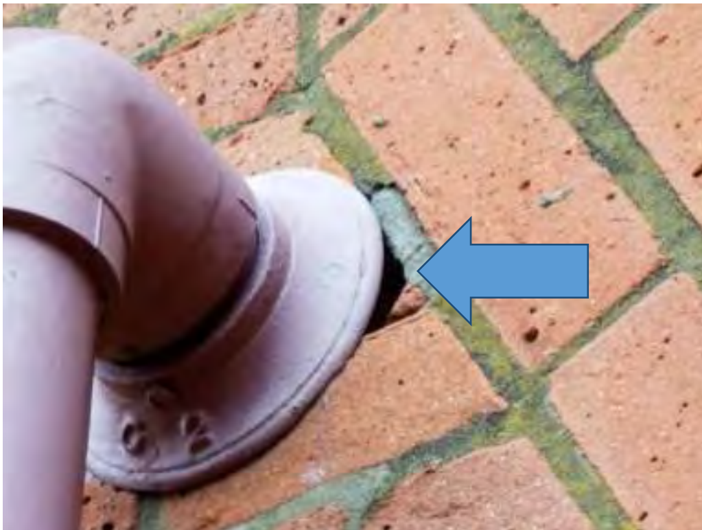
GAPS AROUND SPRINKLER DRAIN NEEDING SEALANTS
