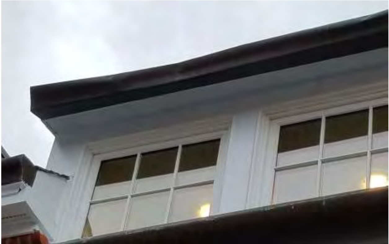
EXAMPLE OF DAMAGED GUTTERS (WEST ELEVATION)
