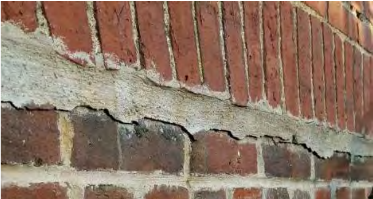
POORLY EXECUTED REPOINTING (WEST ELEVATION)
