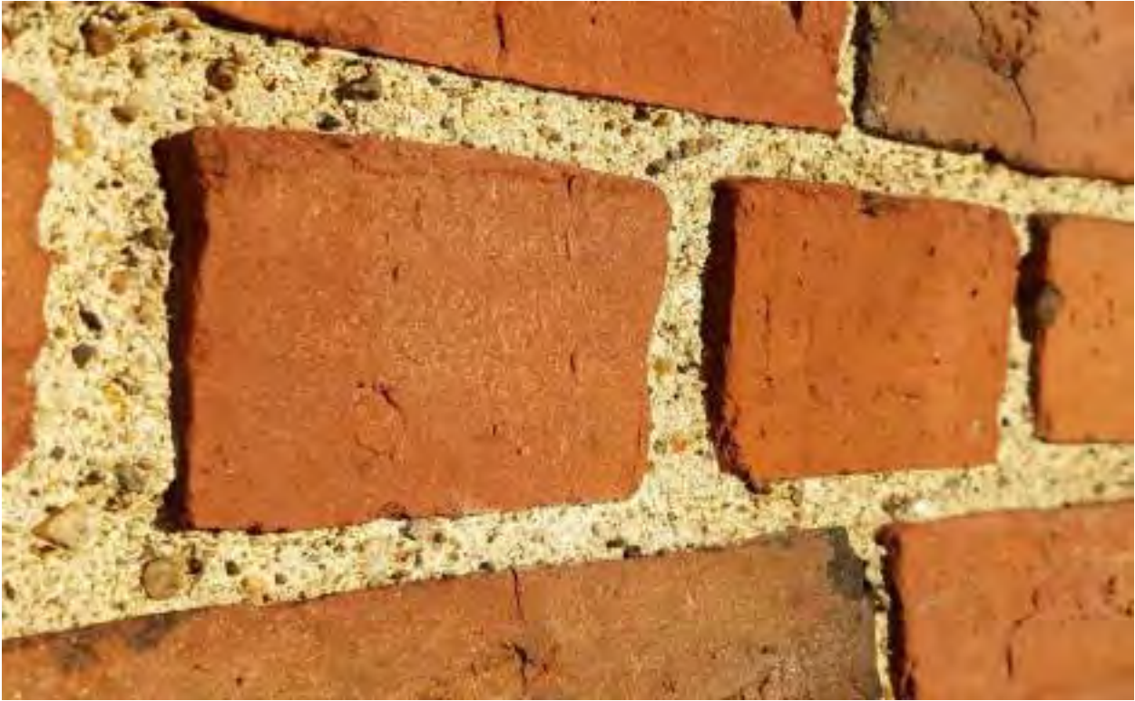
CLOSE-UP OF ORIGINAL MORTAR JOINTS SHOWING COURSE TEXTURE and WIDE SPREAD EFFLOREENCE
