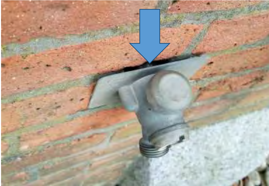
GAPS AROUND EXTERIOR HOSE BIBS NEEDING SEALANTS
