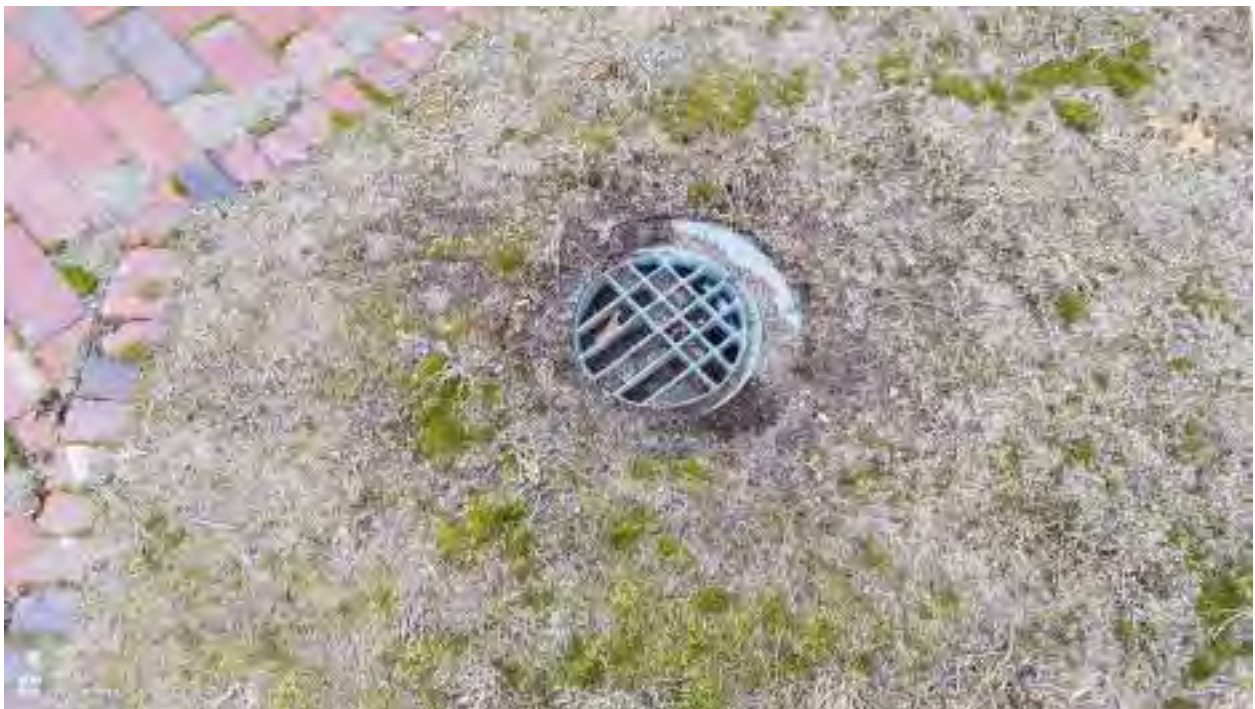
TYPICAL LANDSCAPING LIGHTS FILLED WITH DEBRIS
