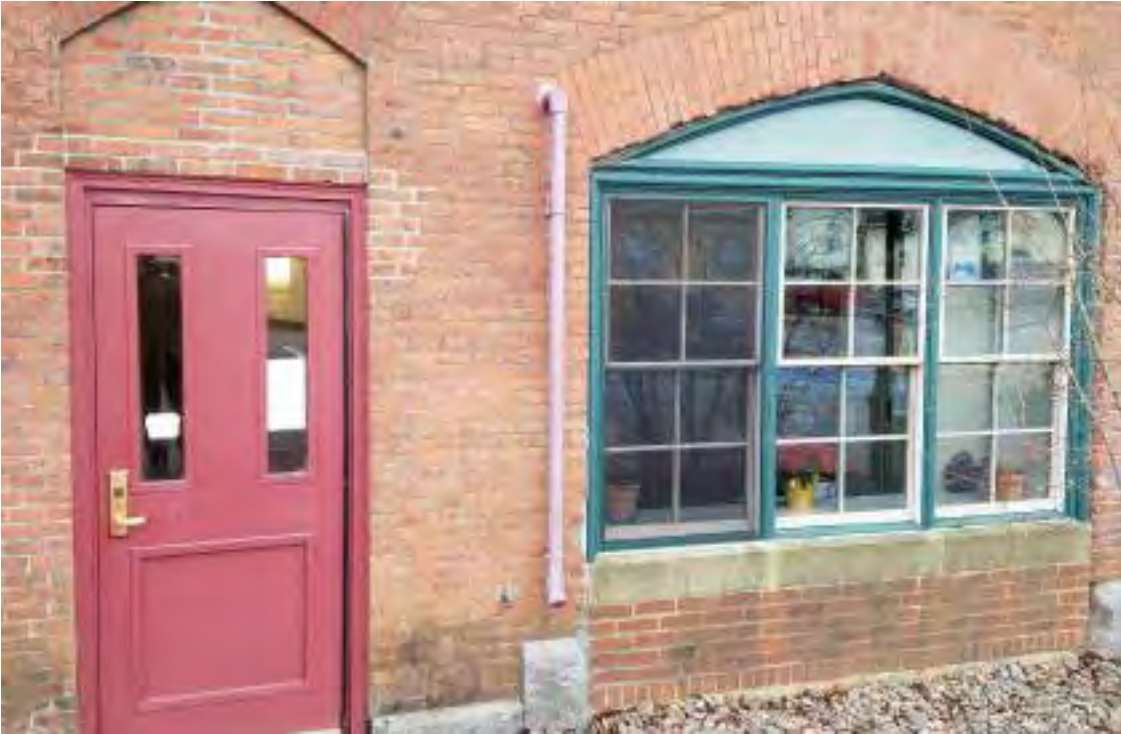
TYPICAL METAL DOORS and WINDOW UNIT (Note missing screens here & elsewhere)
