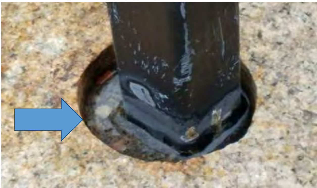
GAPS AROUND GUARDRAIL POSTS COLLECTING WATER & ICE
