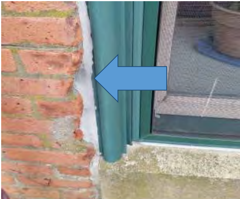
TYPICAL WINDOW UNIT SHOWING PERIMETER CAULKING
