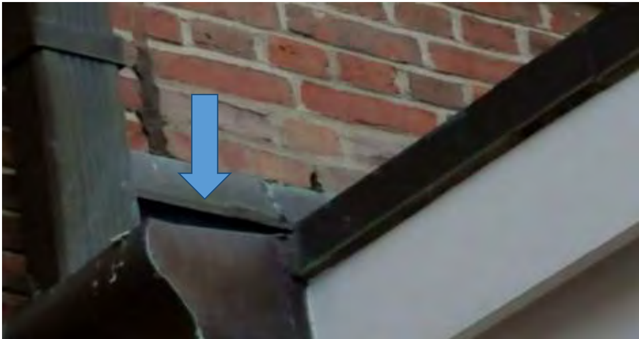
UPLIFTED COUNTER FLASHING (ARROW) ON REAR ELEVATION
