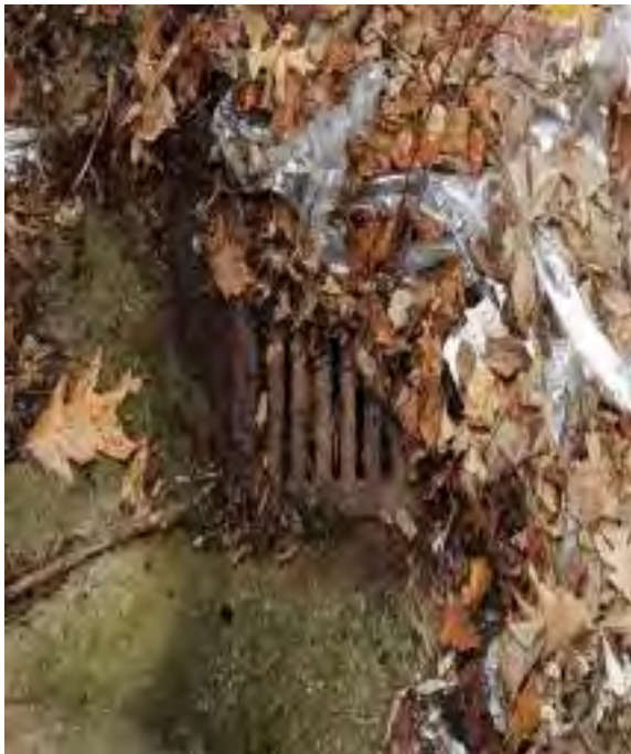
CLOGGED DRAIN IN EXTERIOR STAIRWELL
