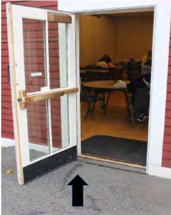
Poor drainage has led to frost heaving and door failure to open. All locations
