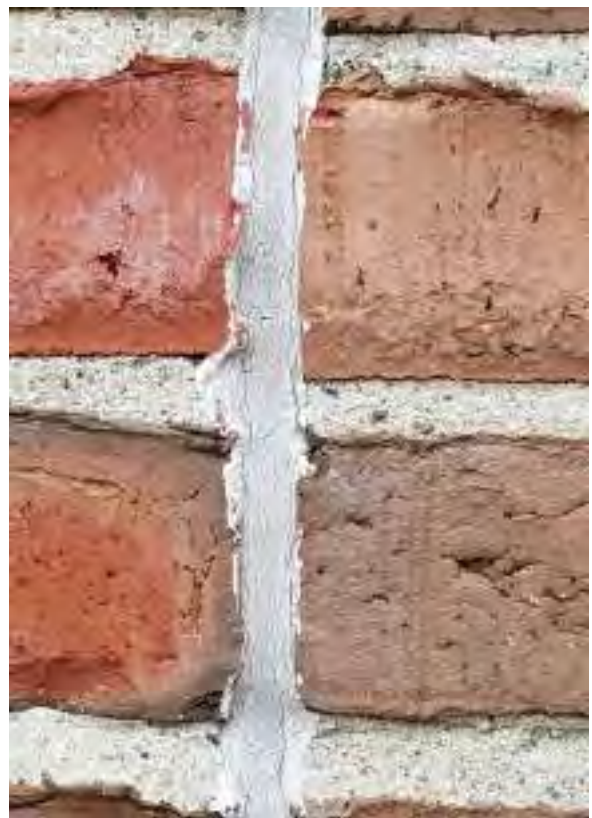
MASONRY CONTROL JOINT TO BE REDONE
