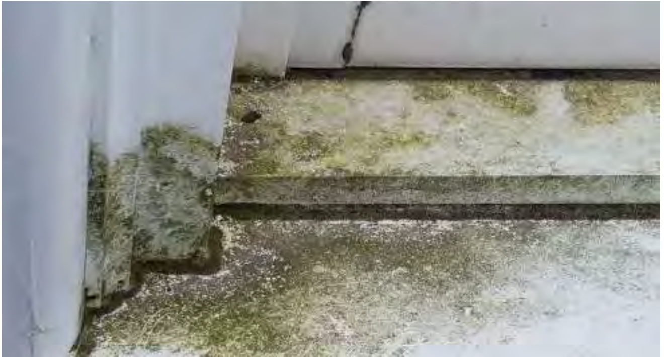
MILDEW & DETERIORATED SEALANTS SHOWN AT EASTERLY WINDOW UNIT WITH POSSIBLE REVERSE SLOPING SILL
