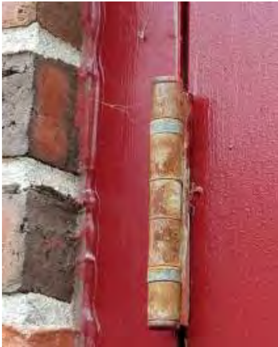
RUSTED DOOR HINGES (SOUTH ELEVATION)
