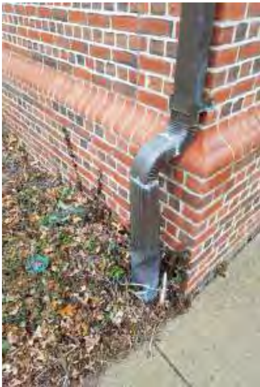
DAMAGED DOWNSPOUT
