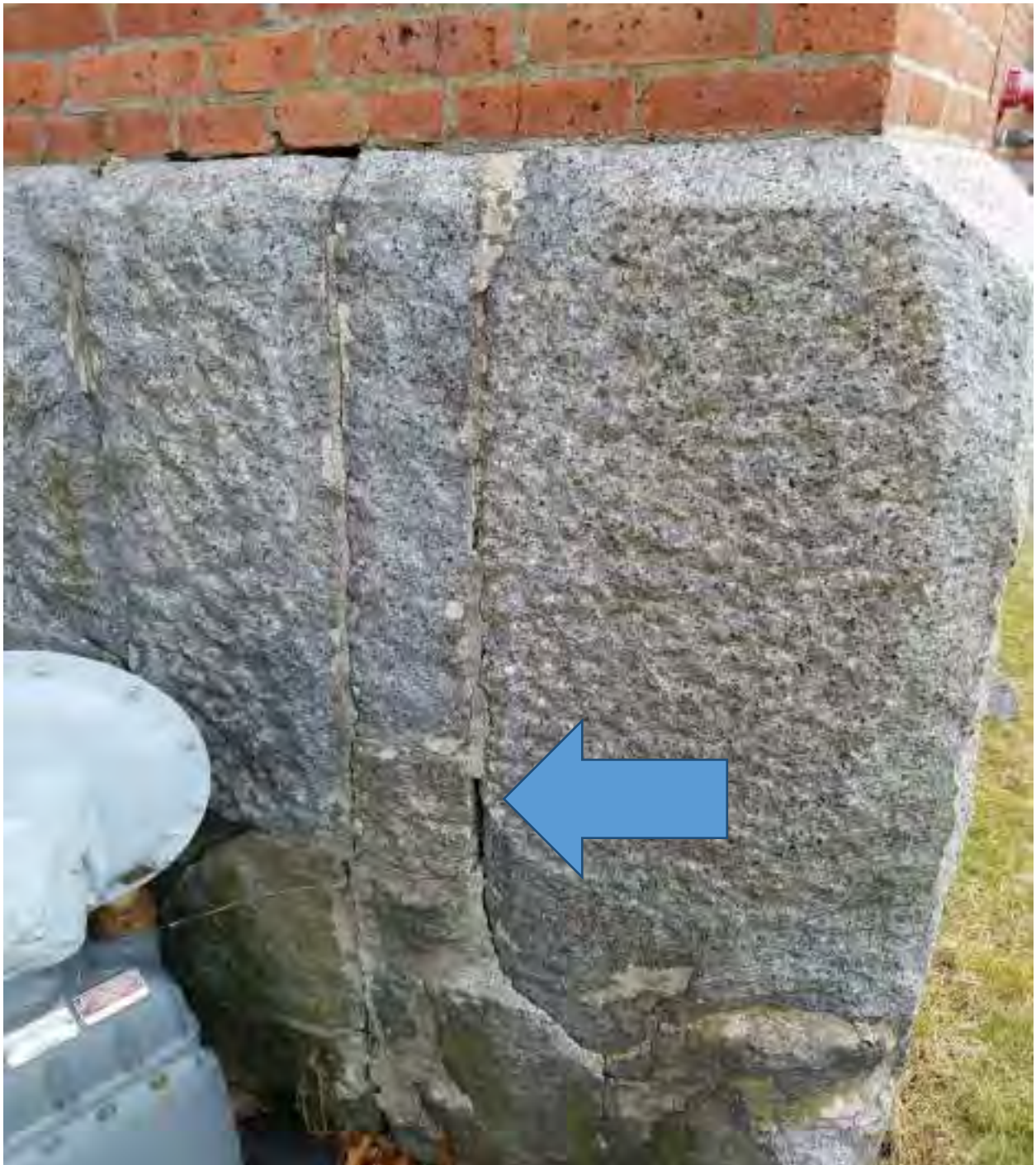
TYPICAL CRACKS IN GRANITE FOUNDATION CAP STONES
