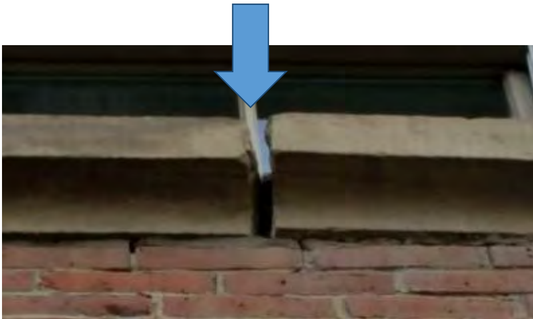
COMPLETELY DETERIORATED JOINTS IN LIMESTONE SILLS and SOURCE OF WATER INFILTRATION
