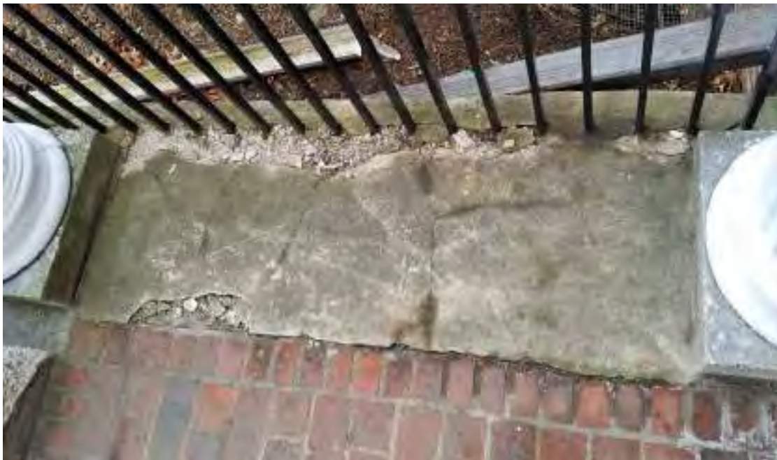
DETERIORATED EDGES OF ORIGINAL ENTRY PLATFORM (NORTH ELEVATION)
