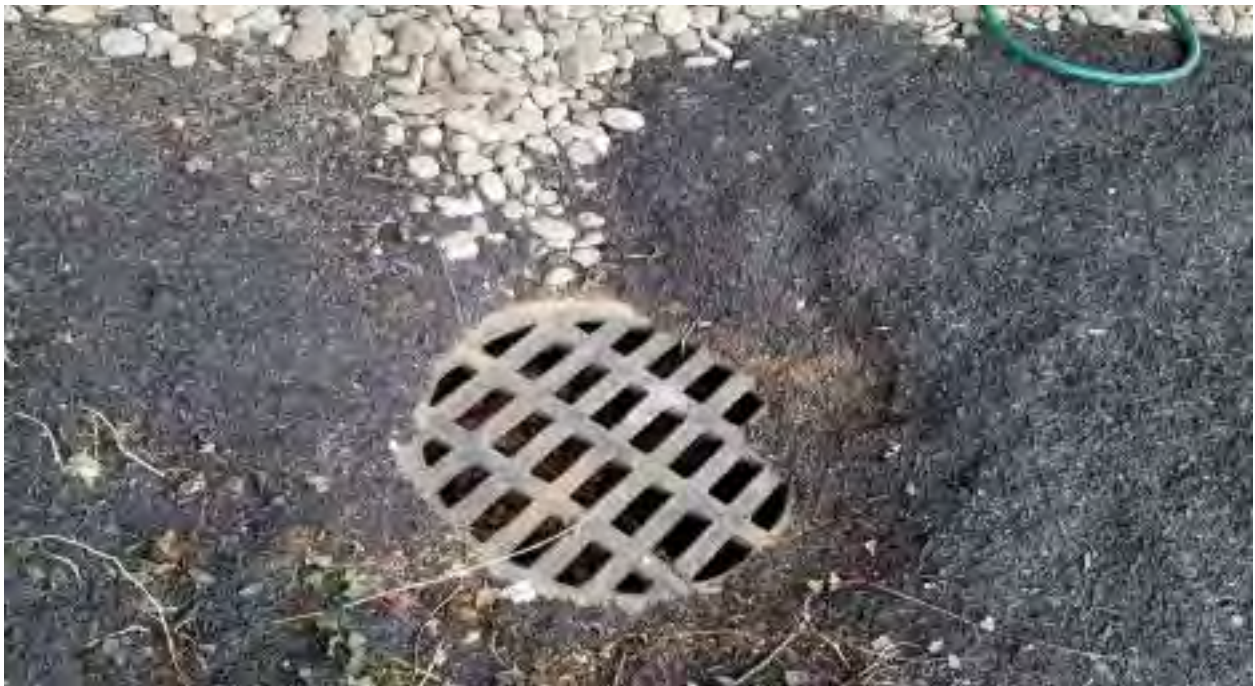
AREA DRAIN AT REAR LANDSCAPING AREA SHOWING MULCH WASHING INTO SUMP
