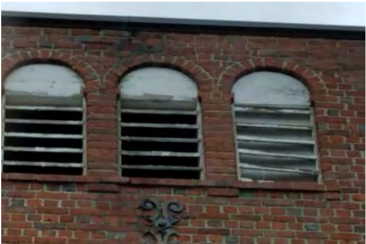
LOUVERS AND CAST IRON BRACKETS NEEDING PAINTING (REAR ELEVATION)
