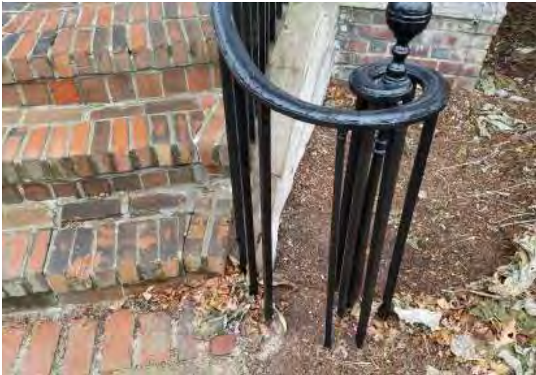
DETERIORATED BRICK STEPS AT ORIGINAL ENTRANCE STEPS (NORTH ELEVATION)
