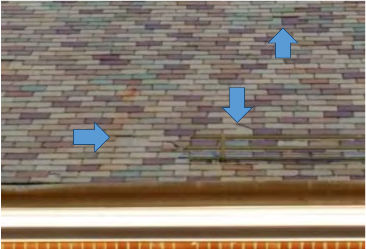
WEST-FACING SLATE ROOF SHOWING MISSING SLATES
