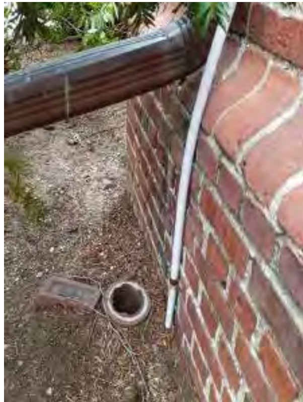
UNCONNECTED DOWNSPOUT
