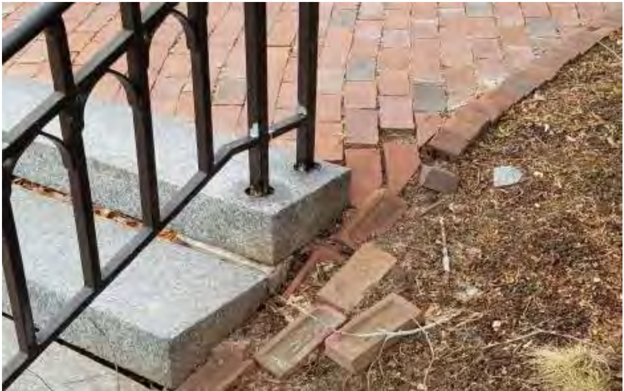
POOR CONDITION OF GRANITE STEPS AT FRONT ENTRANCE WALKWAY SHOWING GAPS IN GRANITE AND LOOSE BRICKS
