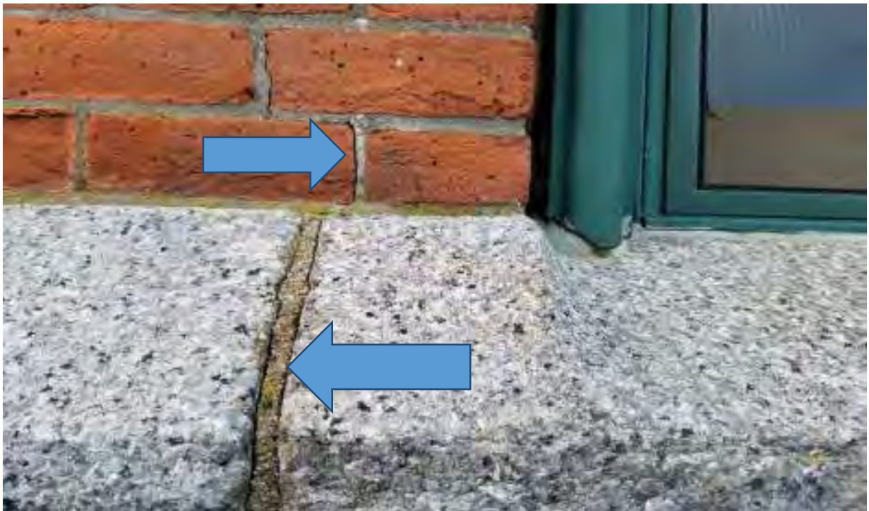
EXAMPLE OF OPEN JOINTS IN GRANITE SILLS and NOTE CRACKS IN MORTAR AT BRICK
