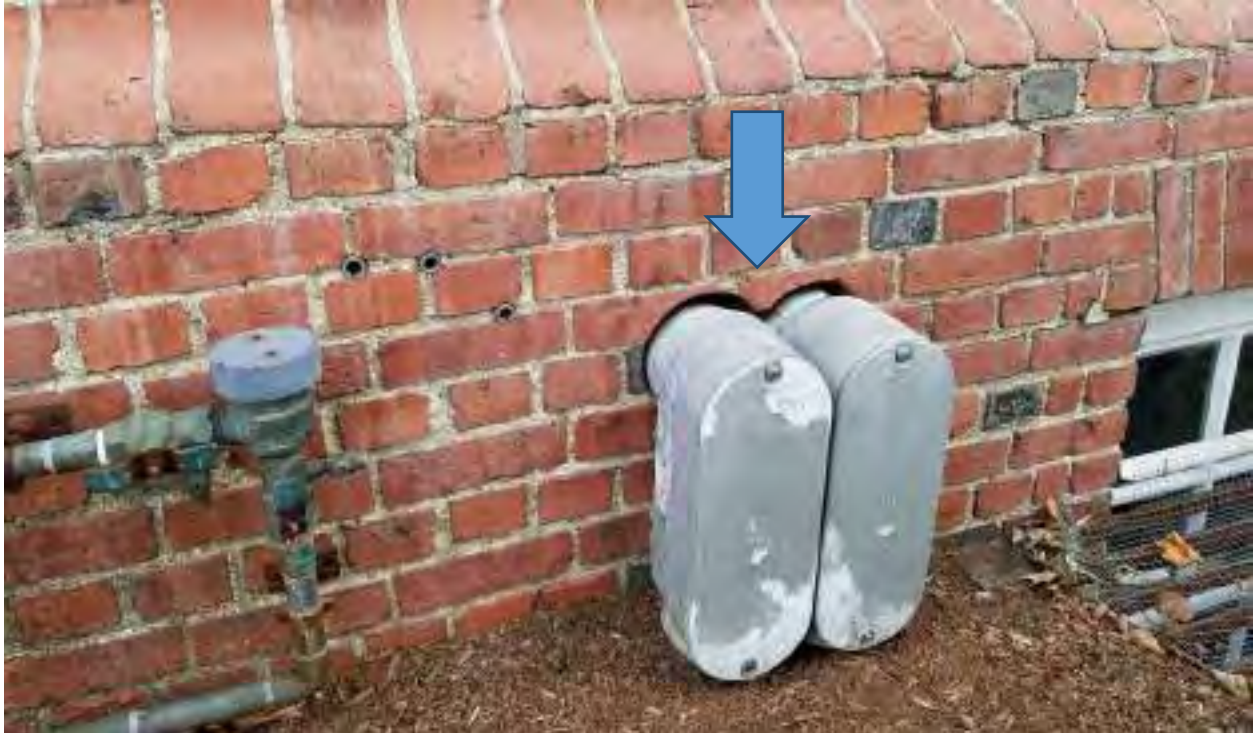
PROVIDE SEALANTS AROUND ELECTRICAL SERVICE PENETRATIONS (WEST)
