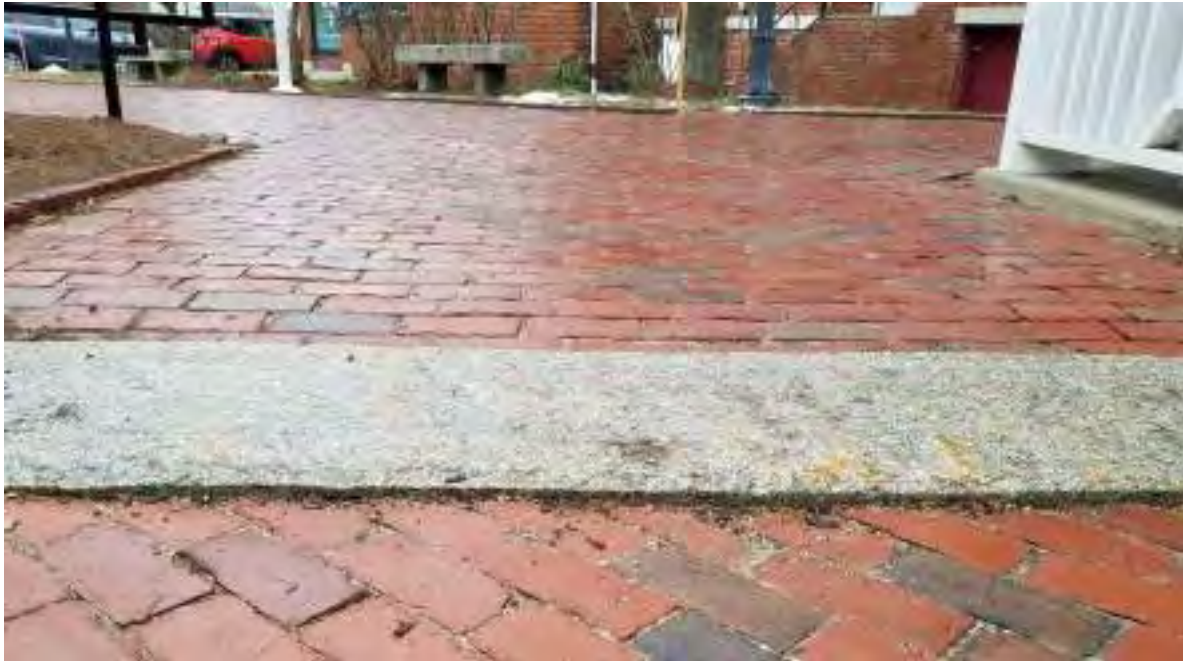
GRANITE ACCENT STRIP LIFTED CAUSING HAZARD ALONG ACCESSIBLE ROUTE
