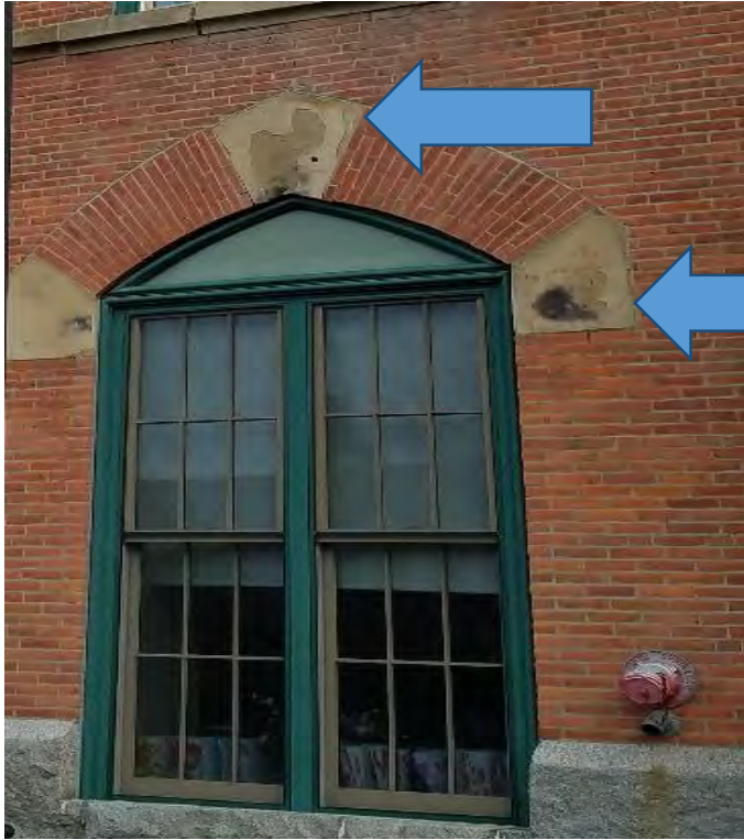
TYPICAL DETERIORATED LIMESTONE KEYS
