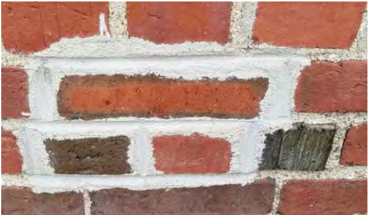
SHOWING POORLY EXECUTED REPOINTING DONE PREVIOUSLY (WEST ELEVATION)
