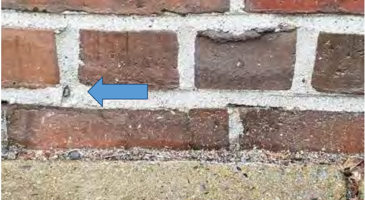
WEEP HOLES BLOCKED (REAR) ALONG SIDEWALK
