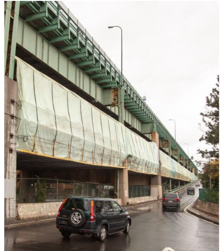
Tobin Bridge dust and pollutant containment system in Chelsea, MA
