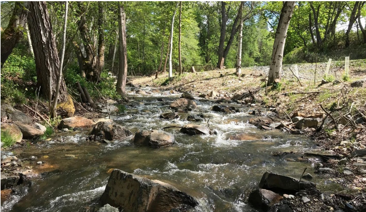
Figure 6. Roughened channel after dam removal on Wagner Creek, Oregon (Rogue River Watershed Council website)
