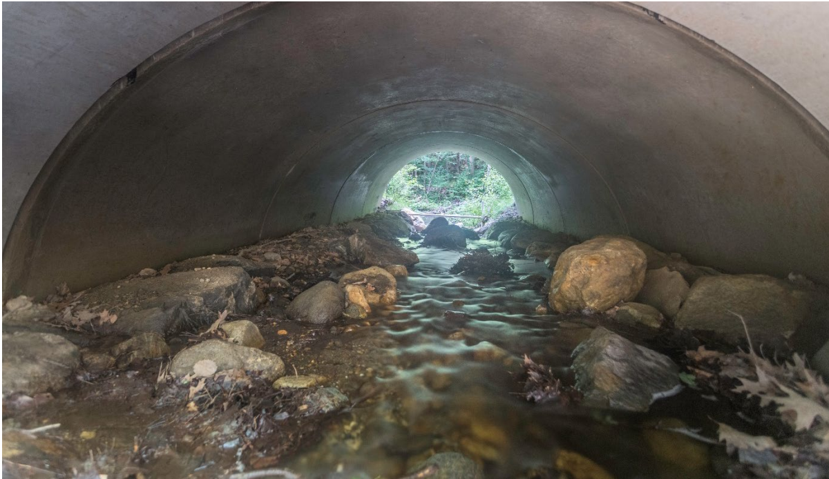
Figure 9. Banks within the structure provide bank-edge habitat where water velocities are typically lower than in the main part of the channel. In this photo, banks also contribute to the formation of a low-flow channel that provides sufficient water depth for aquatic organism passage at low flows.
