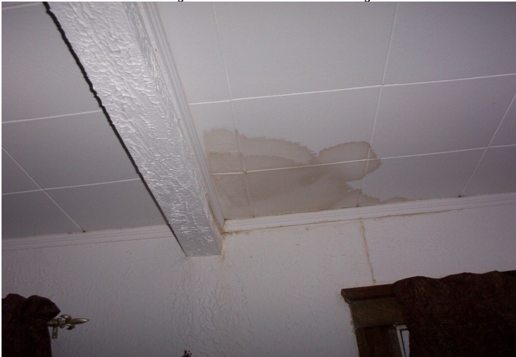
Family 705, 319 Washington Street Living Room Has Water Stains on Ceiling
