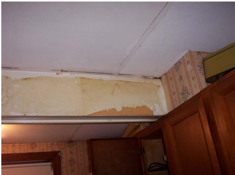
Family 705, 76 Beech Street Water-Stained Ceiling, Peeling Wallpaper in Kitchen
