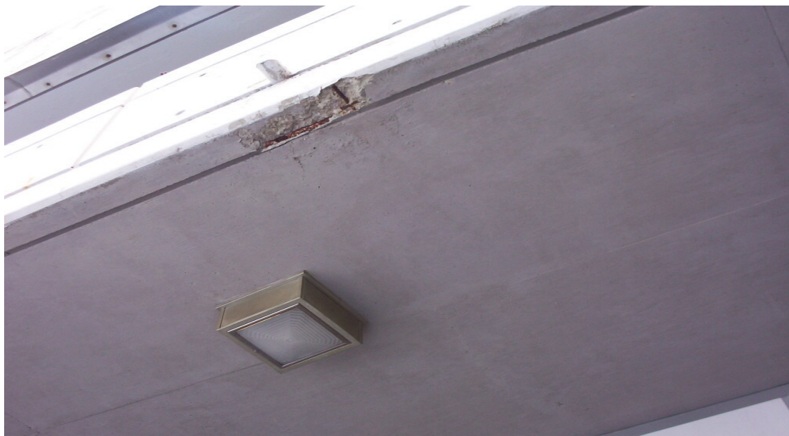
Elderly Development 667, Steele Building Common Areas, Exterior Concrete Breaking Away
