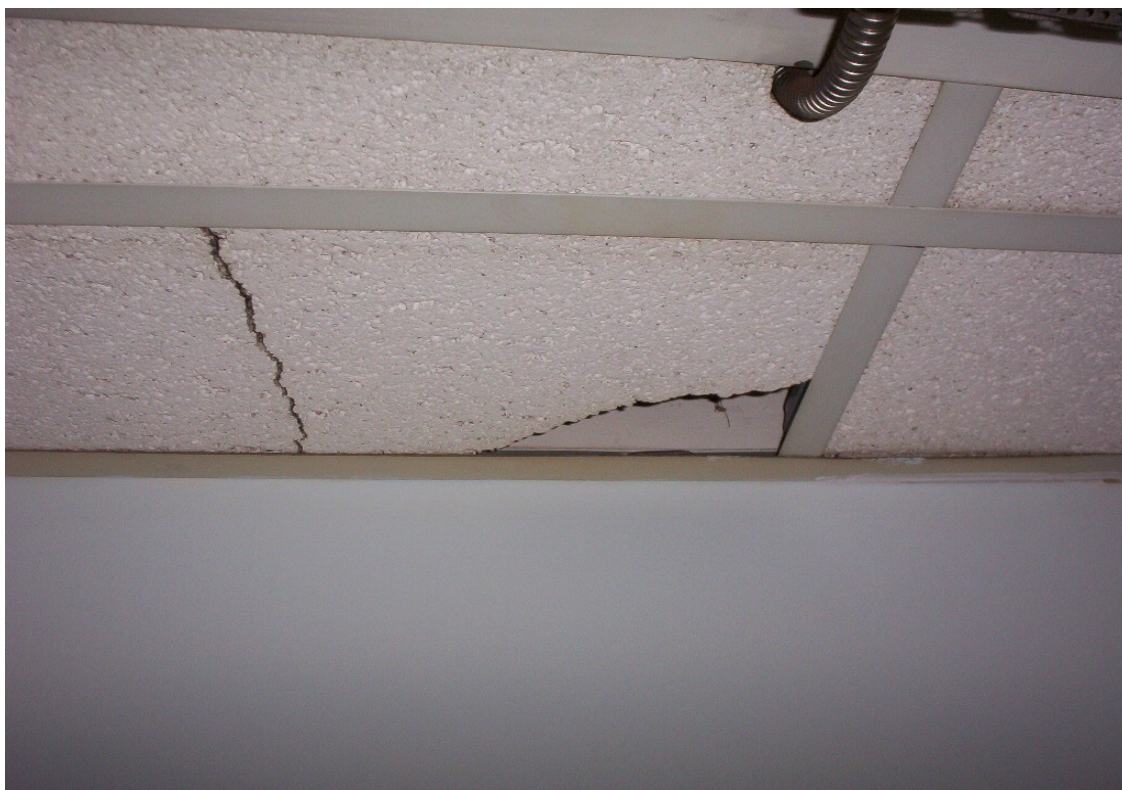
Elderly Development 667, McCarthy Building, Common Area, 7 th Floor Broken Ceiling Tiles
