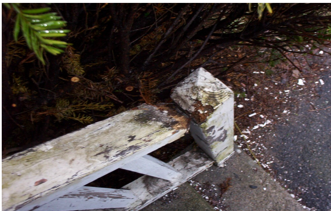
Family 705, 489 Lebanon Street Severely Deteriorated Railing
