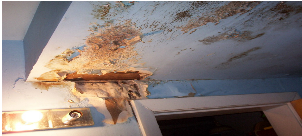
Family 705, 487 Lebanon Street Peeling Paint and Mold on Ceiling in Bathroom
