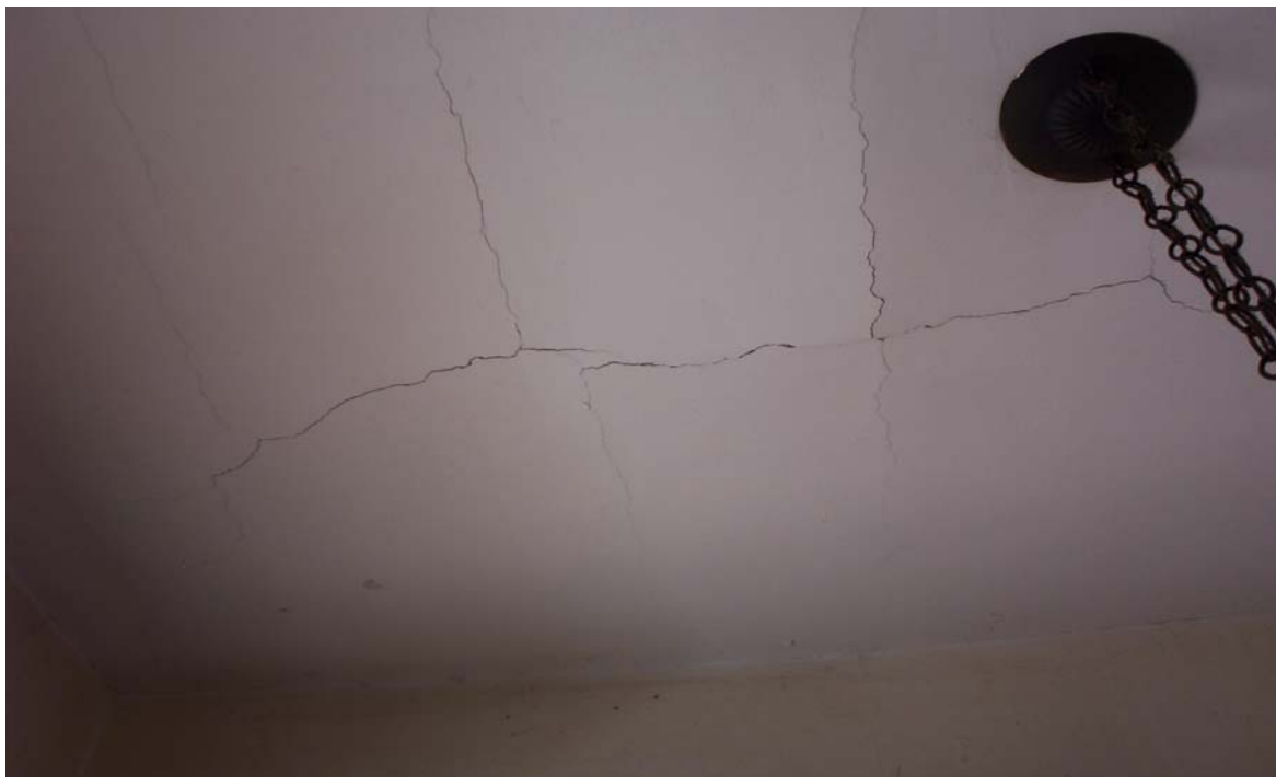
Family 705, 76 Beech Street Common Area Stairwell Has Cracked Ceiling
