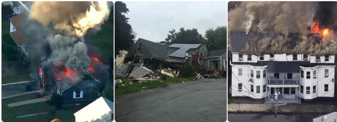
Figure 1: Structures Burn or Explode As a Result of the Natural Gas Over-pressurization.
