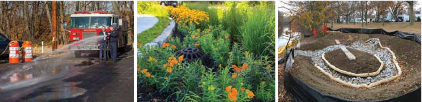
Alongside infiltration trenches, Arlington has employed other small-scale stormwater control systems, including (left to right) porous pavement, rain gardens, and updated outfalls
