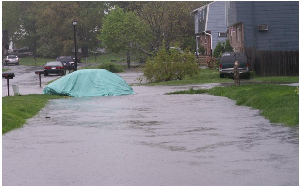
City of Methuen – Bloody Brook Culvert Improvements Bloody Brook at Bicknell Avenue Looking North
