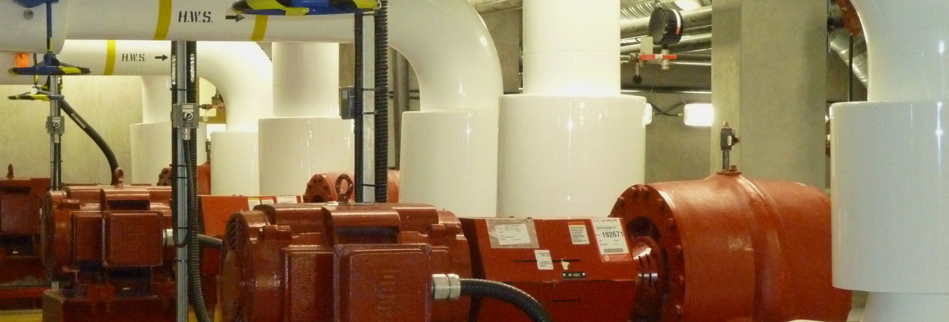
Sample Hot Water Pumps
