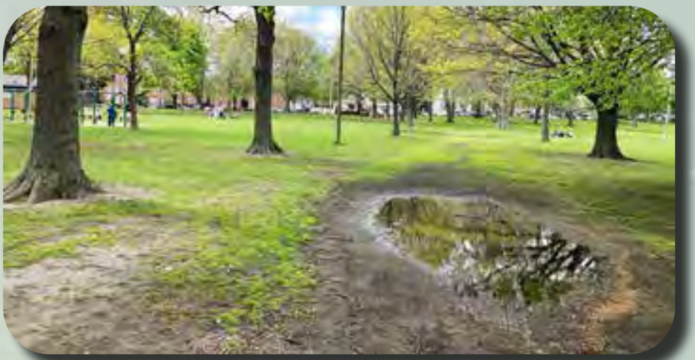
DRAINAGE AND GRADING ISSUES AT ENTRY PATH
