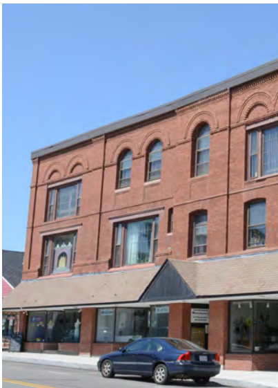
Figure D-52. This is one of several multi-tenanted buildings in Downtown Attleboro that uses an overhang in lieu of awnings. While an overhang offers shade and weather protection, the individual storefronts are less visible.
