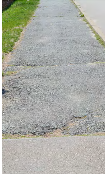
Figure D-5. Sidewalk to public parking area.
