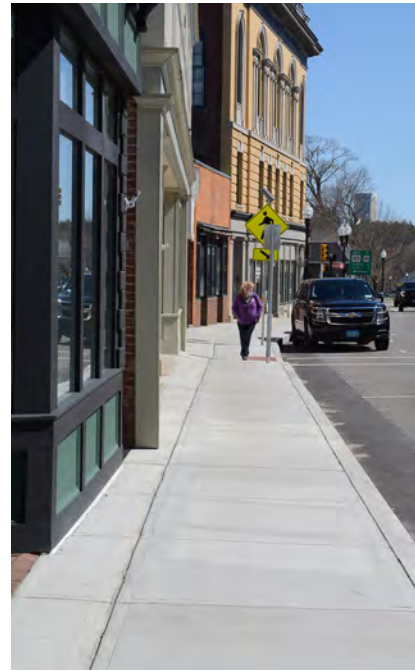
Figure D-3. New Center Street sidewalk.
