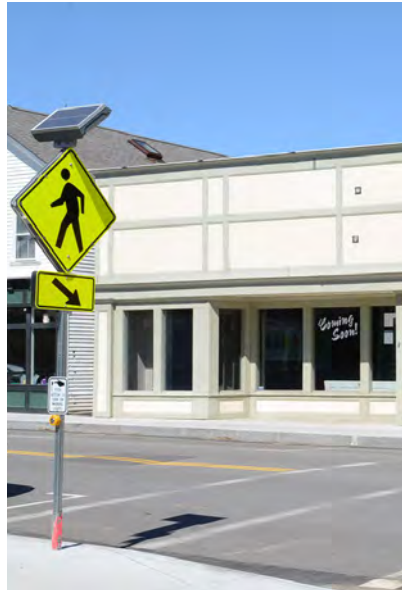
Figure 34 and 35. The pavement markings need to be repainted on these crosswalks on Center Street. On the right is a new pedestrian crossing sign to increase visibility to motorists with a solar-powered crossing light.
