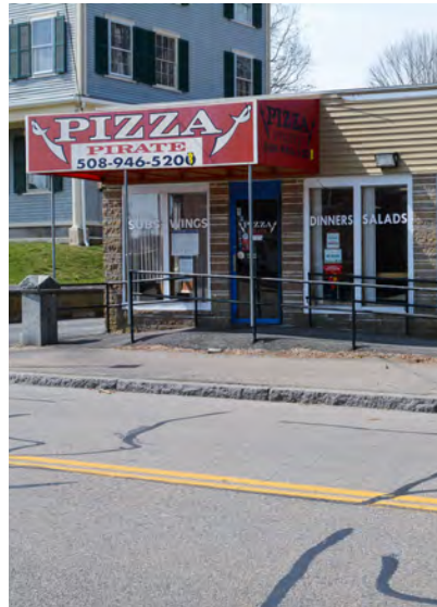
Figure D-51. The Pizza Pirate uses an awning primarily for advertising and an overhang providing some weather protection at the doorway.
