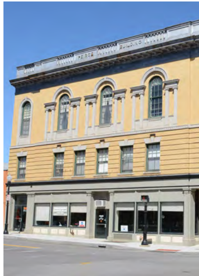
Figure 54. This building has maintained and restored its historic brick façade creating a presence in Downtown Middleborough.
