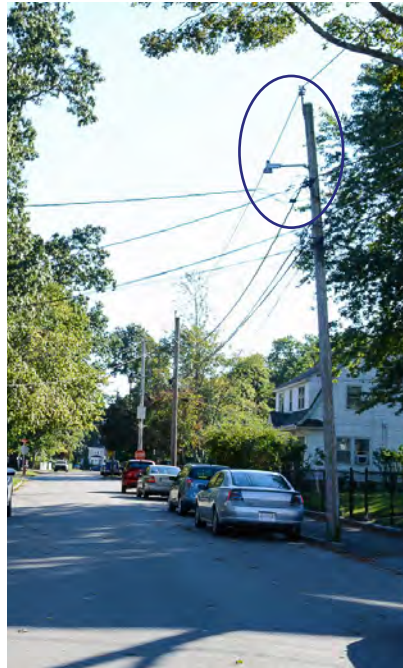
Figure 21. Streetlight on Pearl Street.
