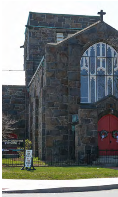
Figure D-2. New Center Street sidewalk.
