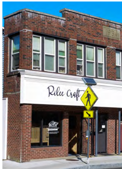
Figures D-49. Rilee Craft sports a clean easy-to-read sign within the sign band of the façade complemented with window graphics.
