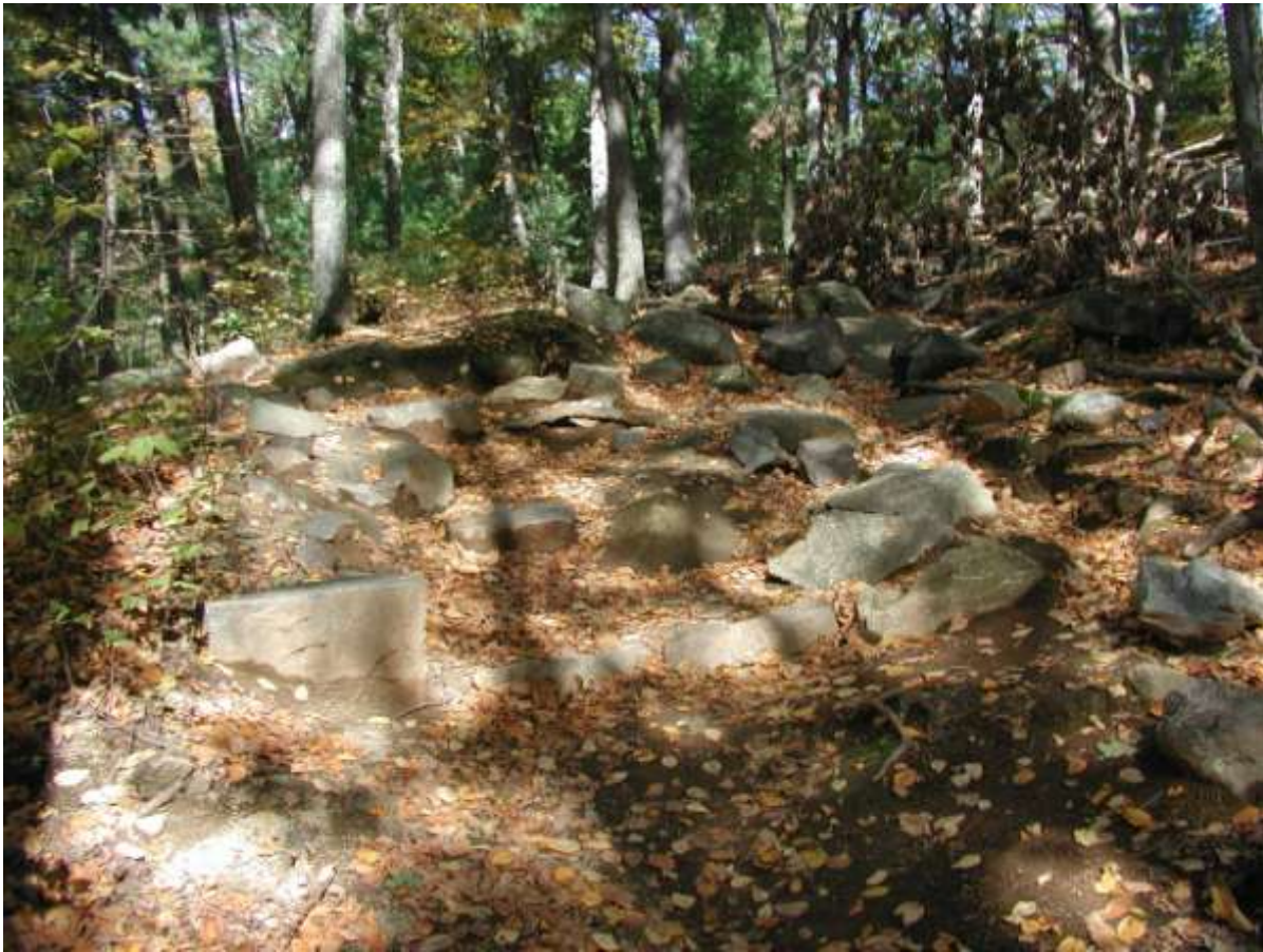
(Stone steps and erosion control structures on the Skyline Trail. Photo by Paul Jahnige )
