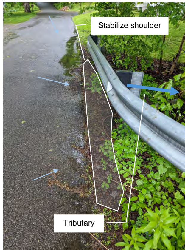
Photo 1-2: Erosion at the culvert crossing of Hatfield Street
