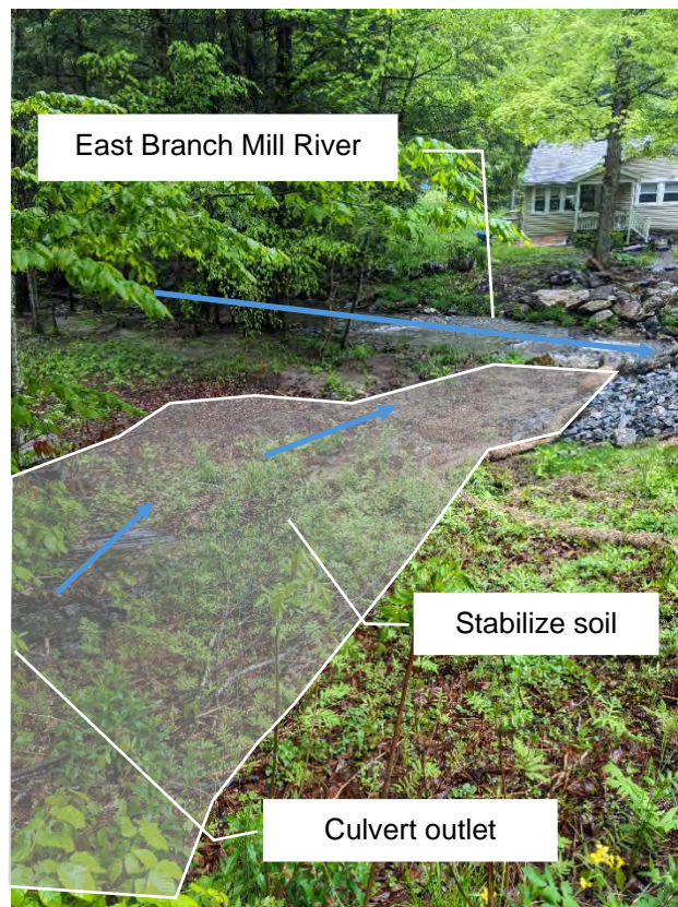
Photo 7-2: Outlet of culvert along Ashfield Road
