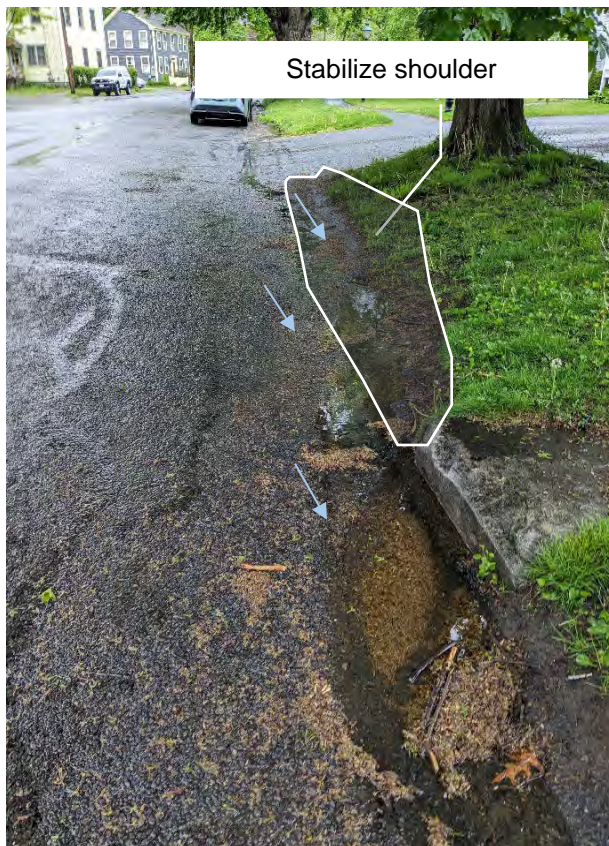
Photo 4-1: Channelization and erosion along the northern shoulder
