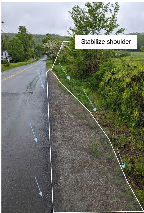
Photo 10-1: Shallow roadside conveyance ditches
