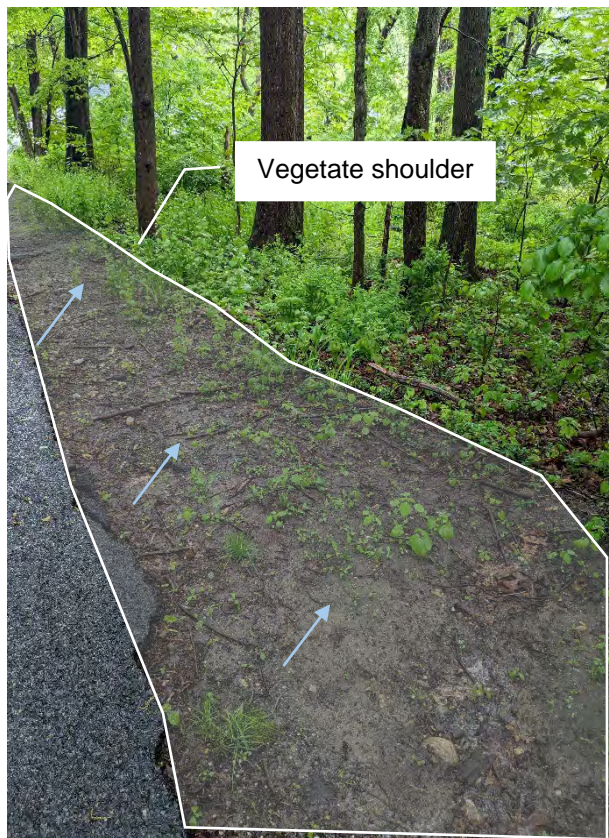
Photo 1-1: Erosion along the shoulder of Hatfield Street
