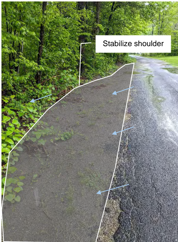
Photo 13B-1: Loose sediment along the eastern shoulder
