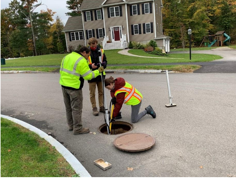
Storm Water Sewer Investigation, Debra Lane, Millis, MA
