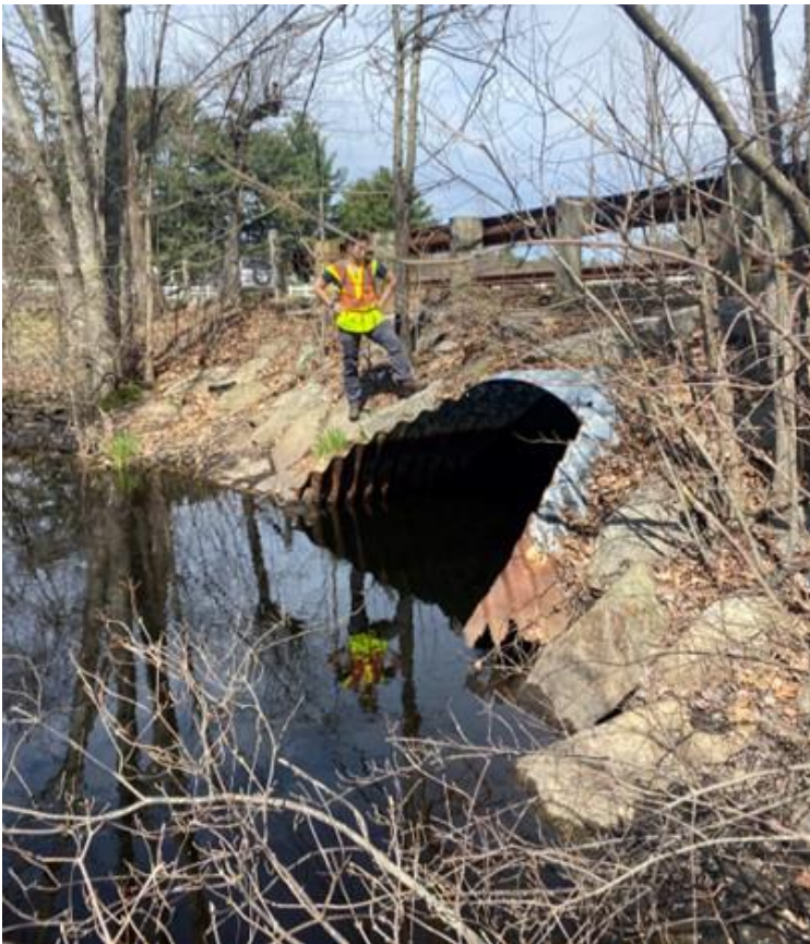
Culvert, Glen Ellen-Orchard St, Millis, MA
