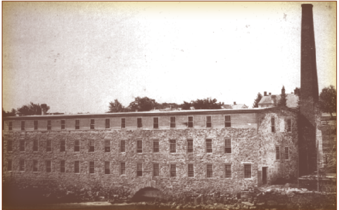
The John Scott Woolen Mill, Millville, demolished.
