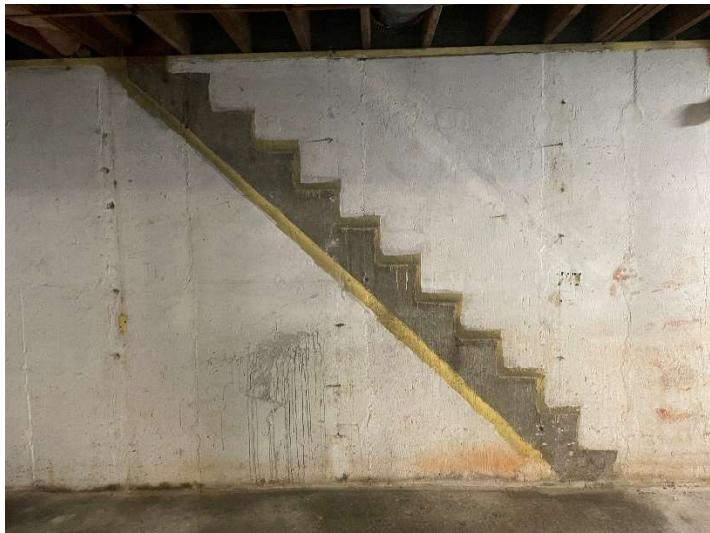
**PHOTO 7:** Existing unfinished ground floor. Build connecting stairs in existing location & finish ground floor level for accessibility and per proposed plans.
