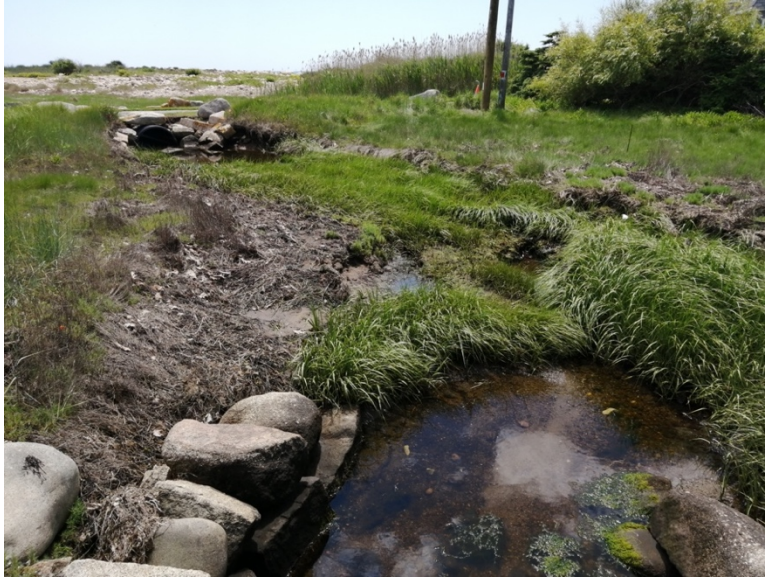
Image F6: Blocked culvert leading to restored marsh
