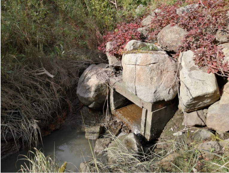
Image F4: Clear and unobstructed culvert at reference marsh
