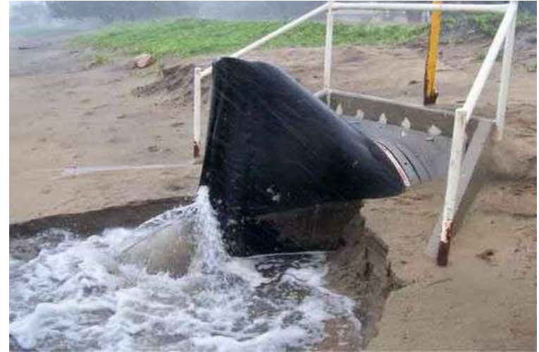
Backflow Prevention Device at Drainage Outfall
