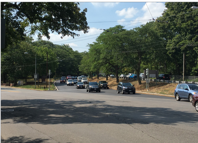
Wide lanes on the southbound approach of Fresh Pond Parkway at Mount Auburn Street create unsafe conditions for drivers as they enter the intersection.
