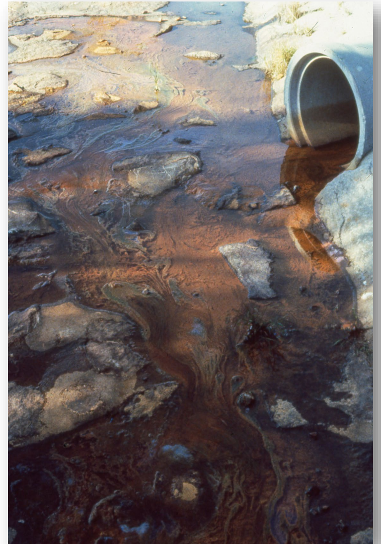
Storm drain outfall Staff Photo, 1985
