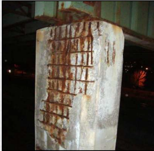
Deteriorating Viaduct
