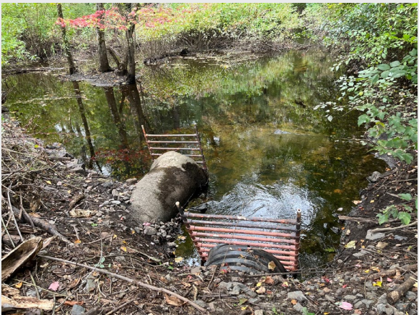
Lower Center Street Stream Crossings
