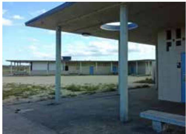
View of Concession/Garage from beach side of Bathhouse. Note the octagonal columns, circular openings in roof, latticework over windows, and concrete bench. (See Appendix K for photo information.)
