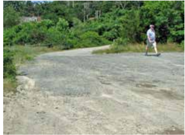
Drivers attempting to avoid potholes in the park's entrance road have driven over vegetation, widening the road (right side of image). (See Appendix K for photo information.)
