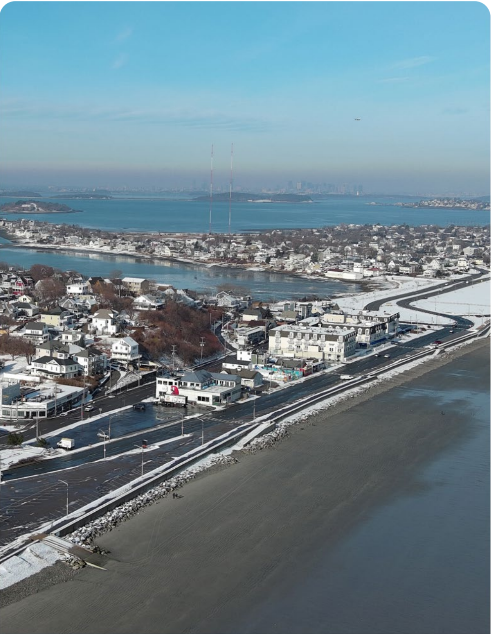
Bird's-Eye View of Project Site, February 2025.
