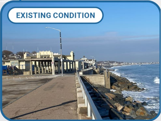
Photo at the parking lot looking West
