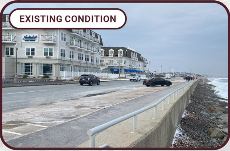
Photo at the existing Hull Shore Drive looking west
