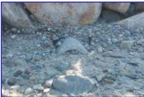
Figure 2-4: Outlet D consisting of an 18" RCP outlet
