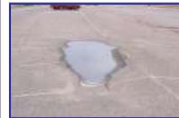
Figure 1-2. Parking Lot 4 with ponding and pavement deterioration to the right.
