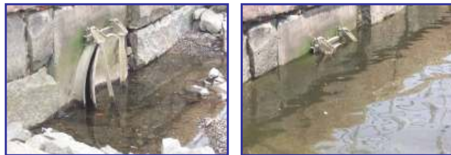
Figure 2-1: Outlet A, consisting of a 48" RCP outlet with tide gate at low tide (left) and high tide (right). The tide gate is locked in a slightly open position.
