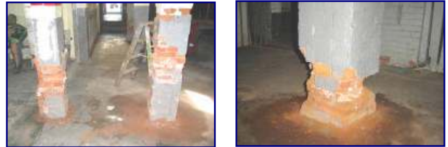
Figure 1-13: Damaged support columns in basement of the Island District Operations Building.
