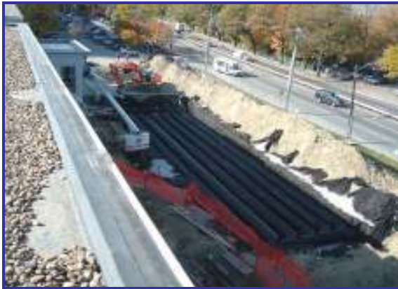
Figure 2-6: Underground detention basin during construction
