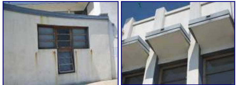
Figure 1-6: Rust and painting requirement on the southern side of the MJM bath House (left). Cracking above the window on the southern side (right).
