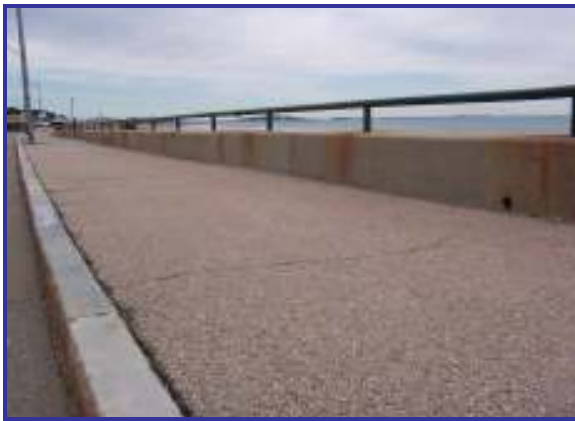
Figure 1-3: Promenade along seawall with weep holes for drainage
