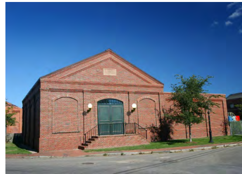
Candle Street Substation. Photo: Design Associates Inc.
