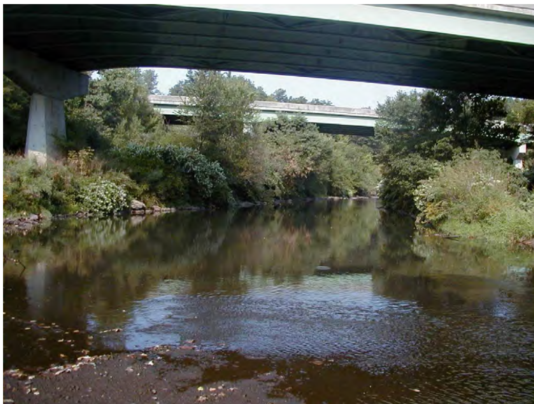
Figure 3 Station NN12 upstream – I-190 Bridges (5/8/2002)
