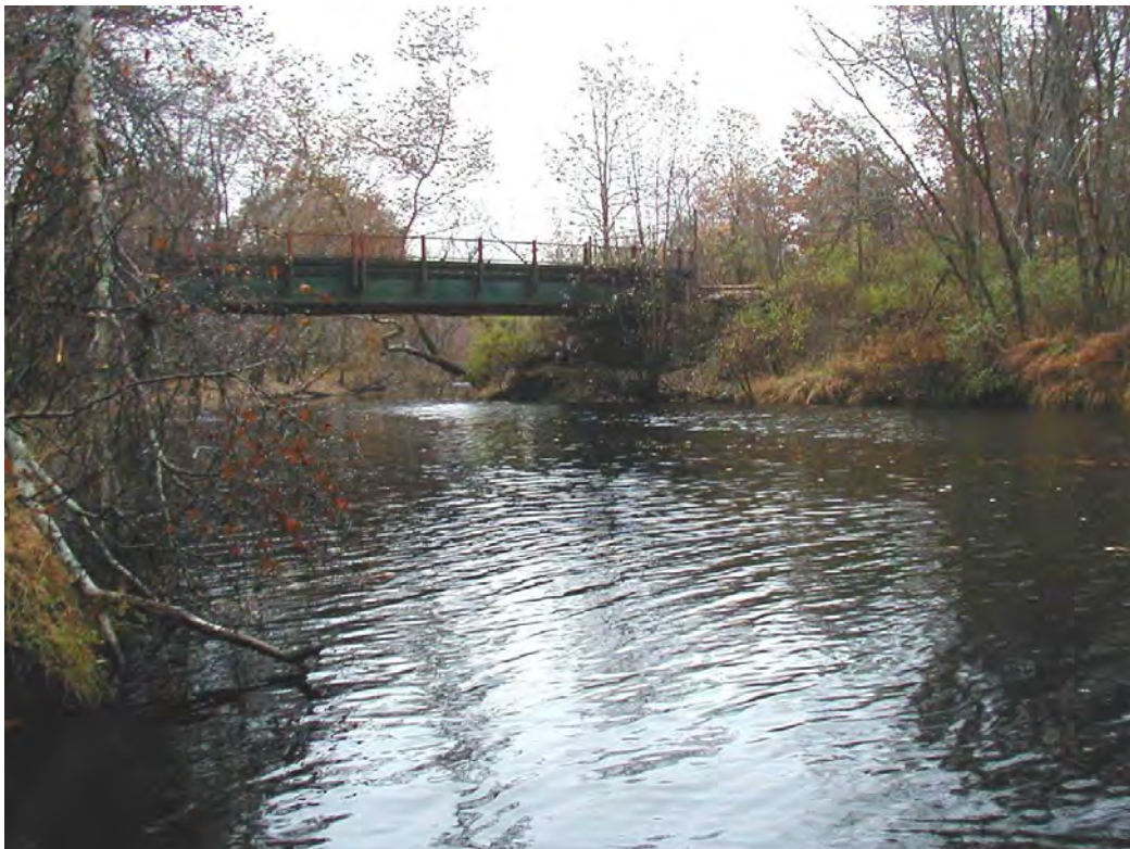
Figure 7 Station NM21 upstream – Tank Bridge (11/6/2002)
