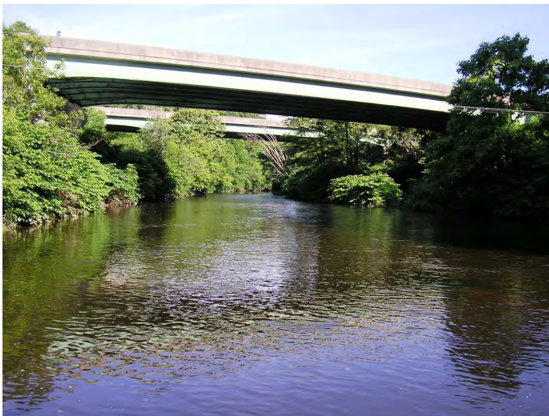
Figure 3 Station NN12 upstream – I-190 Bridges (6/17/2009)
